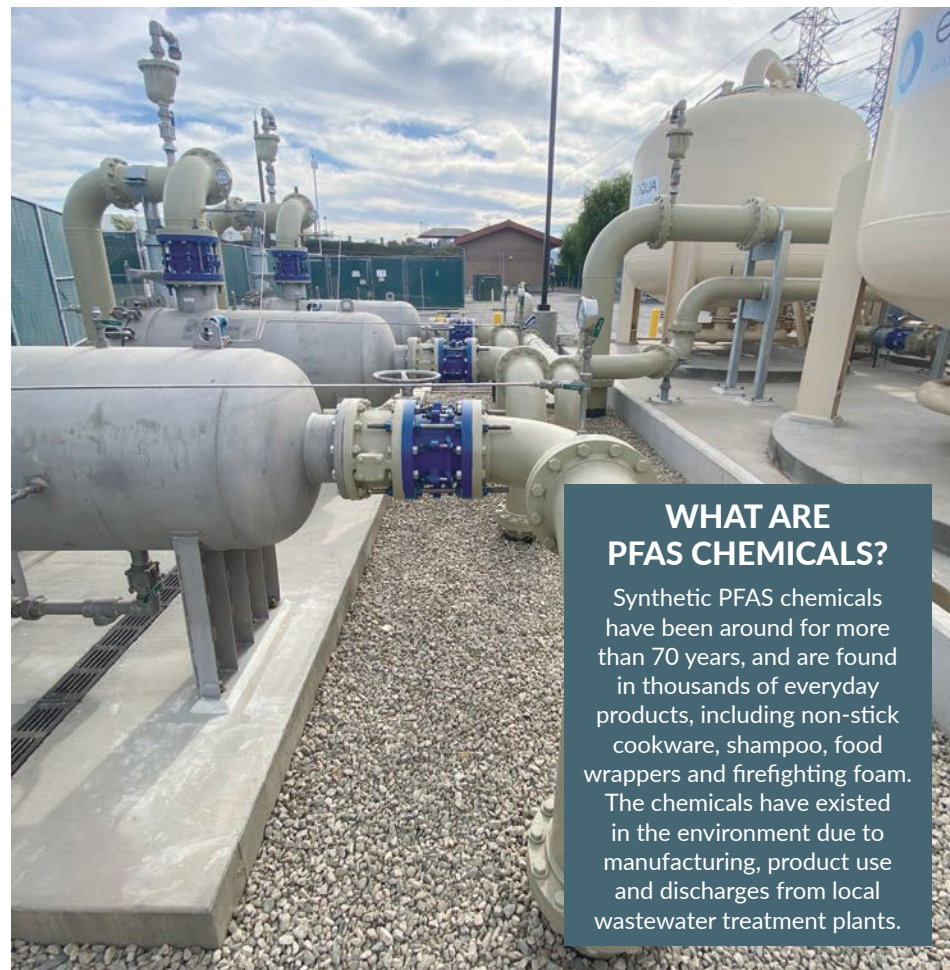
Treatment facility opened in 2021, which removes PFAS from 3 groundwater wells in the area.
