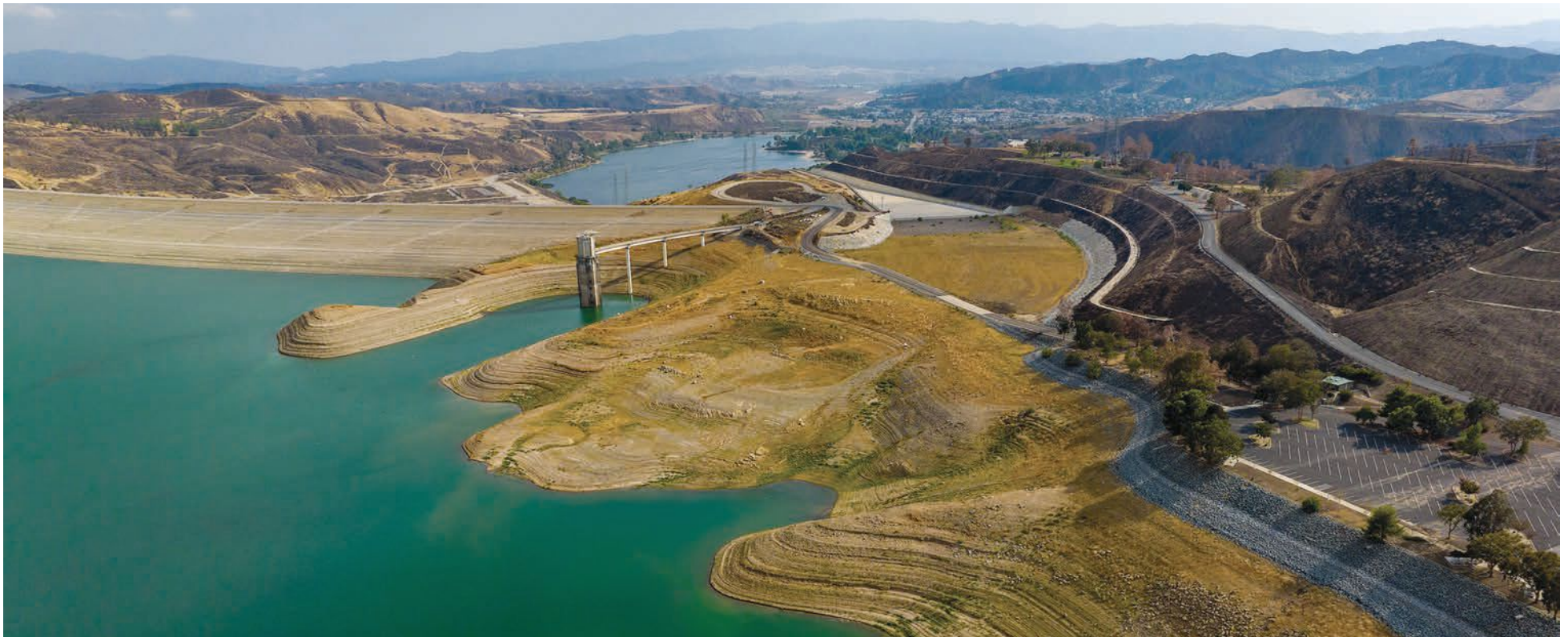
A drone view of Castaic Lake, dam, intake tower, auxiliary spillway, and lagoon. Photo taken Sept. 13. On this date, the storage was 119,442 reservoir acre-feet (AF), which is 37 percent of the total capacity. Photo courtesy of The California Department of Water Resources
