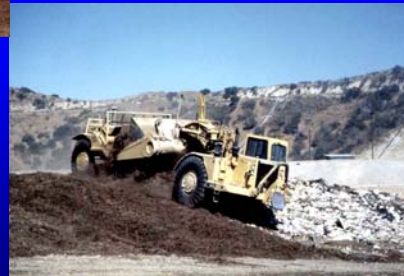
Green waste placed as ADC.
