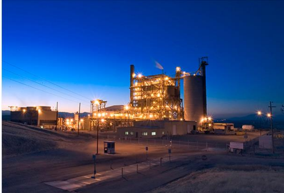
Mt. Poso Cogeneration Plant, Bakersfield (Source: California Biomass Energy Alliance)
