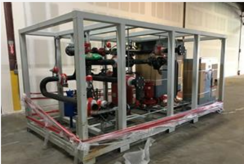
HEATING SYSTEM SKID
