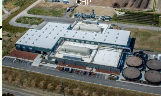
Zero Waste Energy Development Co. San Jose, CA OFMSW + SSO Dry Anaerobic Digestion to CHP
