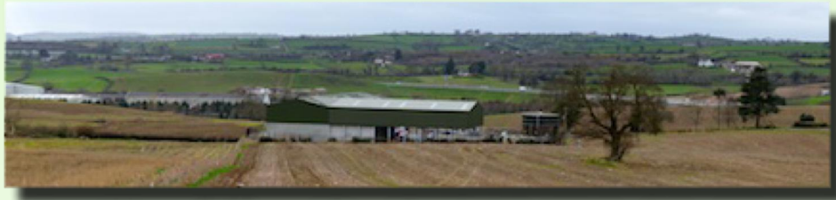
Typical Gasification Plant
