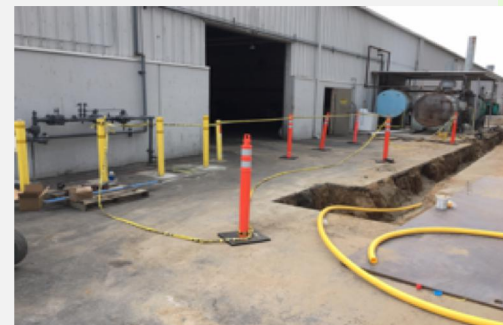
GAS LINE RELOCATION
