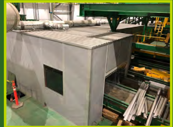
Sort Enclosures / HVAC
