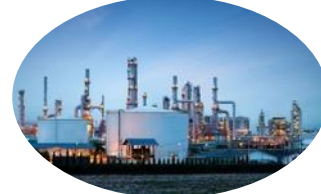
Natural Gas Distribution
