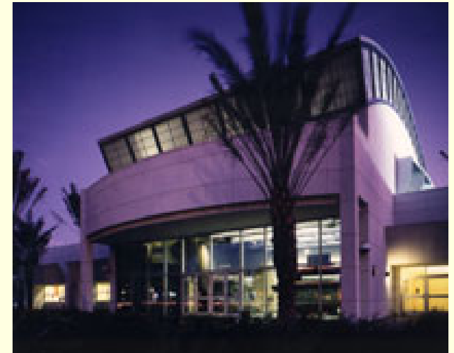
Gas Company's Energy Resource Center, Downey, CA.
