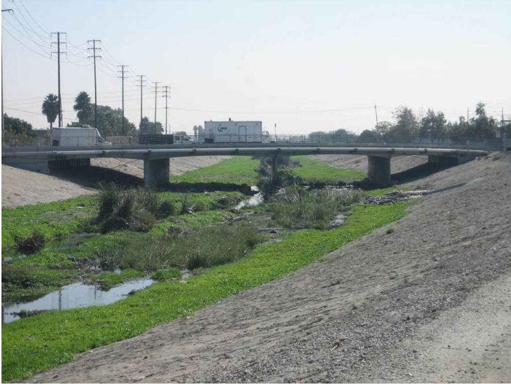
Looking d/s at Santa Fe Ave near Sta. 155+35 (HEC-RAS Model)
