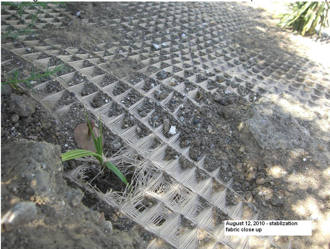
Looking at channel bank stabilization fabric at Sta. 48+25 (HEC-RAS Model)
