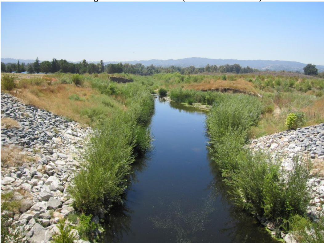
Looking d/s Sta. 2+48.611 (HEC-RAS Model)
