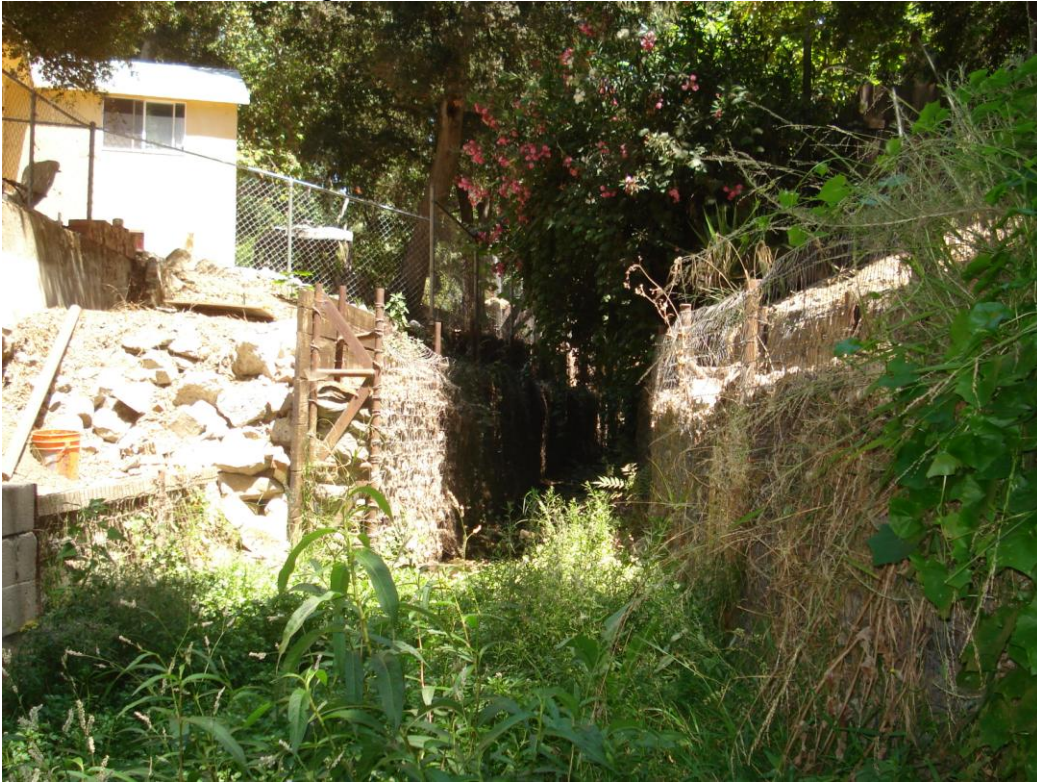
Looking d/s Sta. 40+34 (HEC-RAS Model)
