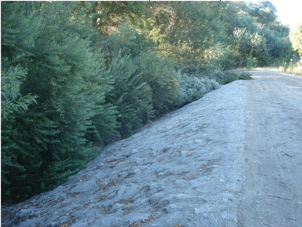
WEST FORK – Looking u/s on access road at Sta. 5+34.32 (HEC-RAS Model)
