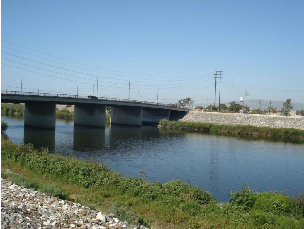
Looking d/s Sta. 117+00 (HEC-RAS Model)
