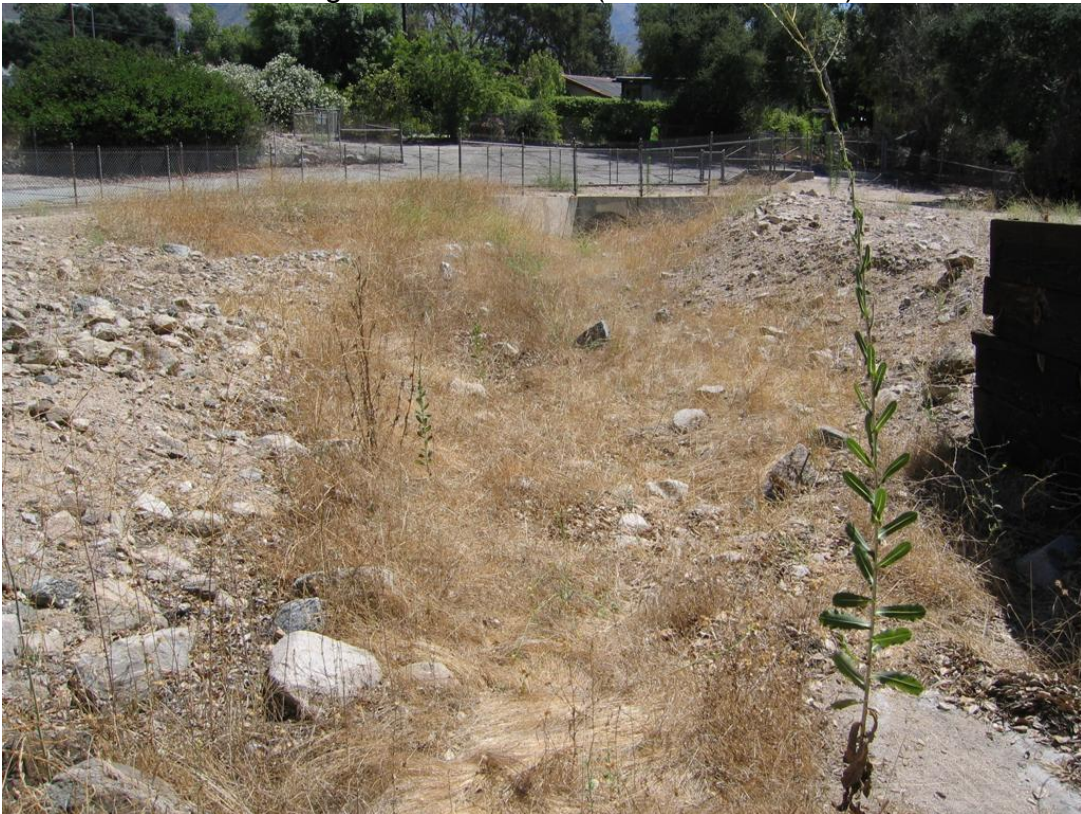
Looking d/s Sta. 1+55.92 (HEC-RAS Model)
