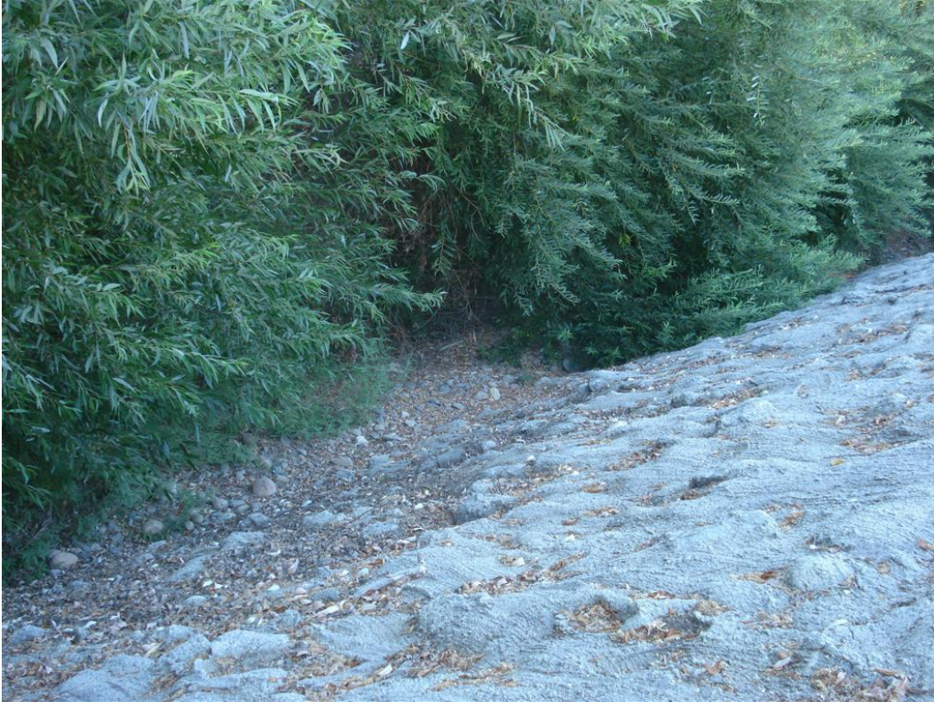
WEST FORK – Looking u/s on access road into channel at Sta. 5+34.32 (HEC-RAS Model)
