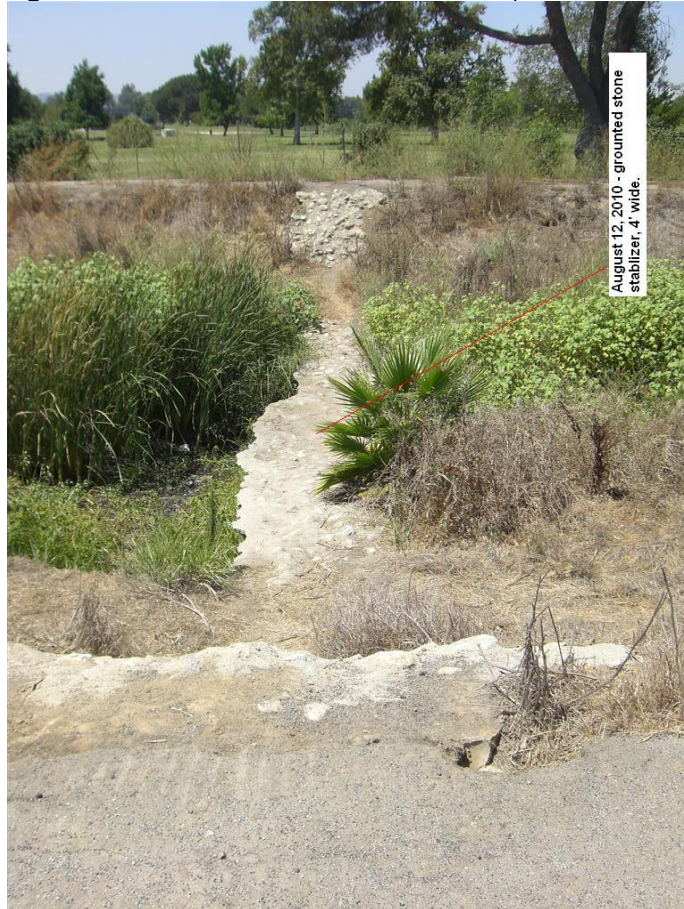
Looking west into channel at Sta. 30+00 (HEC-RAS Model)
