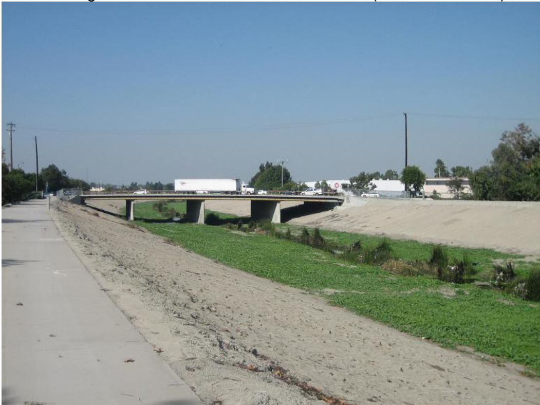
Looking u/s at Del Amo Blvd near Sta. 99+75 (HEC-RAS Model)
