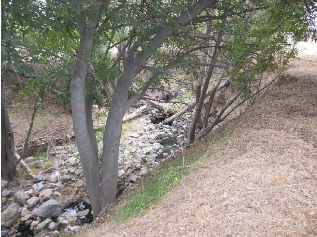
Looking d/s Sta. 1+88.739 (HEC-RAS Model)
