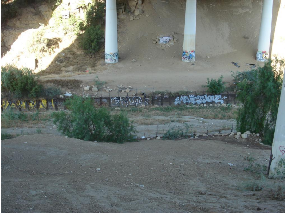
Looking west into the channel from under the 118 Freeway
