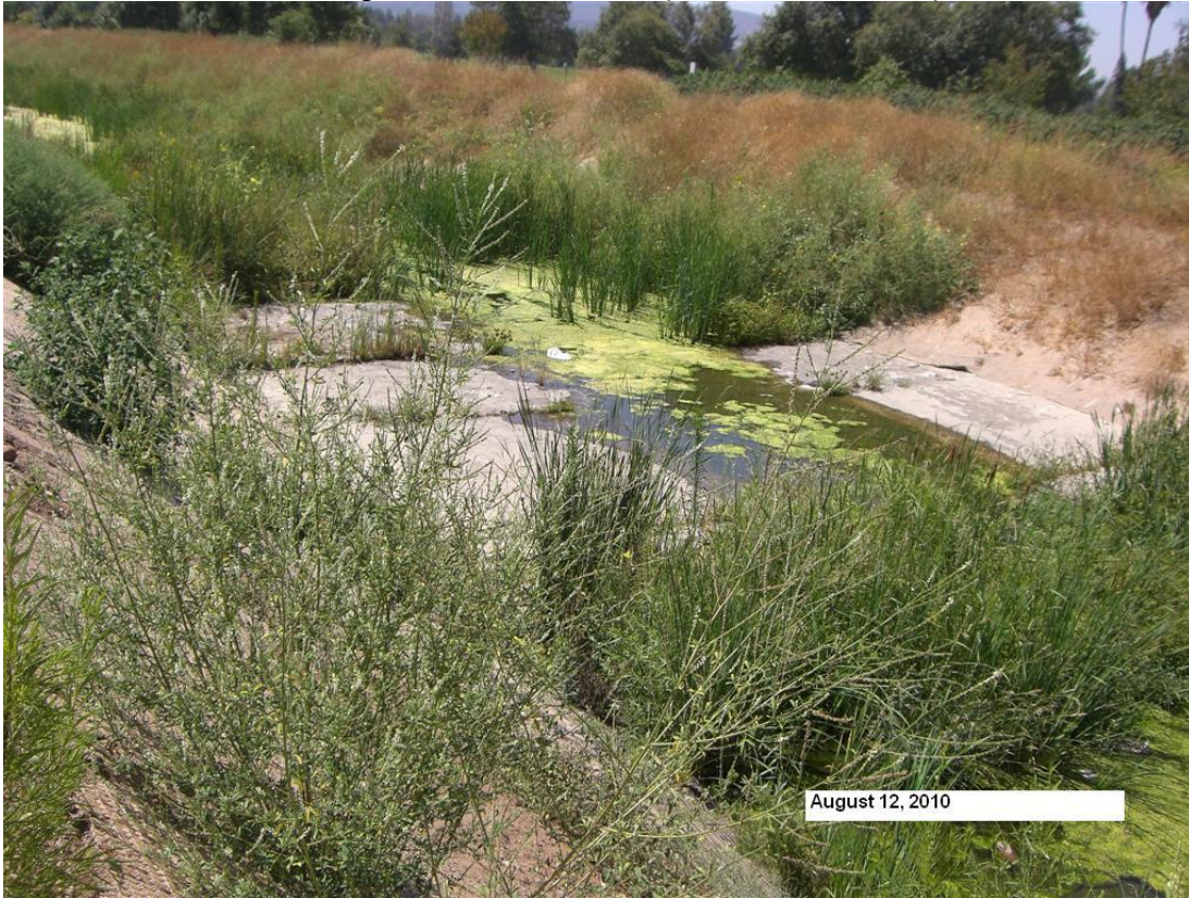
Looking d/s at Sta. 42+70 (HEC-RAS Model)
