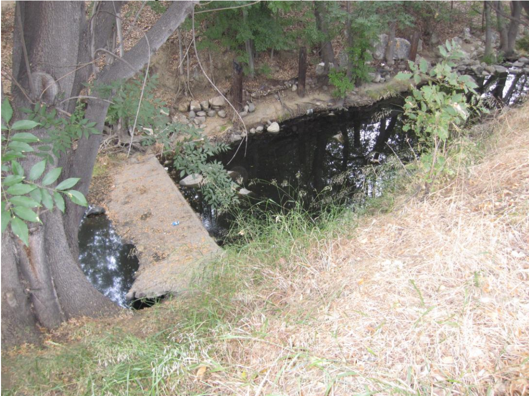
Looking d/s Sta. 2+17.286 (HEC-RAS Model)
