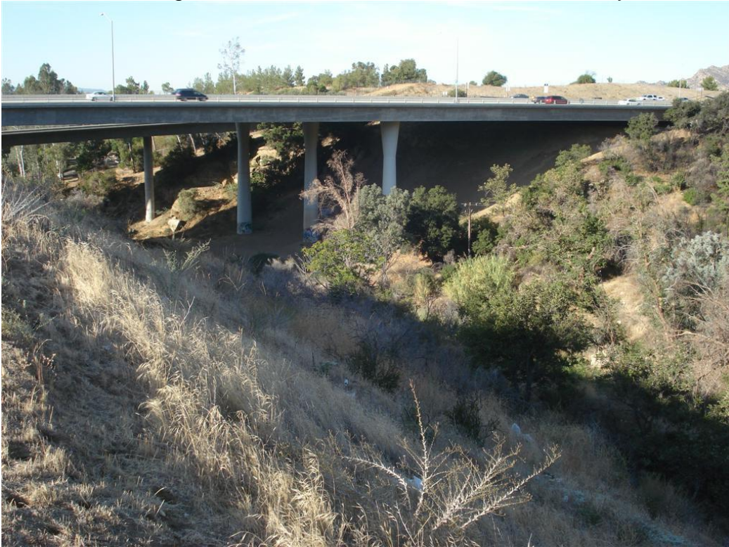
Looking d/s from De Soto Ave onto the 118 Freeway
