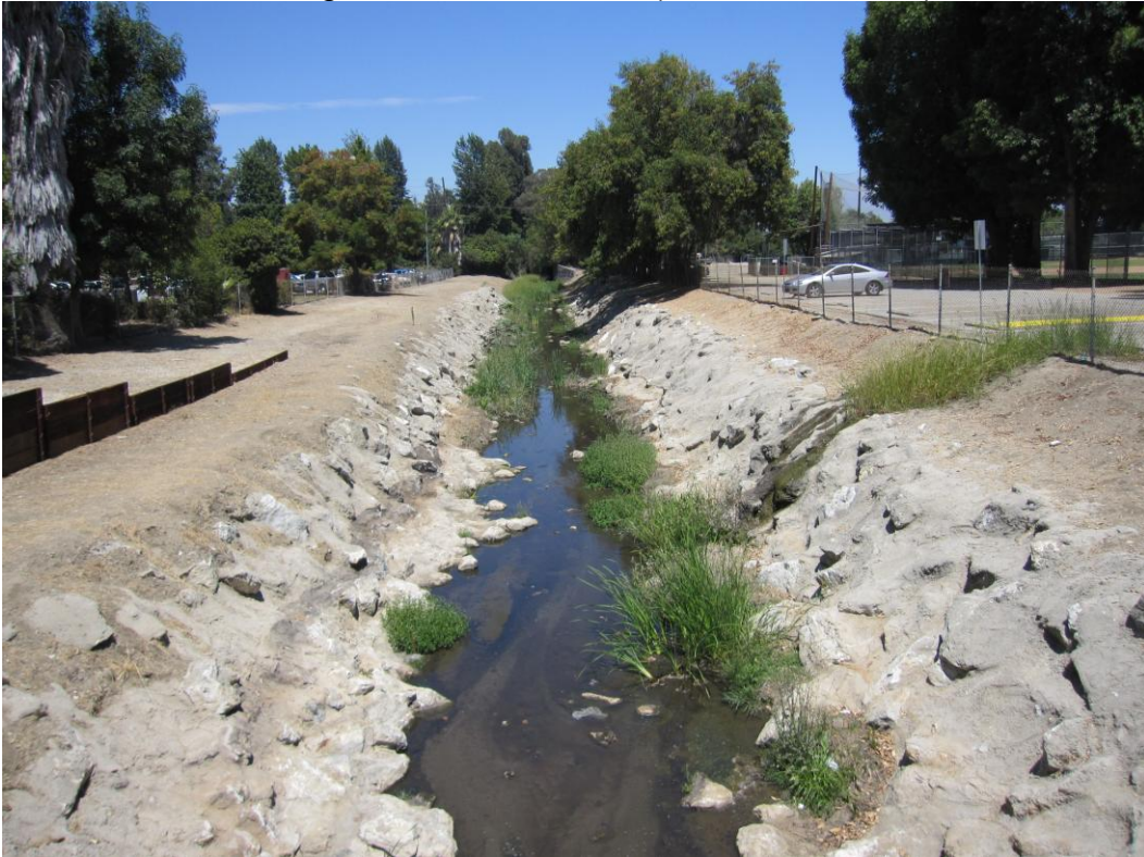
Looking d/s Sta. 11+81.478 (HEC-RAS Model)
