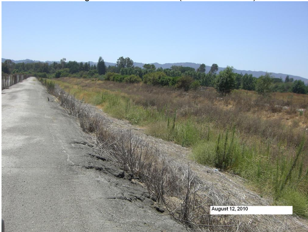
Looking d/s from Sta. 22+00 (HEC-RAS Model)
