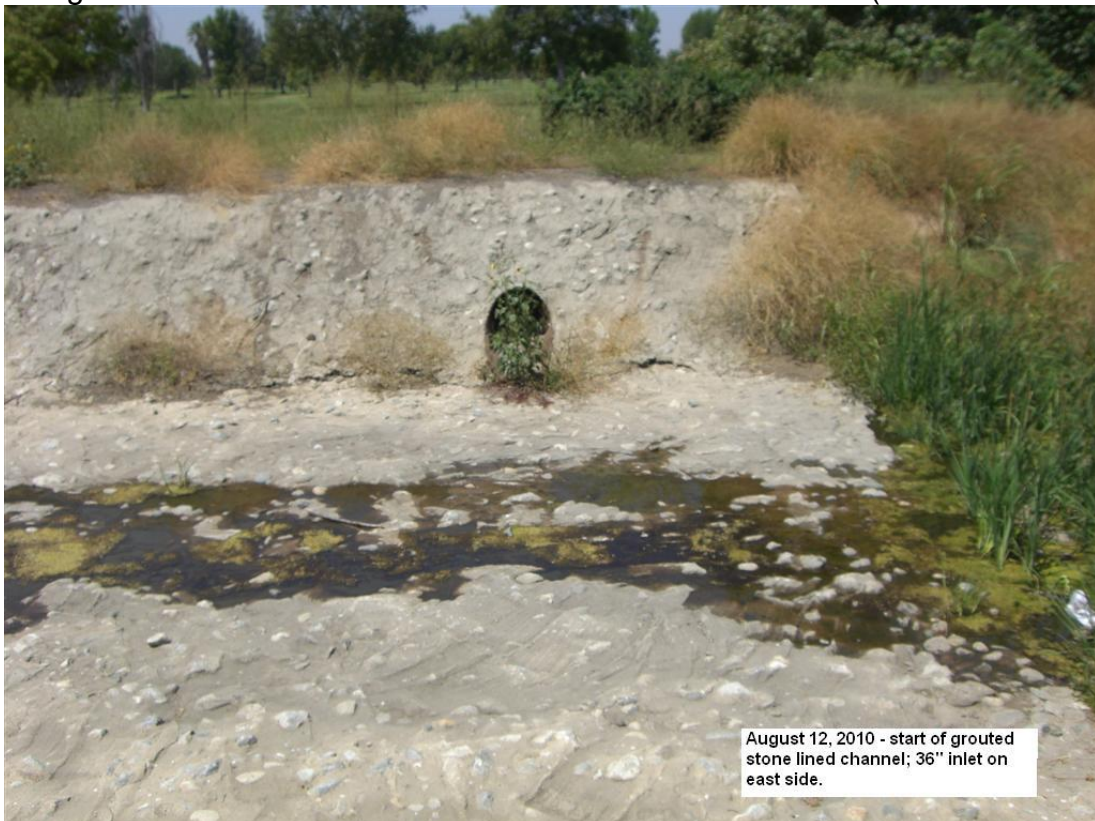
Looking west into channel between Sta. 36+63 and Sta. 36+00 (HEC-RAS Model)
