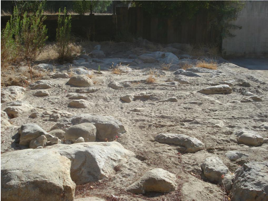
Looking east along approximately Sta. 0+71.09 (HEC-RAS Model)
