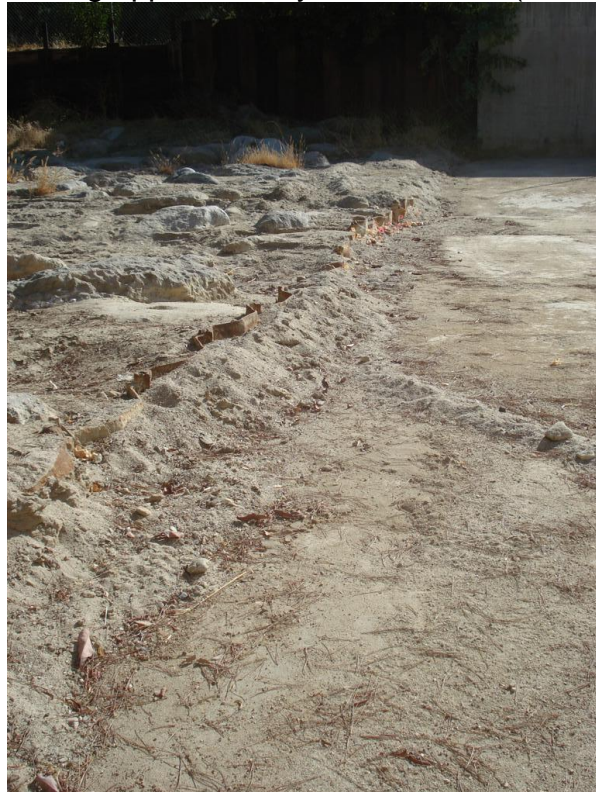
Looking east along approximately Sta. 0+66.00 (HEC-RAS Model)
