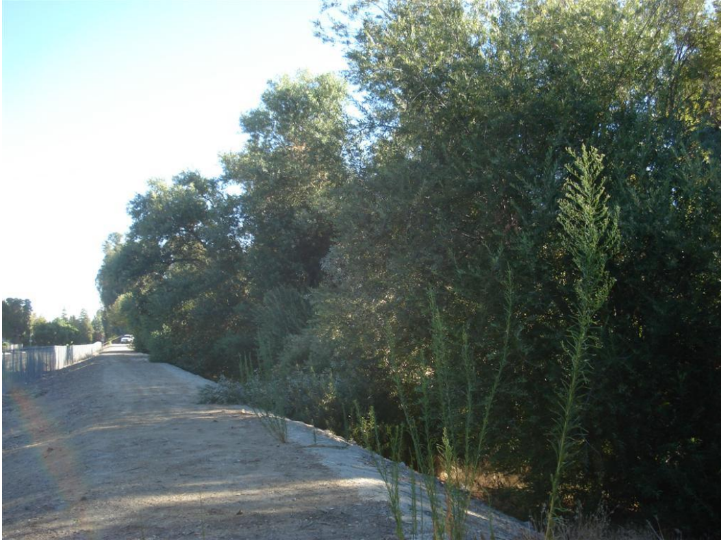
WEST FORK – Looking north u/s on access road into channel at Sta. 6+24.57 (HEC-RAS Model)
