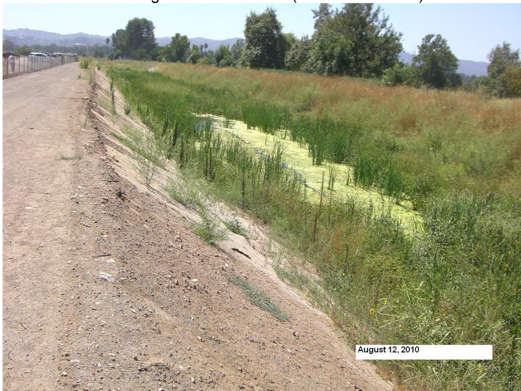
Looking d/s at Sta. 41+30 (HEC-RAS Model)
