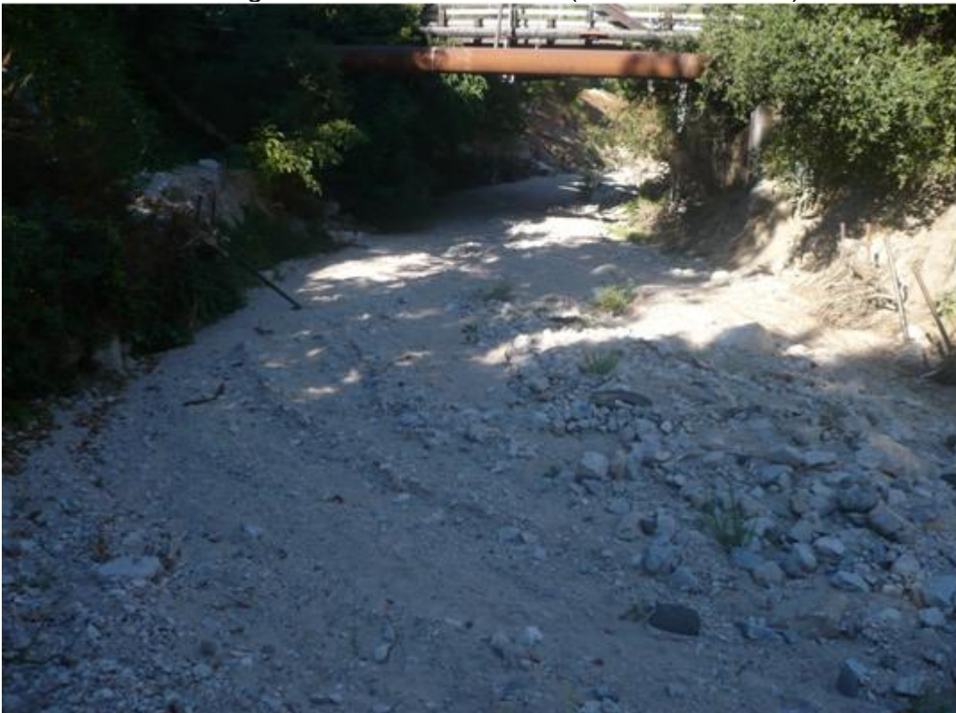
Looking d/s from Sta. 11+34.21 (HEC-RAS Model)
