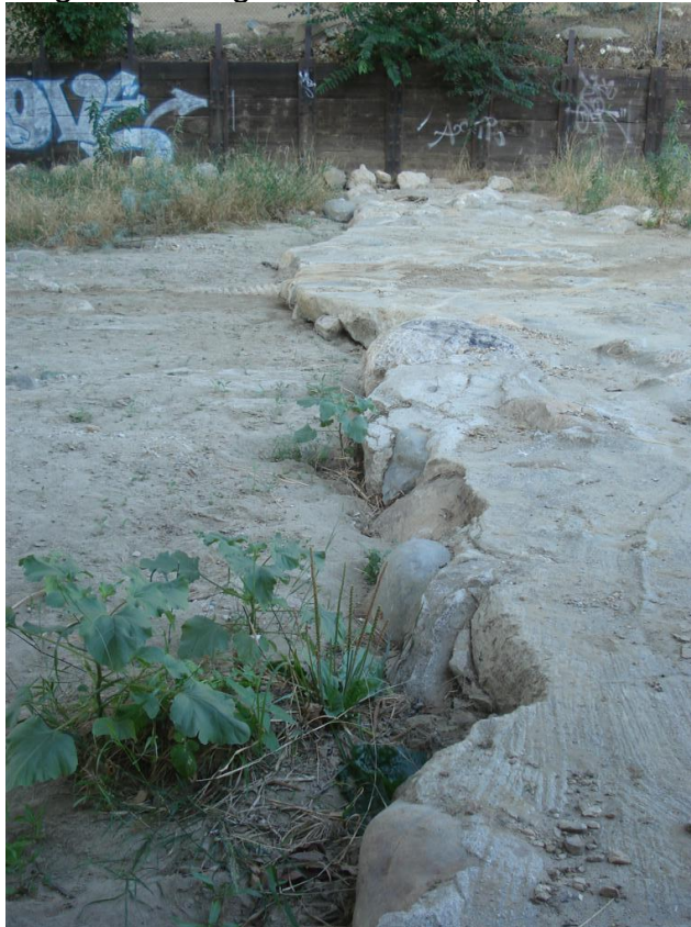
Looking west along Sta. 9+53.44 (HEC-RAS Model)
