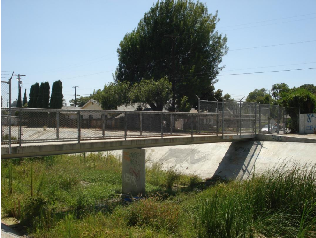
Looking d/s Sta. 140+16 (HEC-RAS Model)
