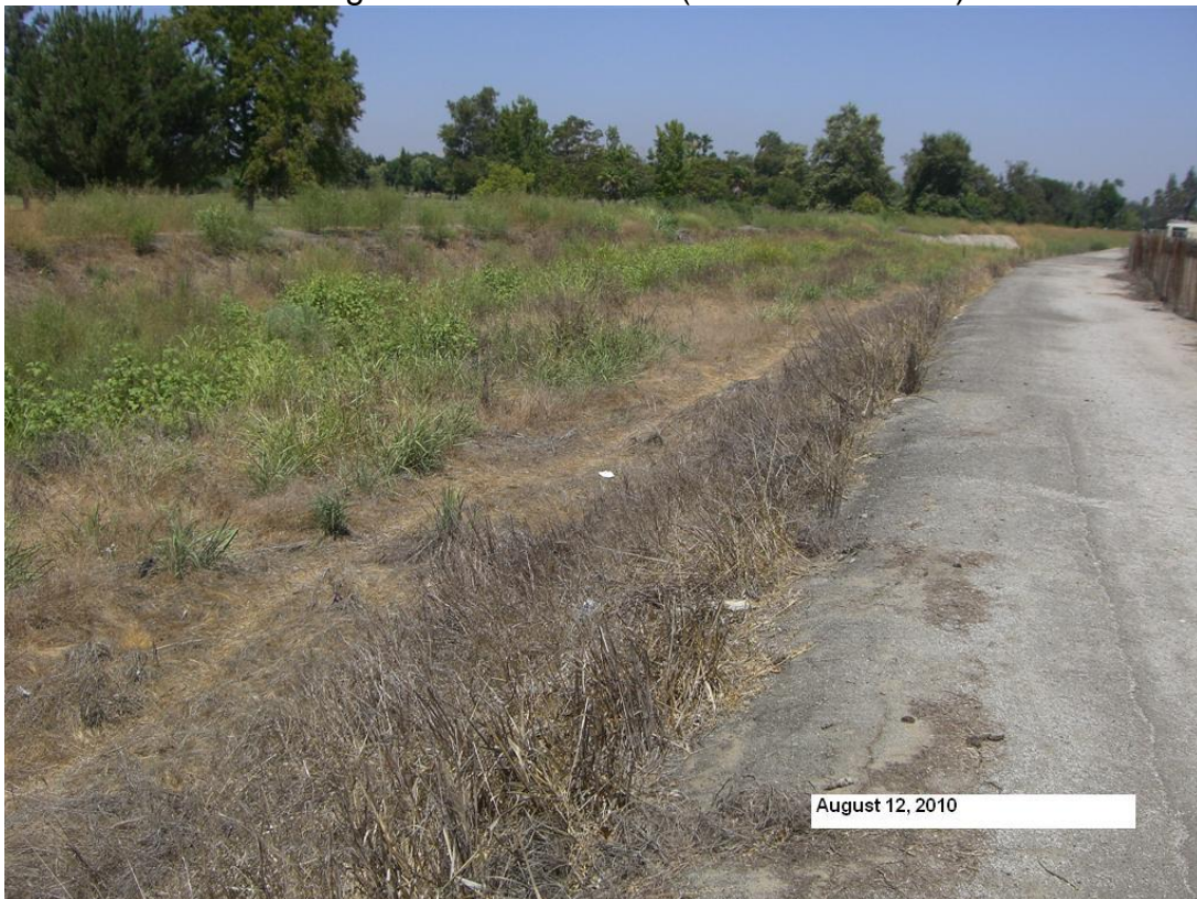
Looking u/s into Sta. 31+00 (HEC-RAS Model)
