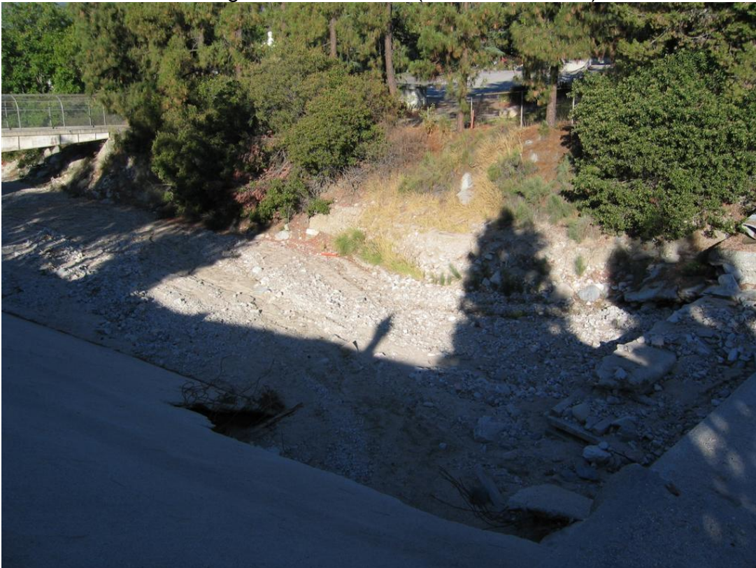
Looking d/s Sta. 8+47.73 (HEC-RAS Model)
