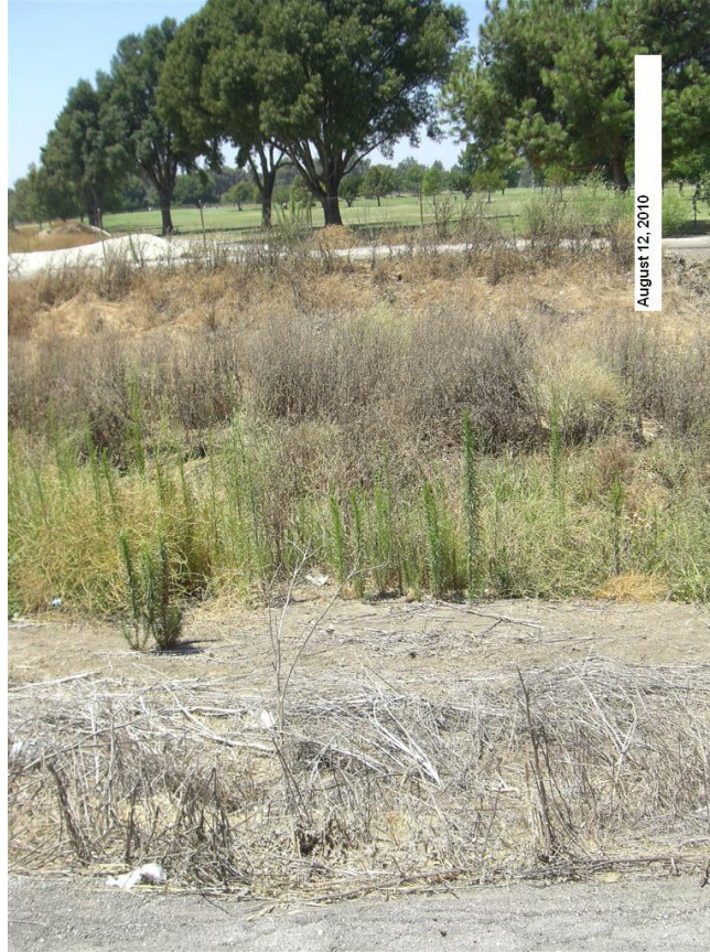
Looking west into channel at Sta. 22+00 (HEC-RAS Model)
