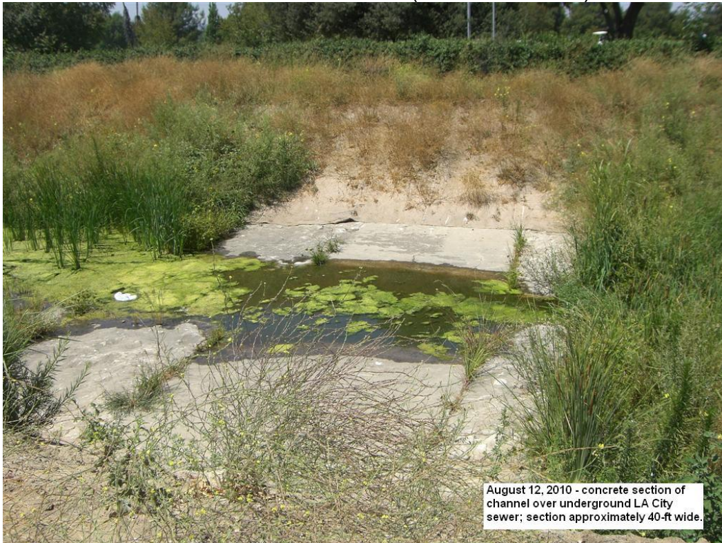
Looking west into concrete stretch of channel between Sta. 42+70 and Sta. 42+30 (HEC-RAS Model)
