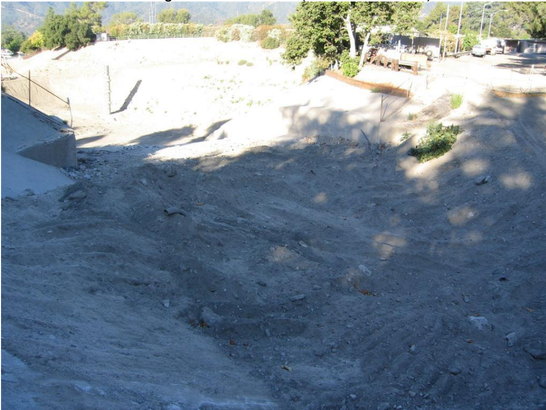
Looking d/s Sta. 0+88.91 (HEC-RAS Model)
