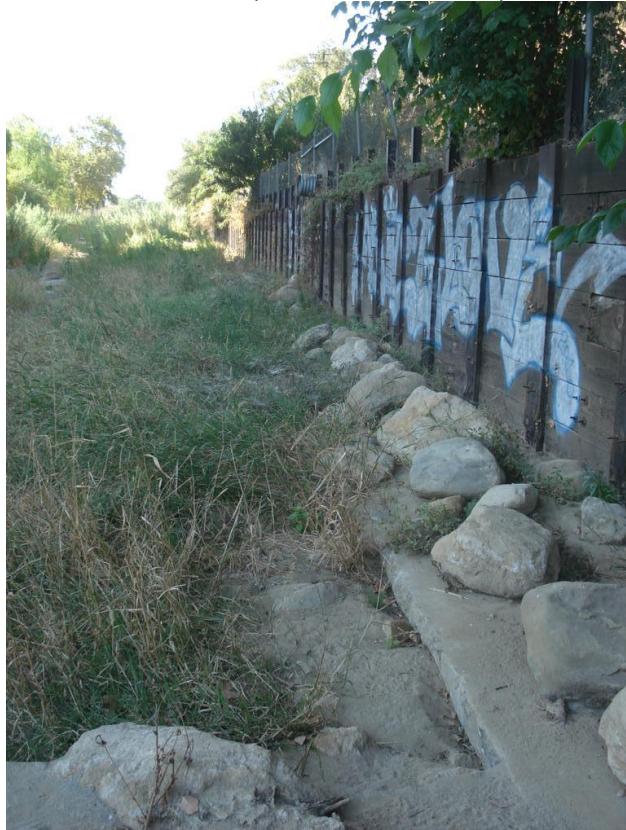
Looking d/s from Sta. 10+23.25 (HEC-RAS Model) at west side of channel
