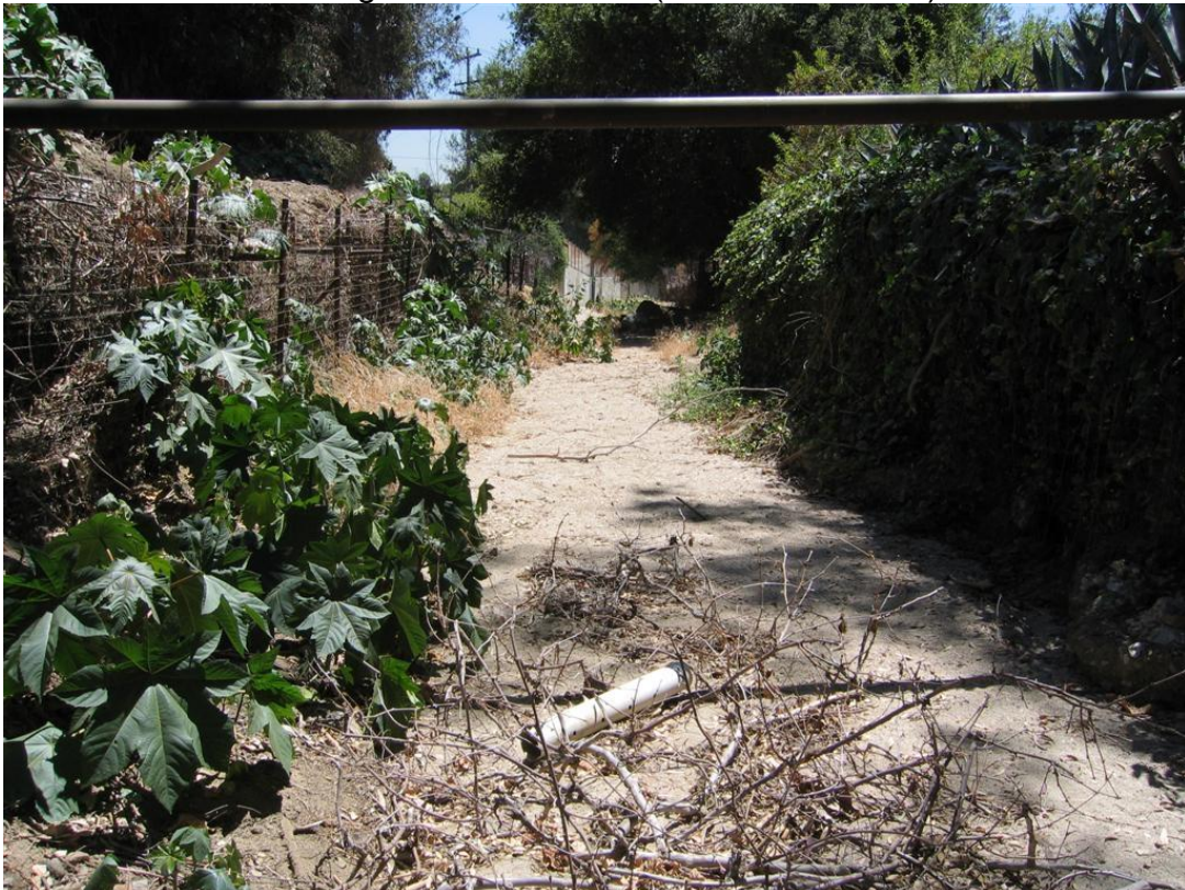
Looking d/s Sta. 4+60.71 (HEC-RAS Model)
