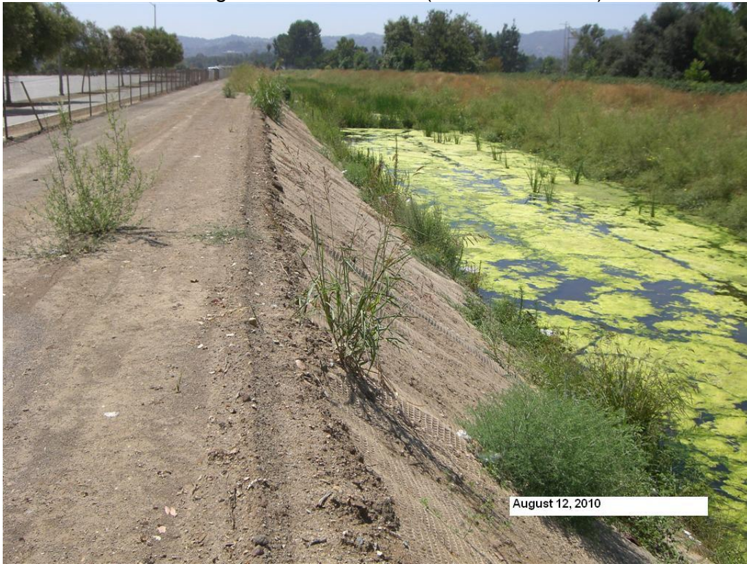
Looking west at stabilization fabric at channel bottom at Sta. 43+00 (HEC-RAS Model)
