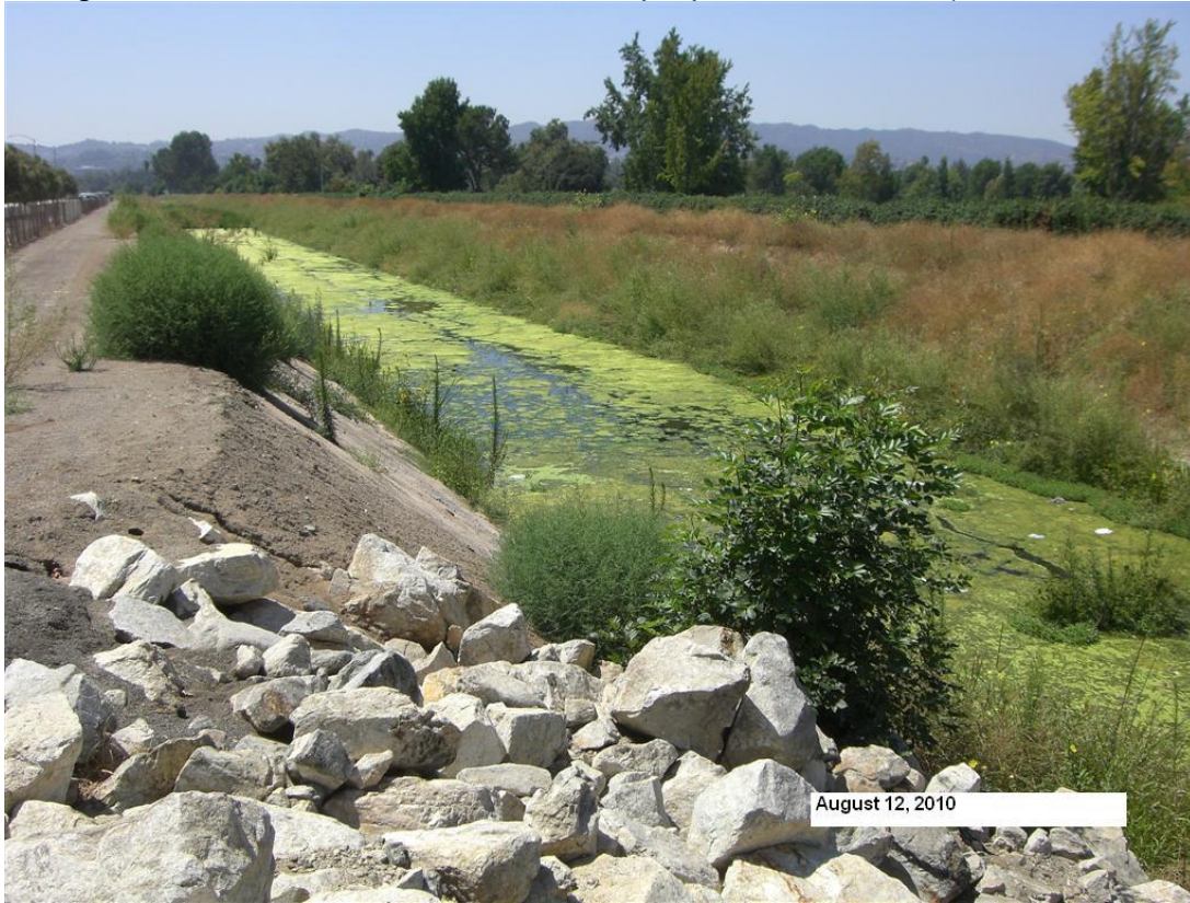
Looking d/s of Sta. 48+75, transition from riprap to soft-bottom (HEC-RAS Model)
