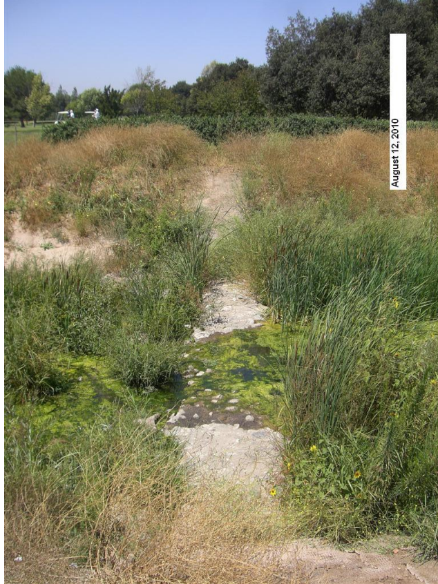
Looking at stone stabilizer located between Sta. 42+30 and Sta. 41+30 (HEC-RAS Model)
