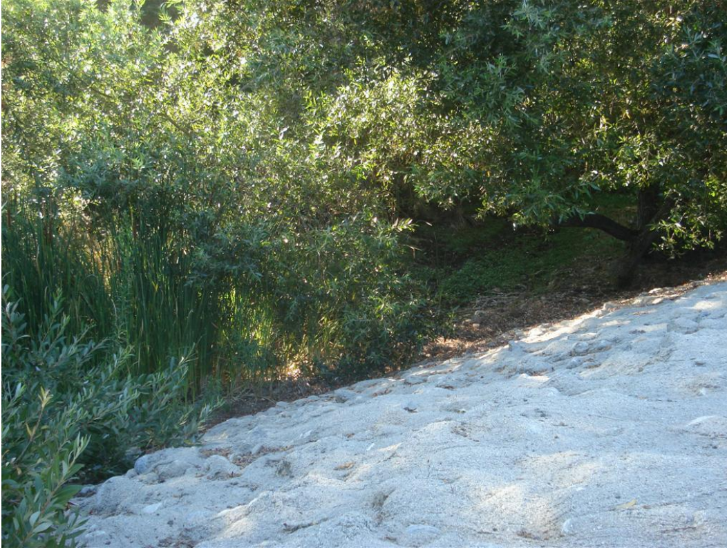
WEST FORK – Looking d/s on access road into channel at Sta. 4+12.95 (HEC-RAS Model)
