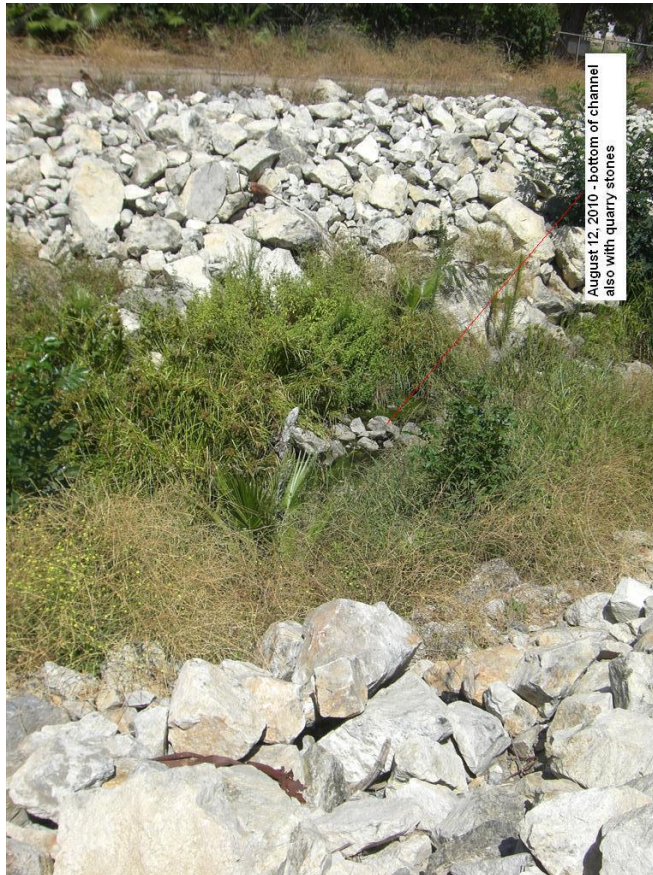
Looking west into channel between Sta. 51+45 and Sta. 50+60 (HEC-RAS Model)
