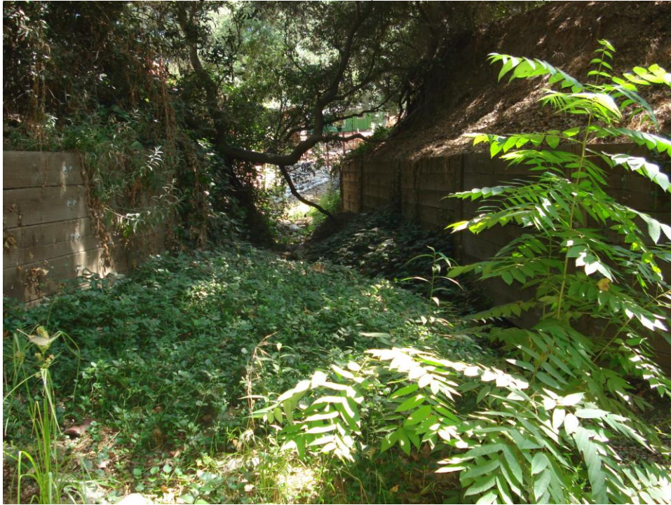
Looking d/s Sta. 47+85 (HEC-RAS Model)
