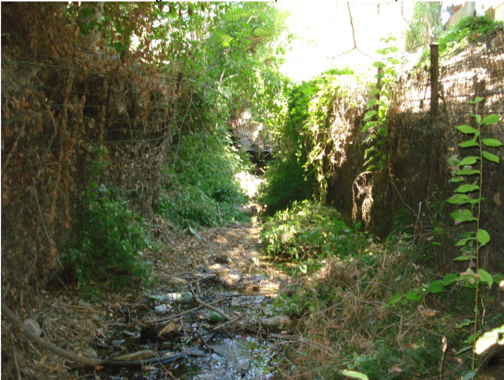
Looking d/s Sta. 50+58 (HEC-RAS Model)
