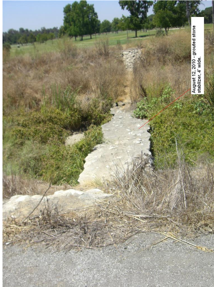
Looking west into channel at stone stabilizer at Sta. 24+00 (HEC-RAS Model)
