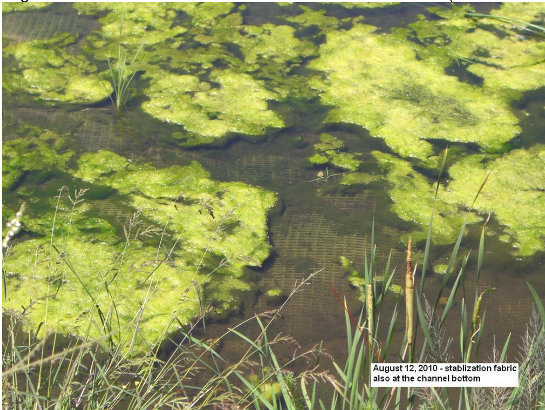
Looking west at stabilization fabric at channel bottom at Sta. 43+00 (HEC-RAS Model)
