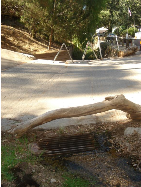
Looking d/s Sta. 21+50 (HEC-RAS Model)
