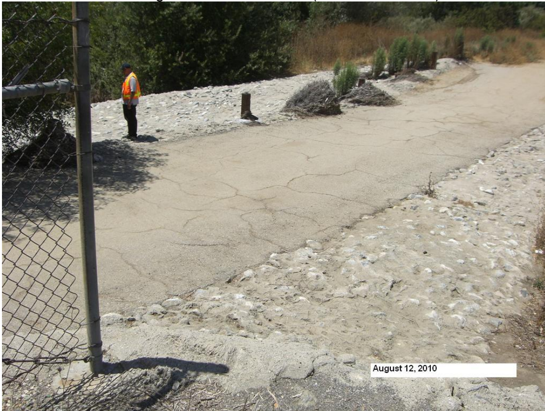
Looking d/s from Sta. 11+91 (HEC-RAS Model)
