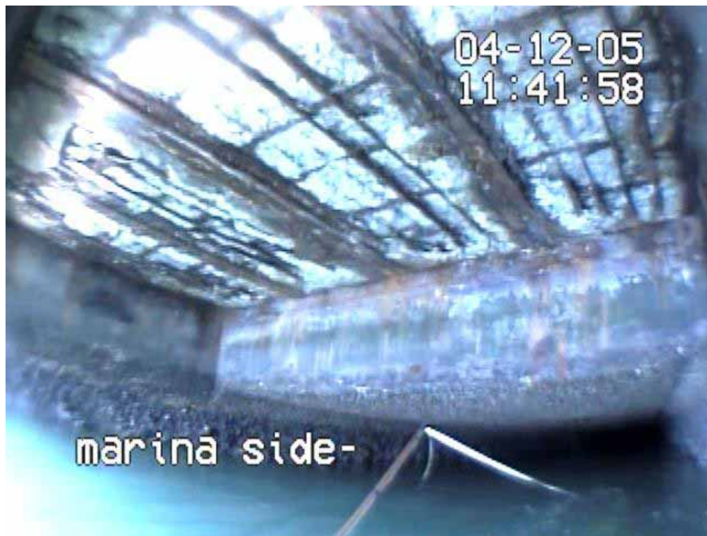
PHOTO 3 - EXPOSED REBAR AND MISSING CONCRETE AT MARINA SIDE COVERS, LOOKING FORWARDS THE LAGOON
