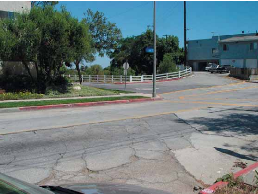
Figure 3.2-7 View along the PE Right-of-Way facing southeast at Termino Avenue and 8th Street
