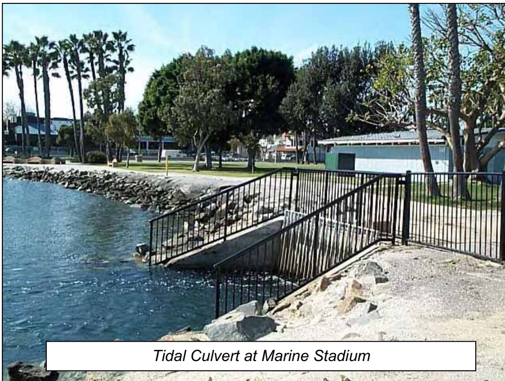
Figure 2.4 Tidal Culvert Site Photos
