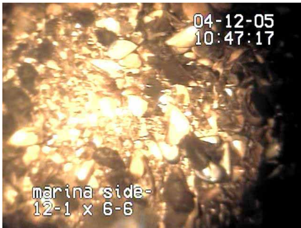
PHOTO 2 - TYPICAL MATERIAL ON BUILD UP OF CLAMS AND MUSSELS ON THE FLOOR OF THE CULVERT
