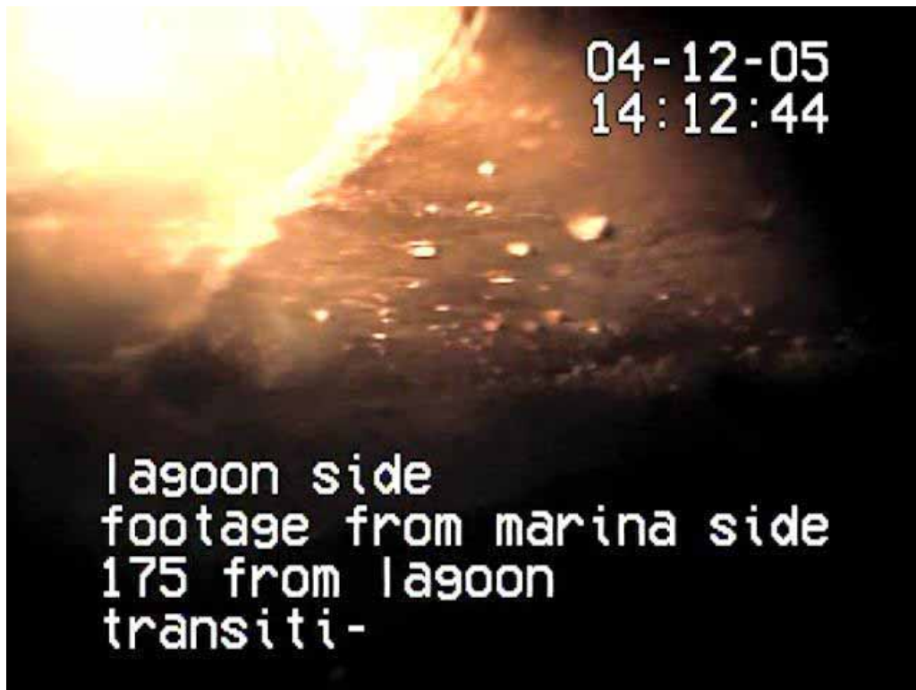
PHOTO 8 - SHOWING START OF TRANSITION. THE EDGED CONCRETE IN ON THE LEFT CENTER IS THE START OF THE TRANSITION WHERE THE TOP OF THE CULVERT LOWERS
