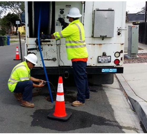
Cleaning a sewer line using hydro jetting.
