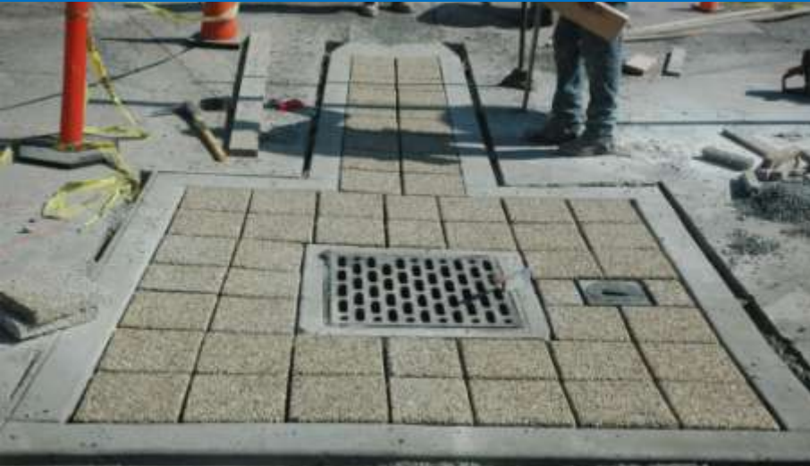
Tiles before Grouting
