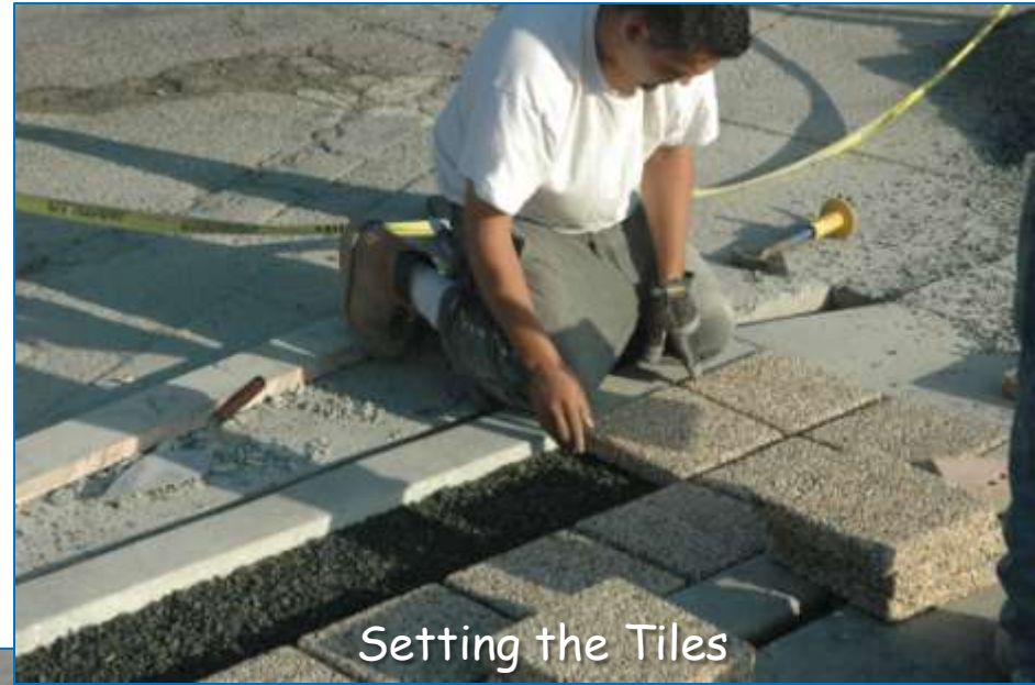
3/8" Fines-free Crushed Stone Bedding Layer
