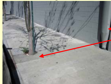
Downspout Planter Boxes/ Bioretention Strip
