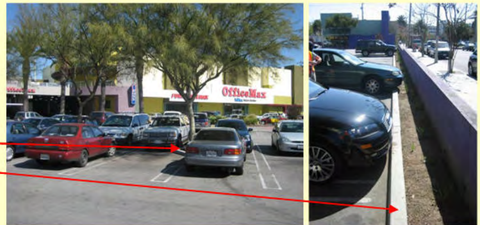
Parking Lot Planter Boxes/ Bioretention Strip w/ Curb Cuts
