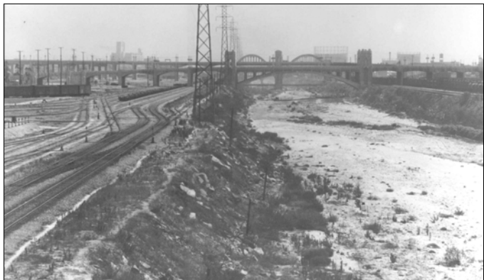
Natural Bottom Los Angeles River @ 4th Street, 1936
