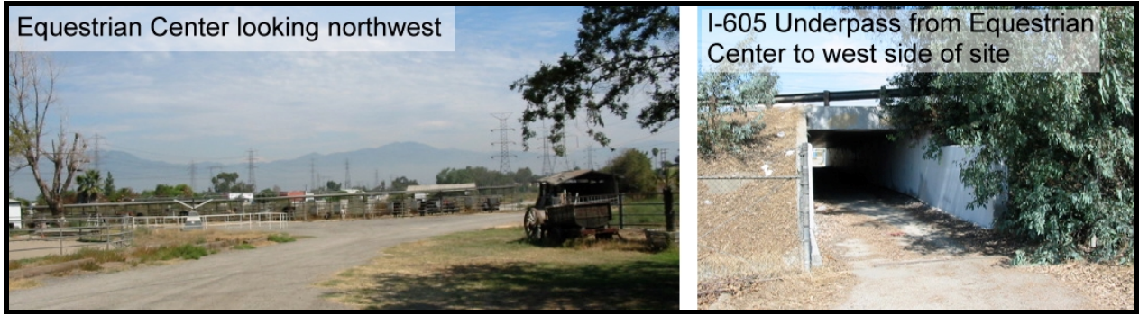
Figure 3-5 Equestrian Facility Existing Conditions
