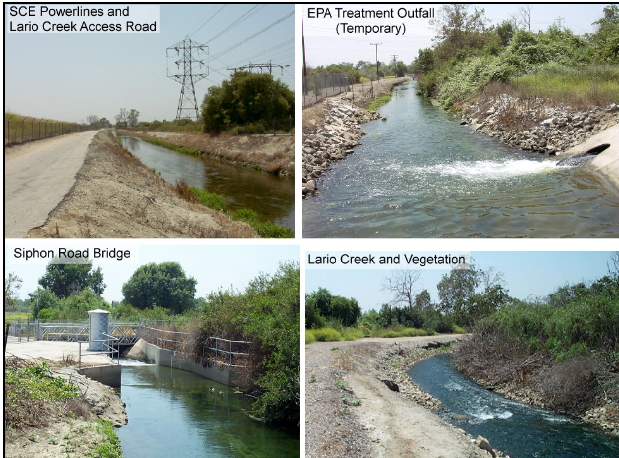
Figure 3-10 Lario Creek Existing Conditions
