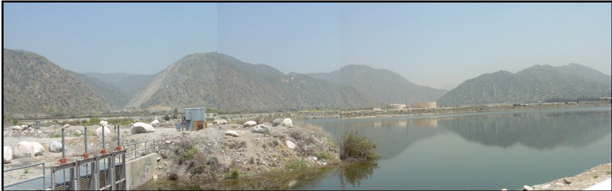
Figure 3-3 Existing Conditions of the San Gabriel Canyon Spreading Grounds
