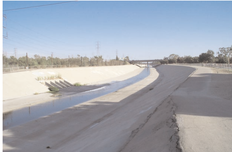
Figure 3-34. The river flows in a concrete channel for 10 miles in Reach 6.
