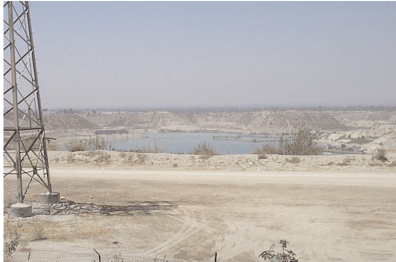
Figure 3-26. The Hanson Quarry is one of the largest mining operations along the river.
