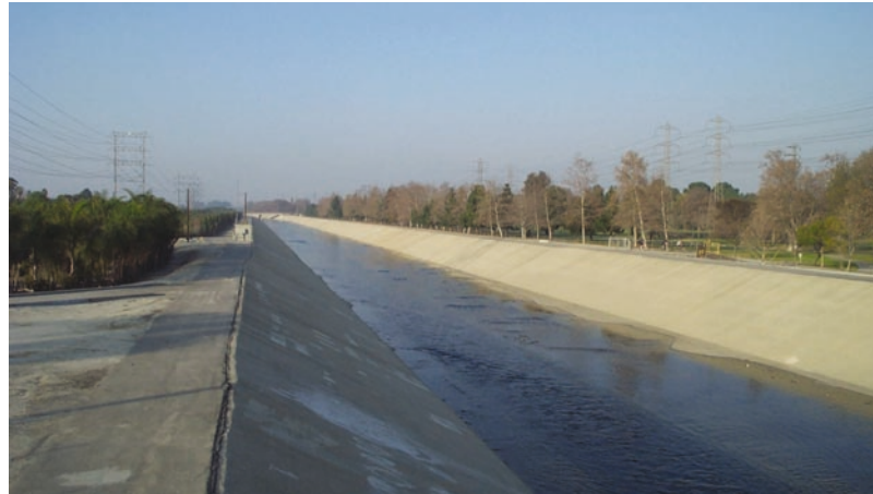
Figure 4-40. Even though the river is in a concrete channel, there is enough open space available at El Dorado Regional Park to consider partial floodplain restoration at this point.
