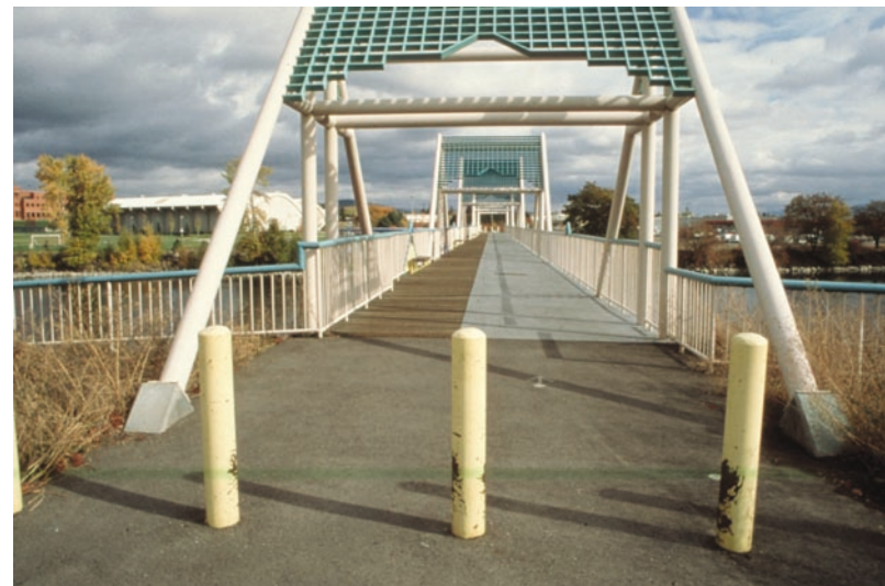
Figure 4-19. Creative bike-pedestrian bridges, like this one in Spokane, Washington, can enliven trails.
