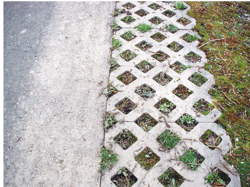
Figure 4-43. Permeable paving at the edges of parking lots and driveways can increase permeable surfaces that allow infiltration.
