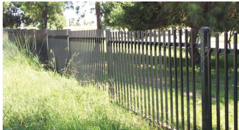
Figure 4-9. Fences can be simple, yet attractive, such as this fence surrounding the Rio Hondo Coastal Spreading Grounds.
