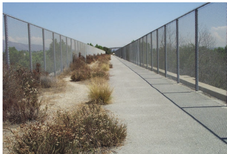
Figure 4-15. Native vegetation grows on top of the Puente-Largo Historic Rail Bridge, alongside the bike trail.
