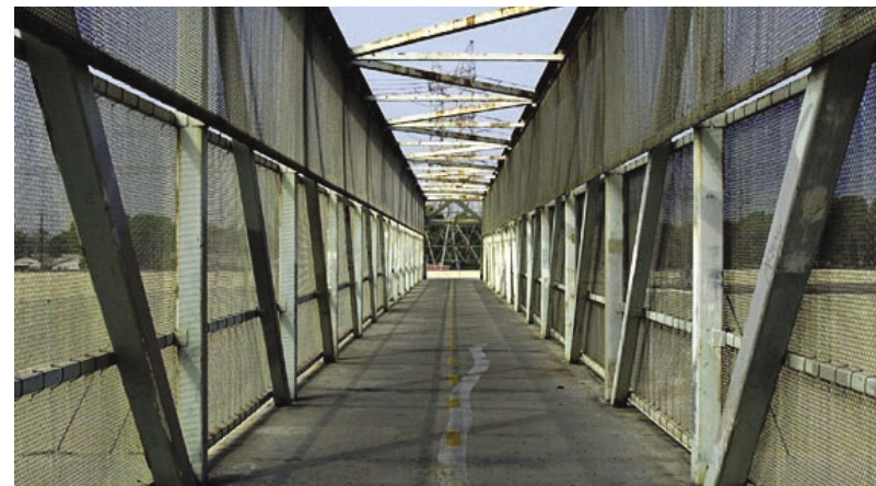
Figure 4-21. The existing bridge at Coyote Creek could be expanded to cross the San Gabriel River near this point.
