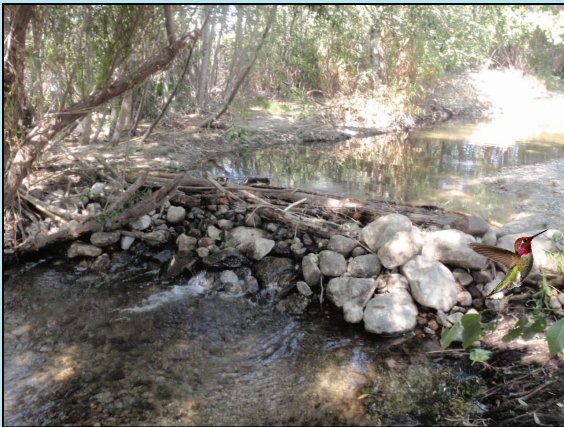
Rock Dam Before Removal
