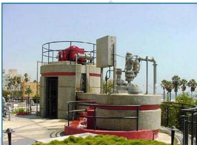
Figure 20: Santa Monica Urban Runoff Recycling Facility
