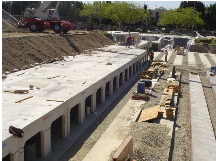
Figure 18: Construction of the Sun Valley Park Infiltration Gallery
