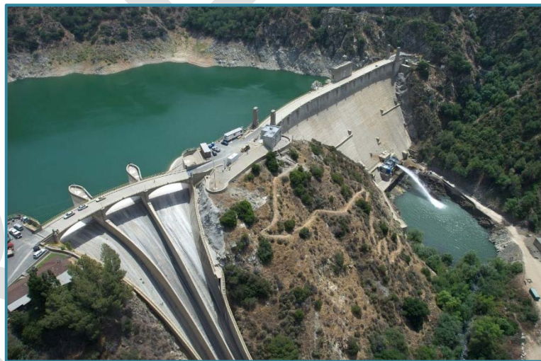
Figure 21: Morris Dam, LACFCD Facility in the San Gabriel Mountains
