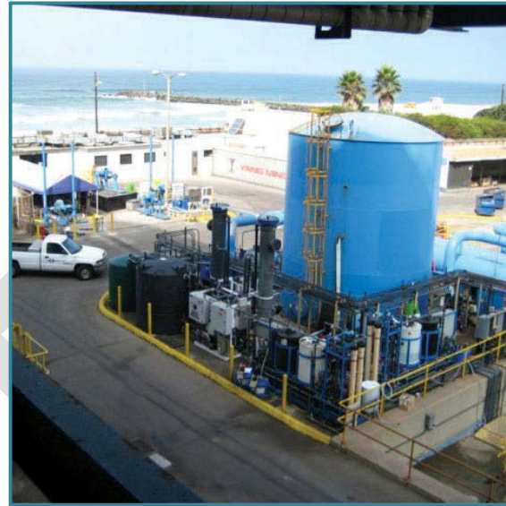
Figure 16: West Basin MWD Desalination Pilot Facility
