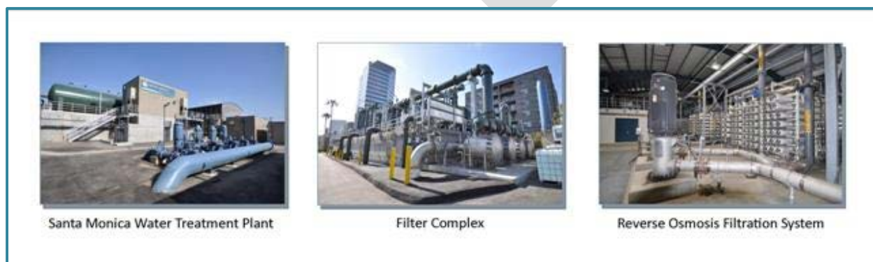
Figure 10: Santa Monica Water Treatment Plant
