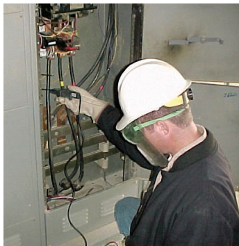
Electrical system being tested at a pump station.
