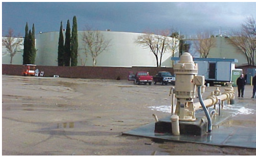
Wellhead with the storage tanks in the background
