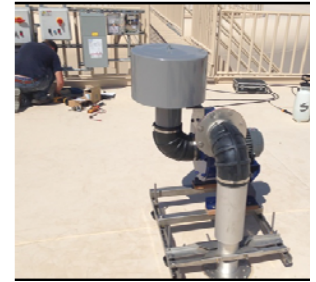
Figure 5: Electrical Unit and Blower
