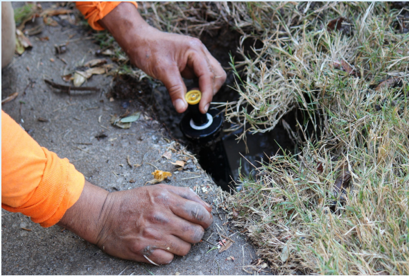
Repairing sprinkler head
