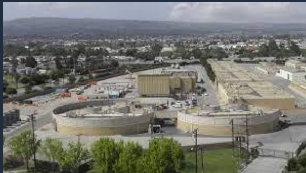
LA County Sanitation Districts, Carson, California
