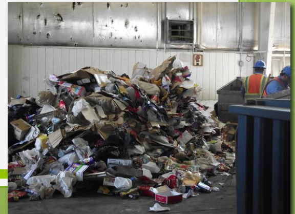
Waste Feed Conveyor To sorting Stations
