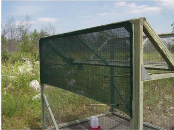
Shade cloth on the west-facing panel.
