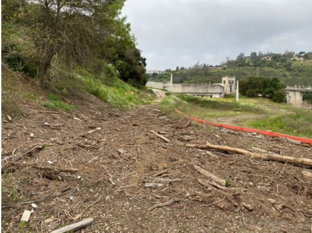
Another view of debris in DG-3A.jpg -118.17334 34.18672
