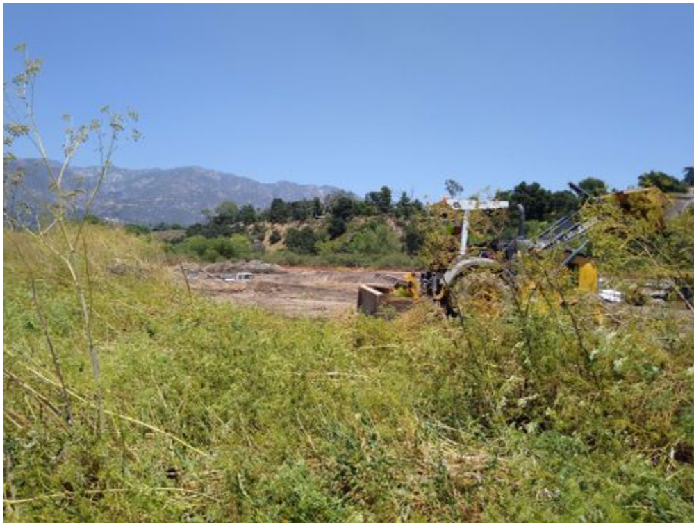
photo_4-clearing emergent vegetation.jpg -118.17388 34.18981
