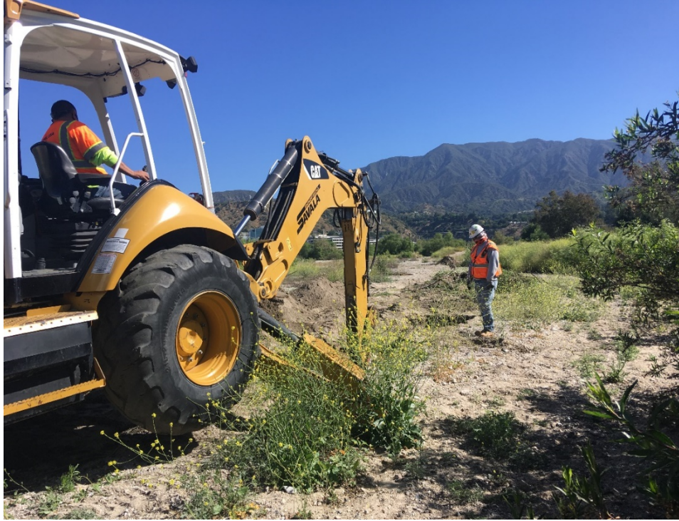
Photo_1-potholing facing NE.jpg -118.17344 34.19028
