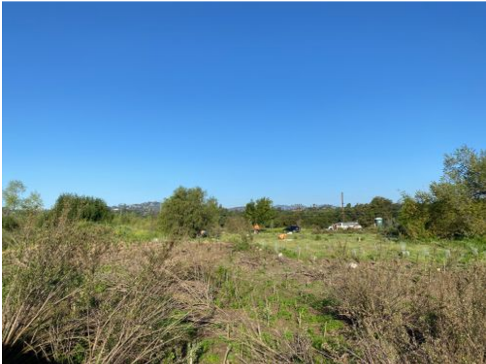
photo_2- Crew removing weeds.jpg -118.17209 34.19374
