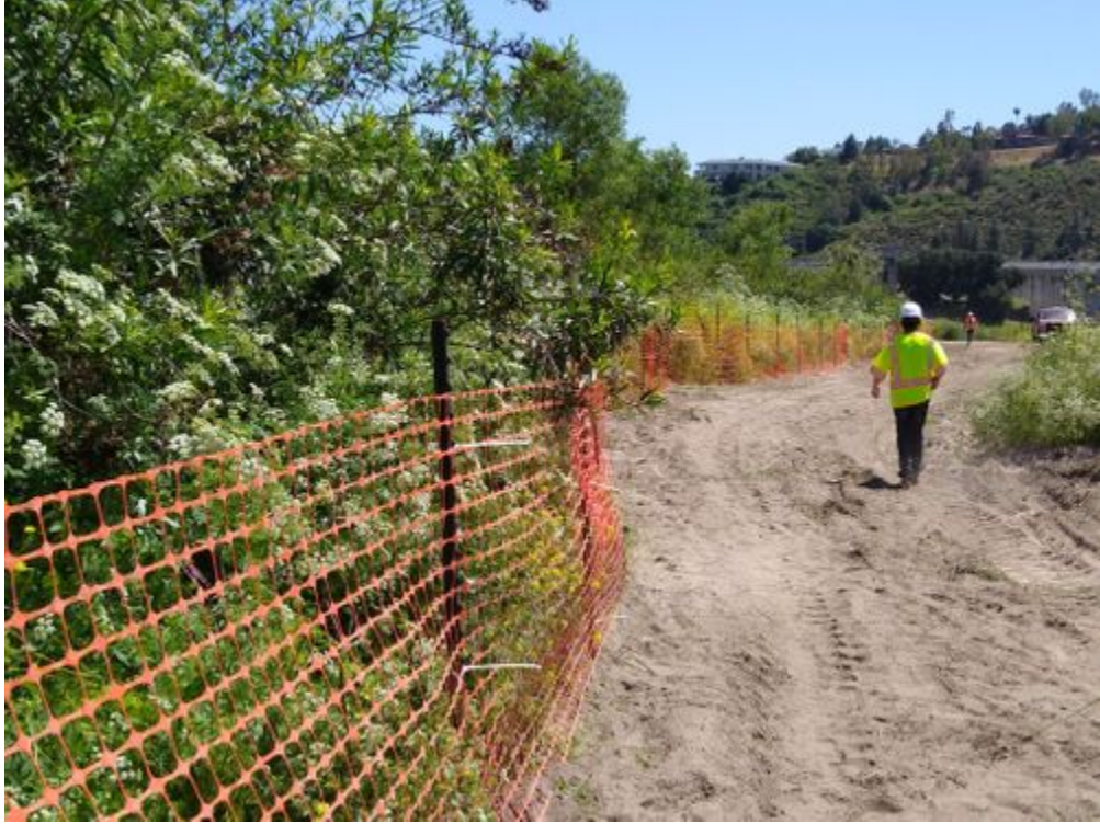
photo_3-esa fence installed.jpg -118.17269 34.18906
