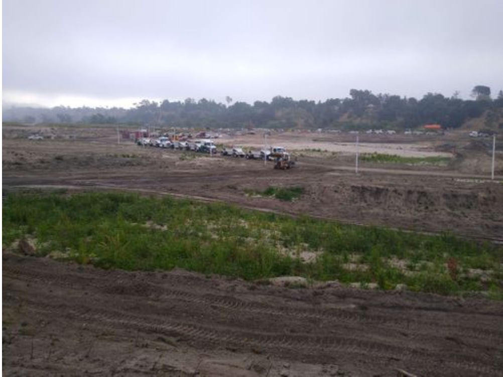
photo_1-start of sediment hauling.jpg -118.17643 34.18815
