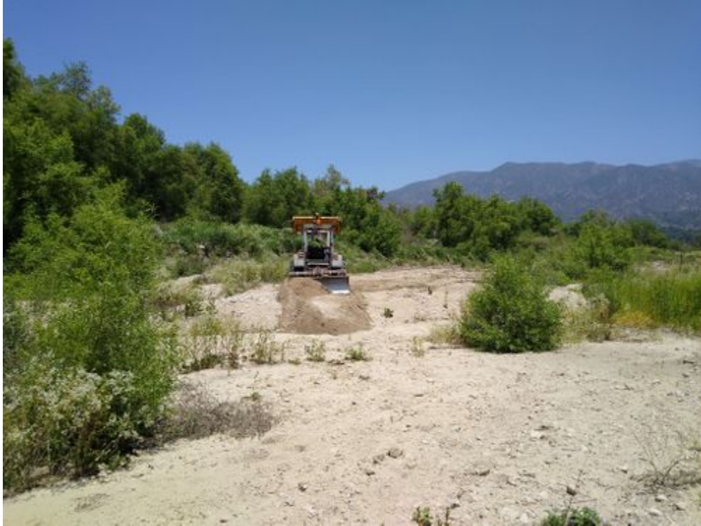
photo_3-clearing of esa fenceline.jpg -118.17671 34.18841
