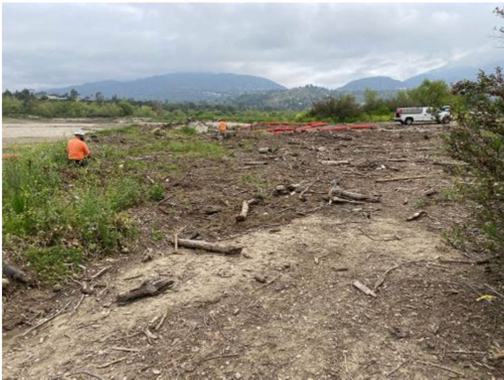
Crew working to remove debris from planted area.jpg -118.17307 34.18738
