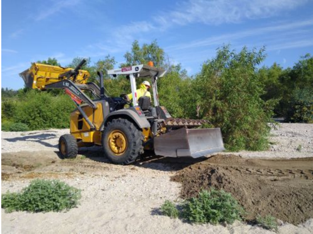
photo_1-clearing esa fenceline.jpg -118.17359 34.19106
