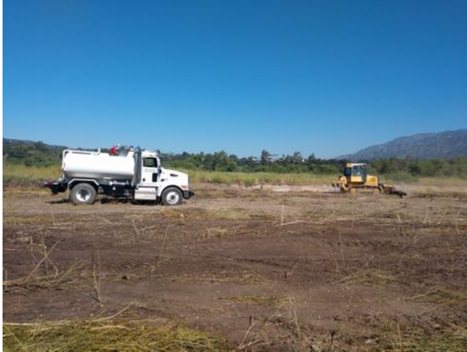
450j and water truck conducting vegetation removal along eastern project boundary -118.17334 34.19893
