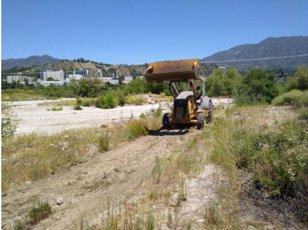
photo_3-clearing esa fenceline.jpg -118.17084 34.19404
