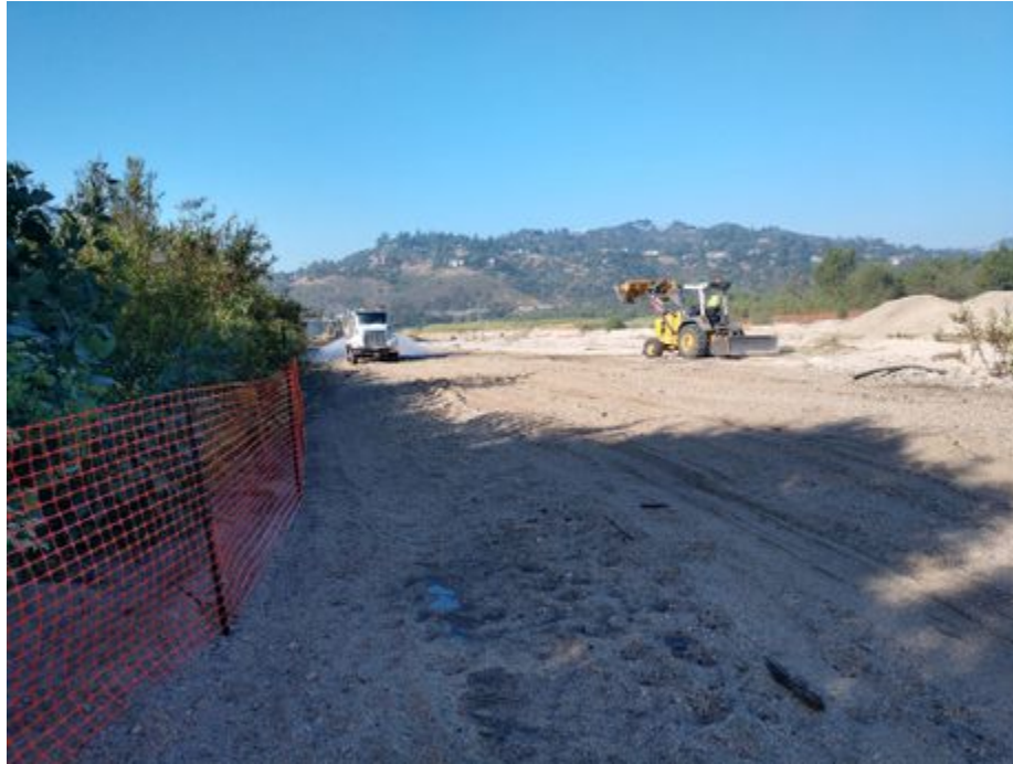
Box scraping and water deposition of potential eastern haul road -118.17249 34.19136
