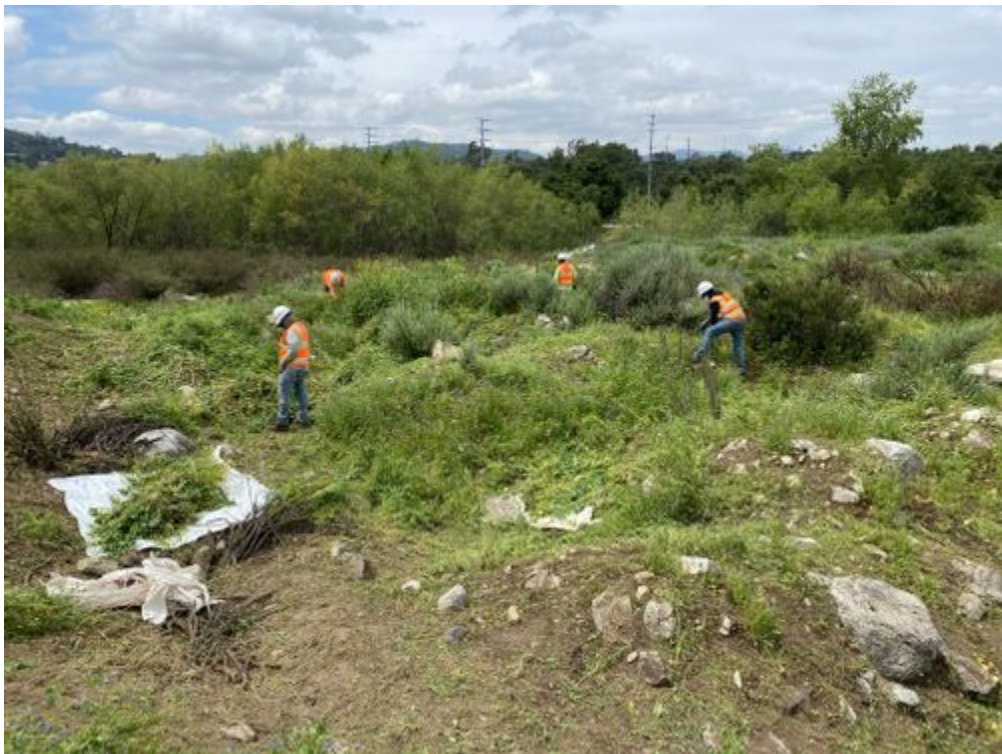
Crew clearing planted area of invasive plants.jpg -118.17295 34.19342
