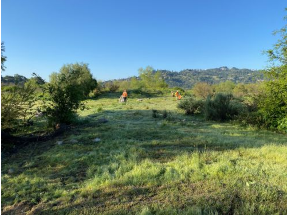
photo_1-Crew clearing vegetation.jpg -118.1725 34.19403
