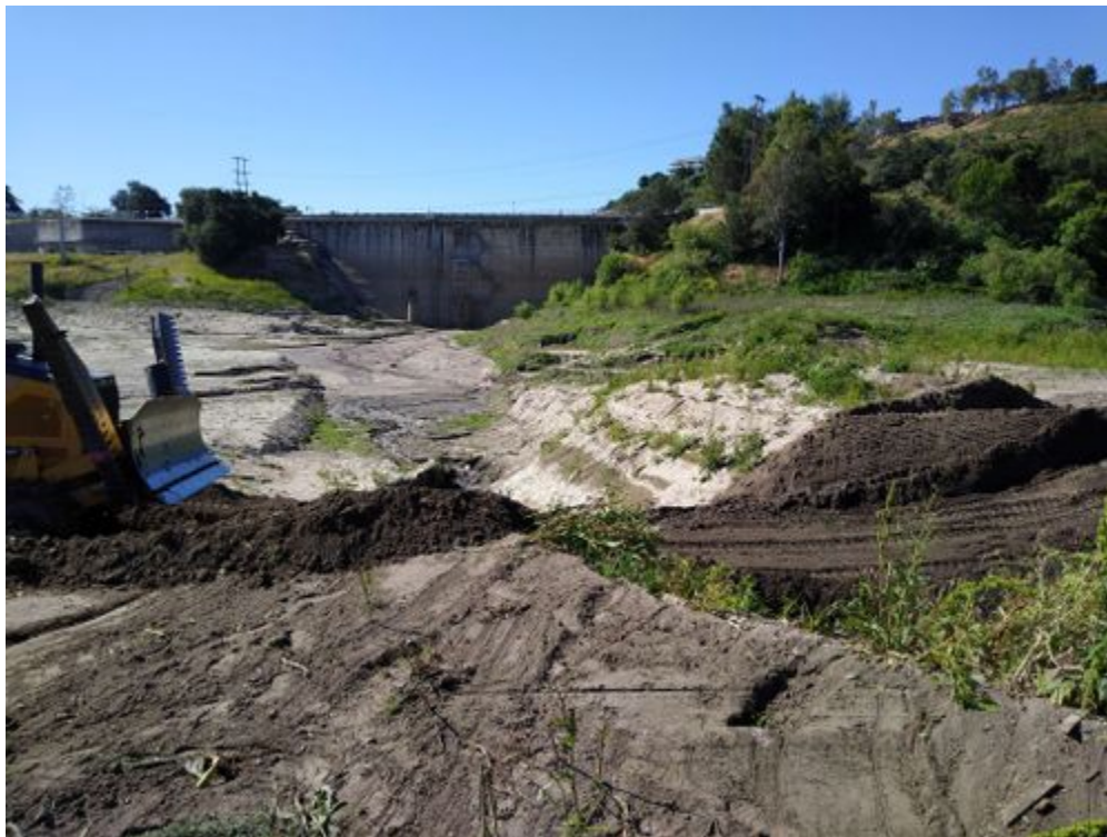
photo_2-clearing west access road.jpg -118.17605 34.1871
