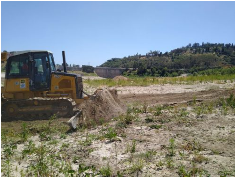
photo_4-backhoe mowing emergent vegetation.jpg -118.17554 34.18942
