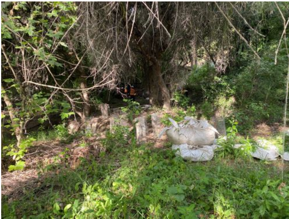
Crew removing non-natives from restoration area.jpg -118.17734 34.1887
