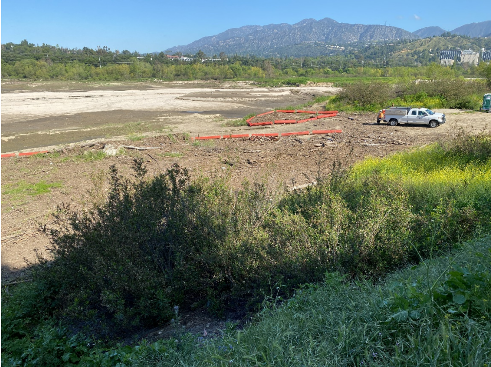
Photo 1_Overview of debris flow DG-3A.jpg -118.173157 34.186587
