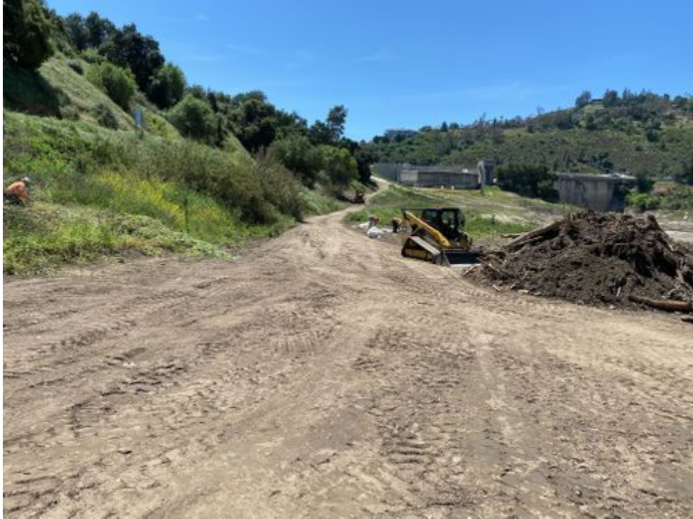
Photo 3_Work area and road after debris removal by DWP.jpg -118.17301 34.18777
