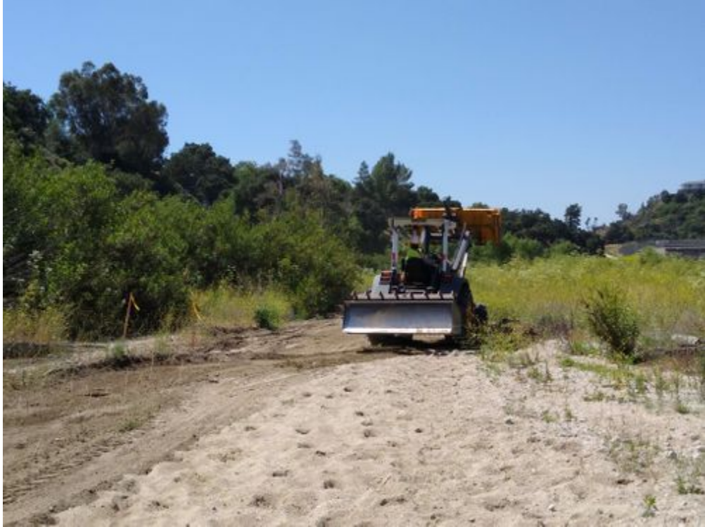
photo_1-backhoe clearing esa line.jpg -118.17266 34.1905
