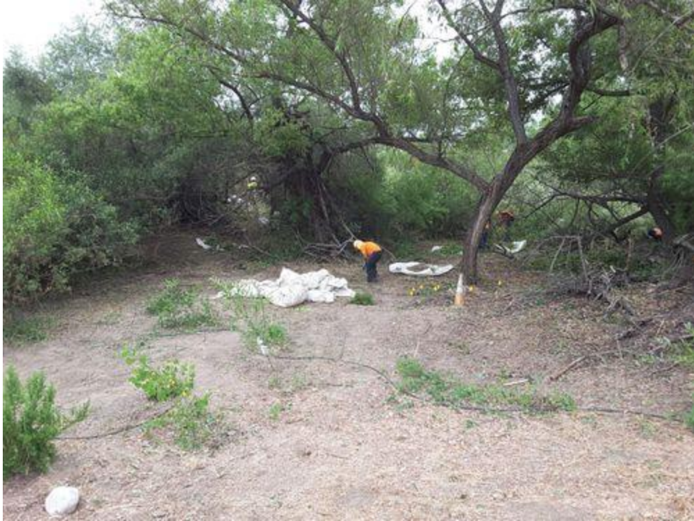
DG-4, DG-4B, during hand pulling looking S.jpg -118.17512 34.19198
