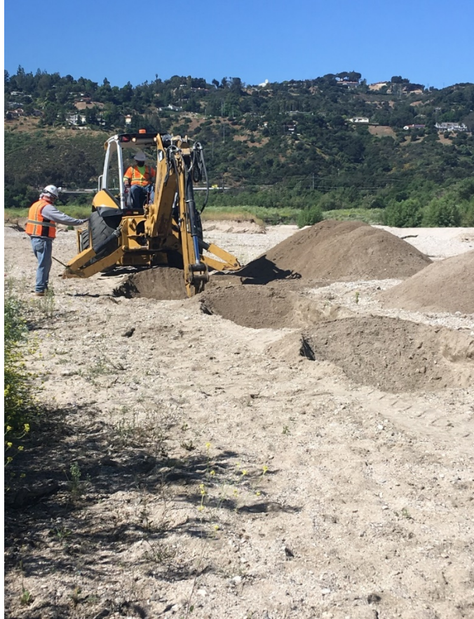
Photo_3-potholing facing S.jpg -118.17344 34.19028
