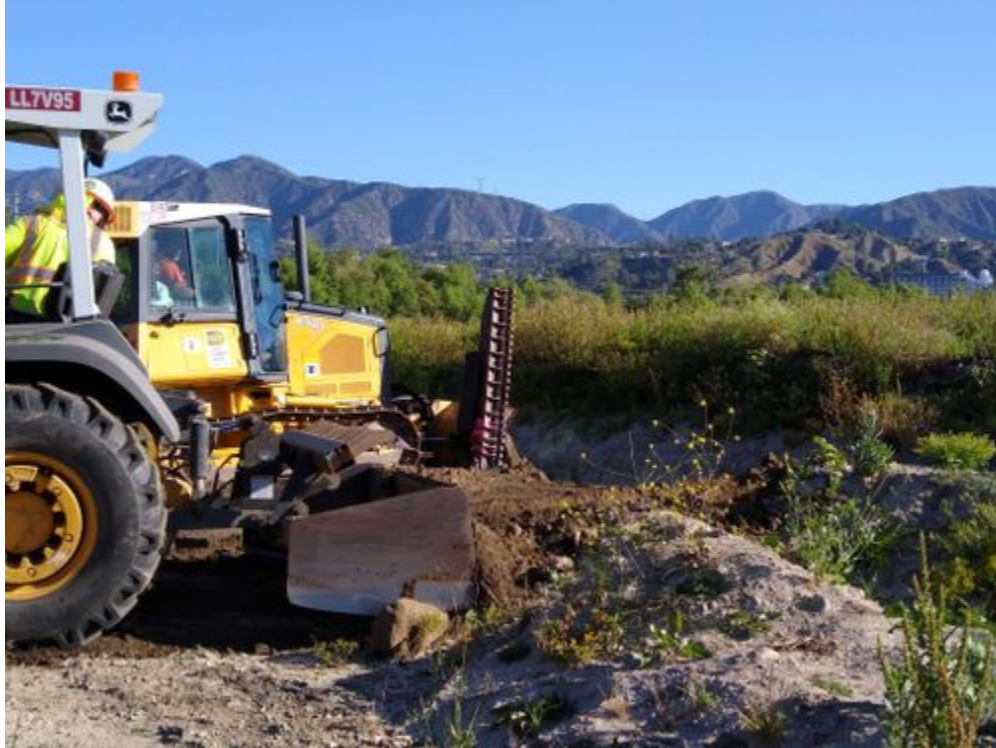
photo_1-pushing emergent vegetation off slope.jpg -118.17616 34.18687
