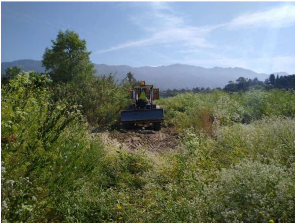
photo_2-clearing esa fenceline.jpg -118.17449 34.19058
