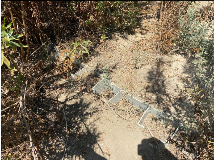
Photo 16: Overview of Grade Control Structure
