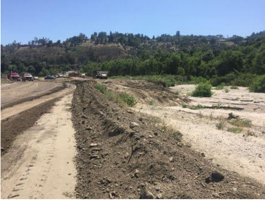
Log Entry Photo D
