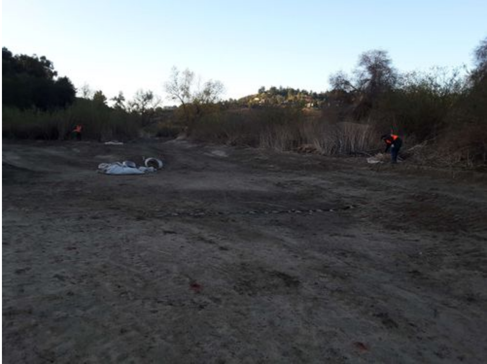
Thatch removal_DG-2 new channels_facing S.jpg -118.17195 34.1909
