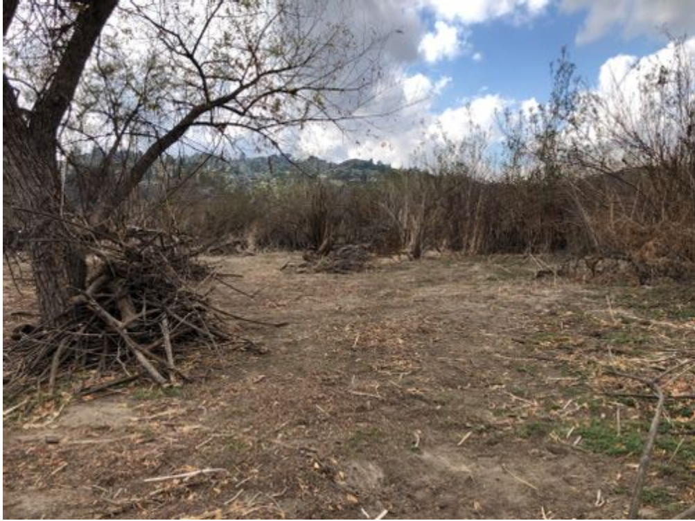
Vegetation clearing after facing S.jpg -118.17223 34.19028
