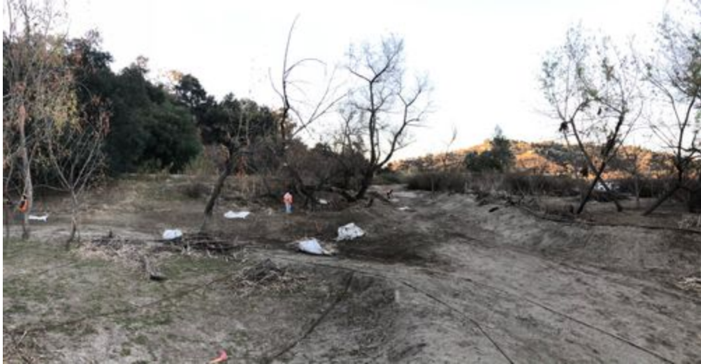
Vegetation clearing_ before_ facingS.jpg
