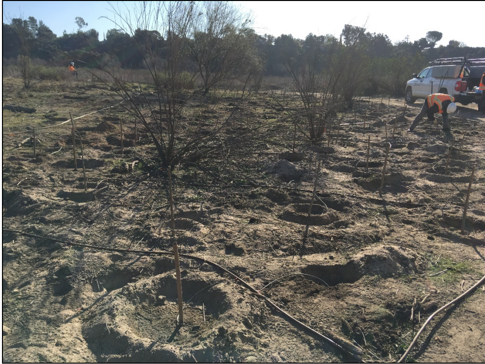
Photo 19. Overview Phase 1 Cutting Installation, facing east.
