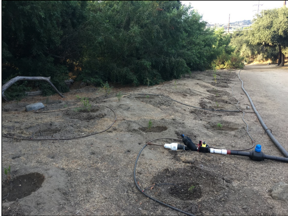
Photo 7. Overview Phase 1 Container Plant Installation, facing south.
