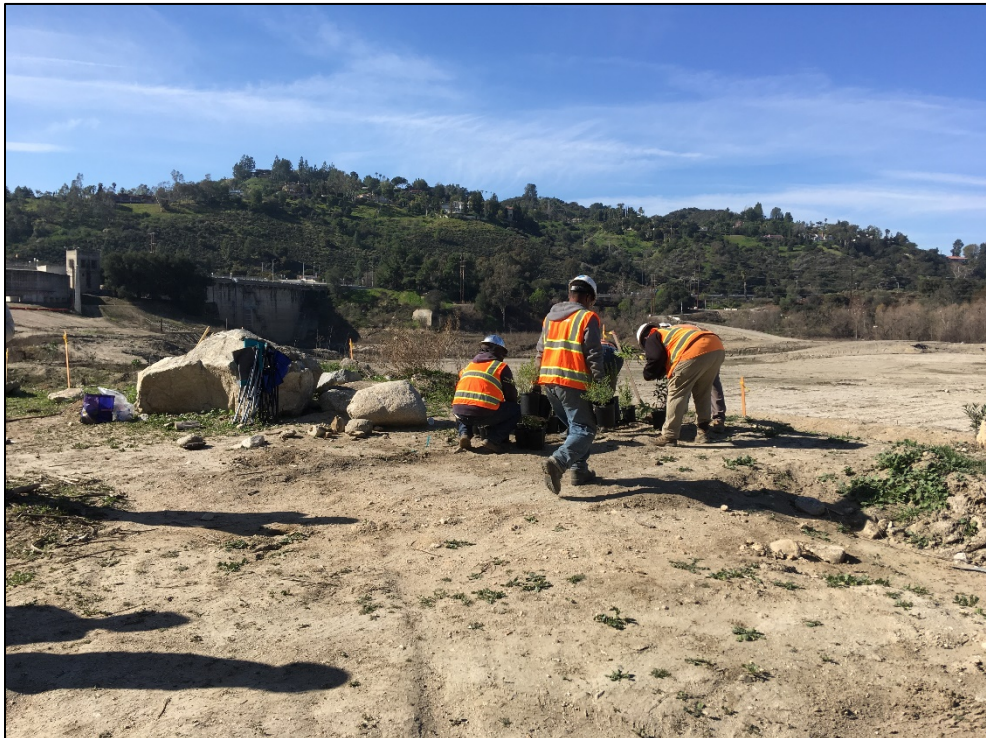
Photo 14. Overview Phase 1 Container Plant Installation, facing northwest.
