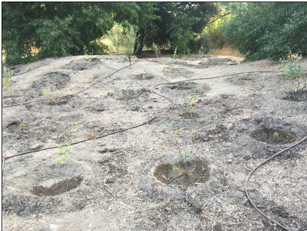
Photo 8. Overview Phase 1 Container Plant Installation, facing east.
