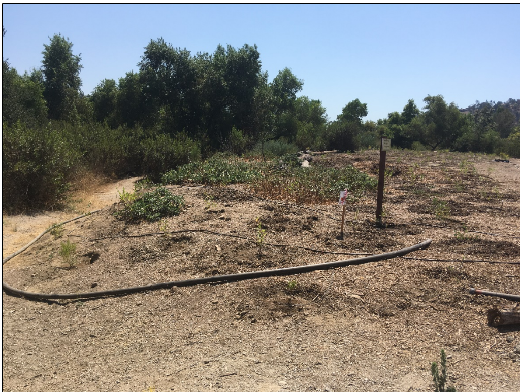
Photo 10. Overview Phase 1 Container Plant Installation, facing southeast.
