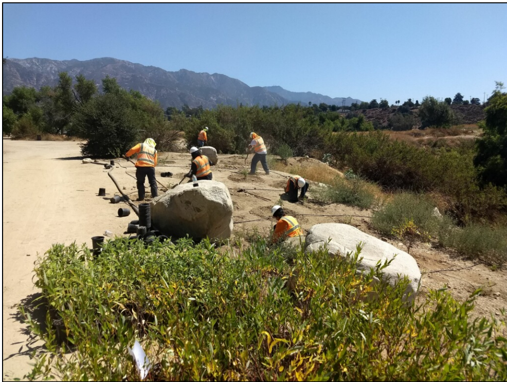
Photo 12. Overview Phase 1 Container Plant Installation, facing north.
