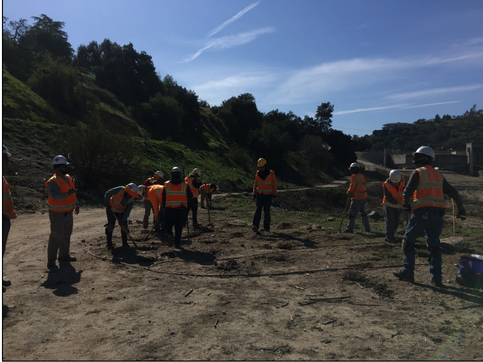
Photo 15. Overview Phase 1 Container Plant Installation, facing south.
