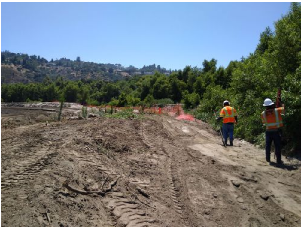
photo_4-ESA fence restoration.jpg -118.17598 34.18923
