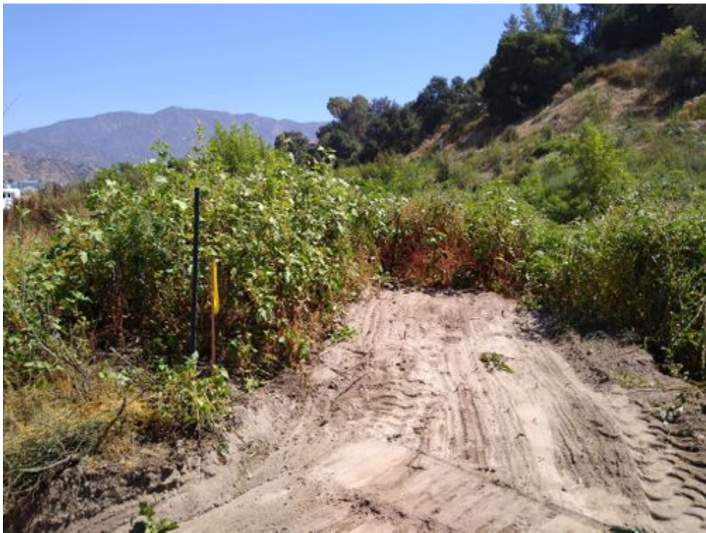
photo_2-esa fence installation.jpg -118.17358 34.18693
