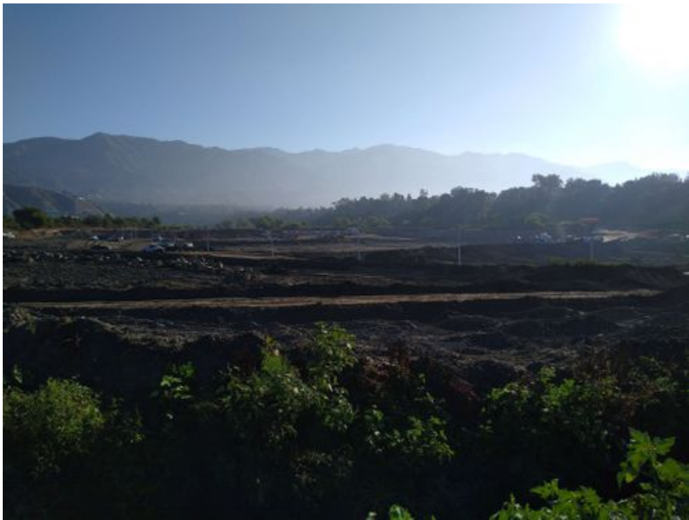
photo_2-sediment hauling activities.jpg -118.17635 34.18707
