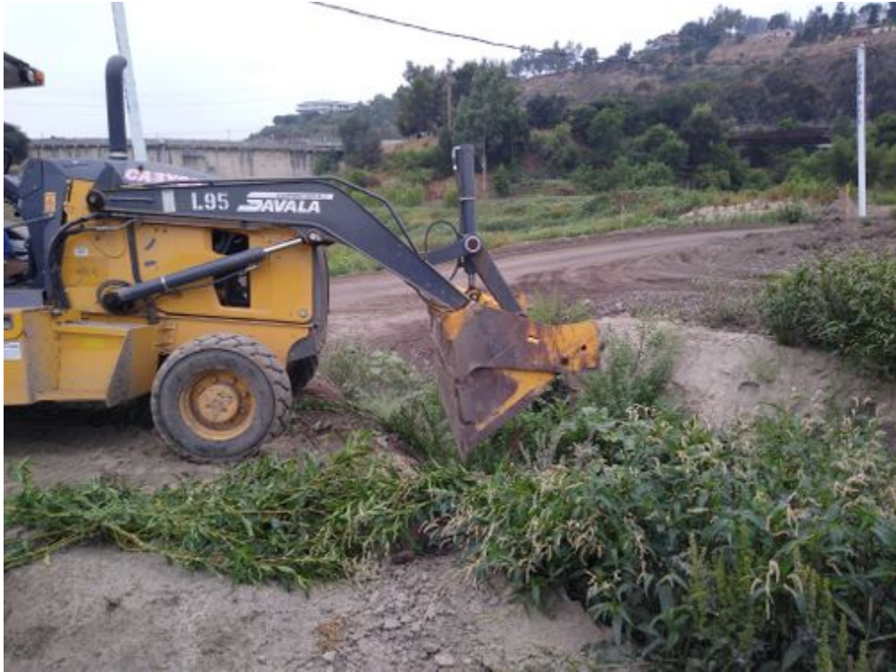
photo_1-emergent vegetation removal.jpg -118.17577 34.18724
