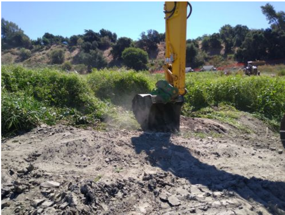
photo_2-excavator clearing vegetation.jpg -118.17454 34.1867
