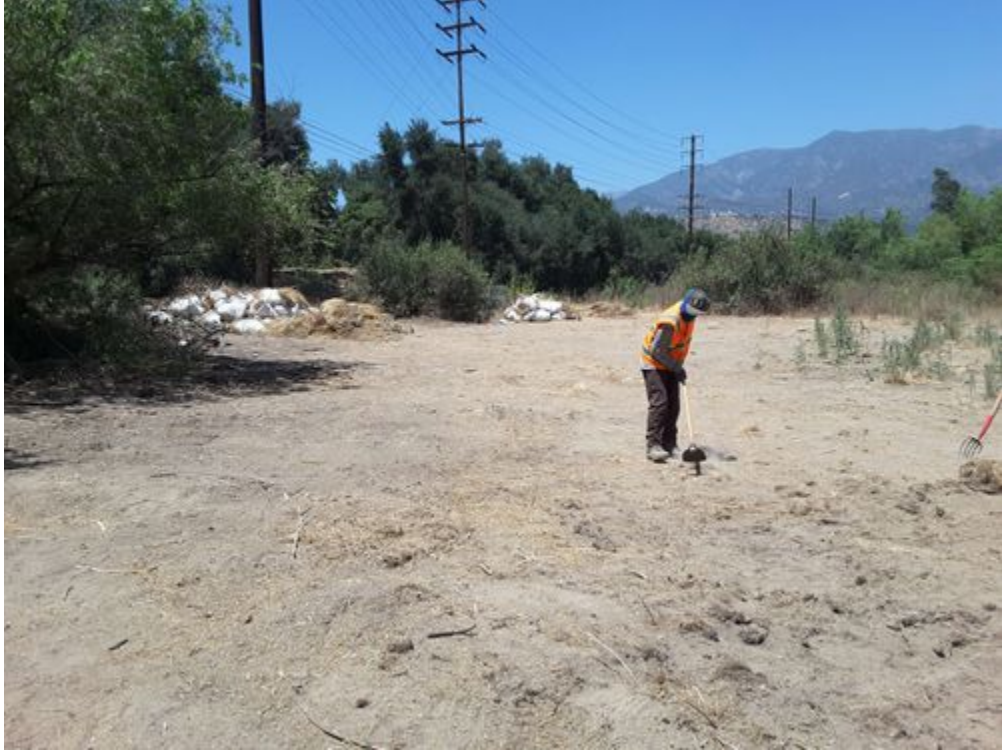
After clearing piles from yesterday, facing N.jpg -118.17695 34.19045
