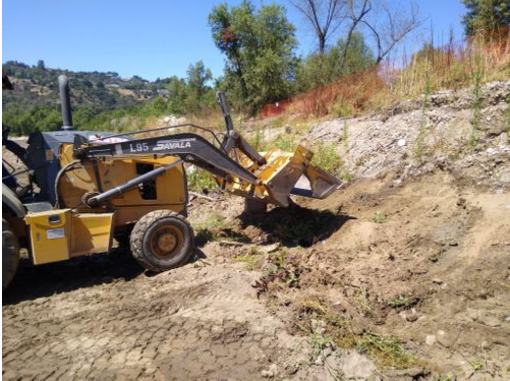
photo_3-vegetation clearing west of scalehouse.jpg -118.17535 34.18974
