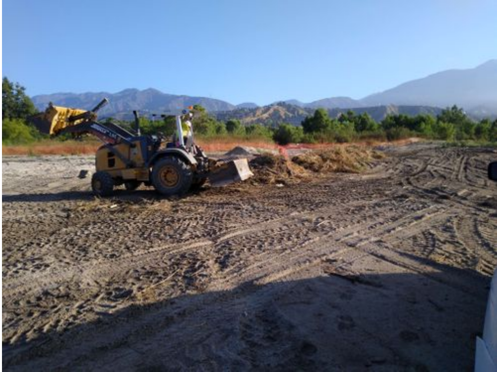
Photo_1-removal of debris piles.jpg -118.17445 34.18993
