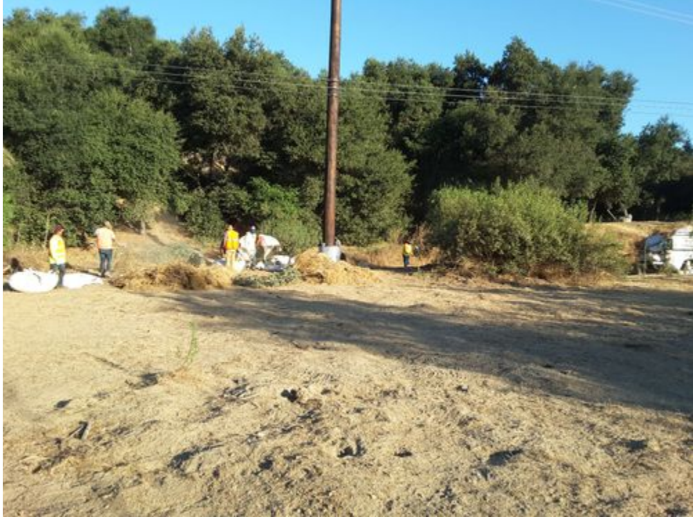
Crew hauling tarps from previous week to dumpster.jpg -118.17678 34.19063
