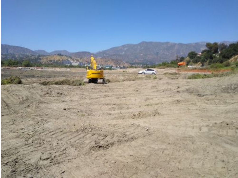
photo_3-work area post removal.jpg -118.17427 34.18635
