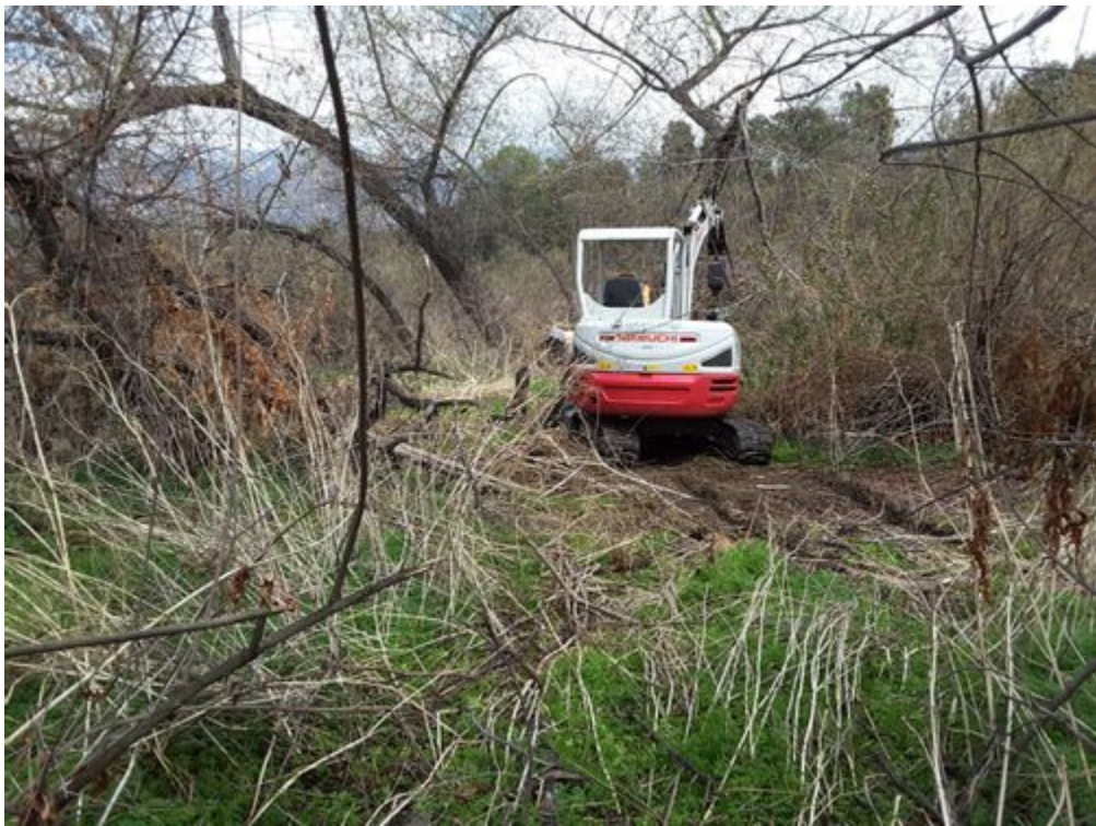
Clearing non-native vegetation for planting_DG-2_facingNE.jpg -118.17257 34.19132
