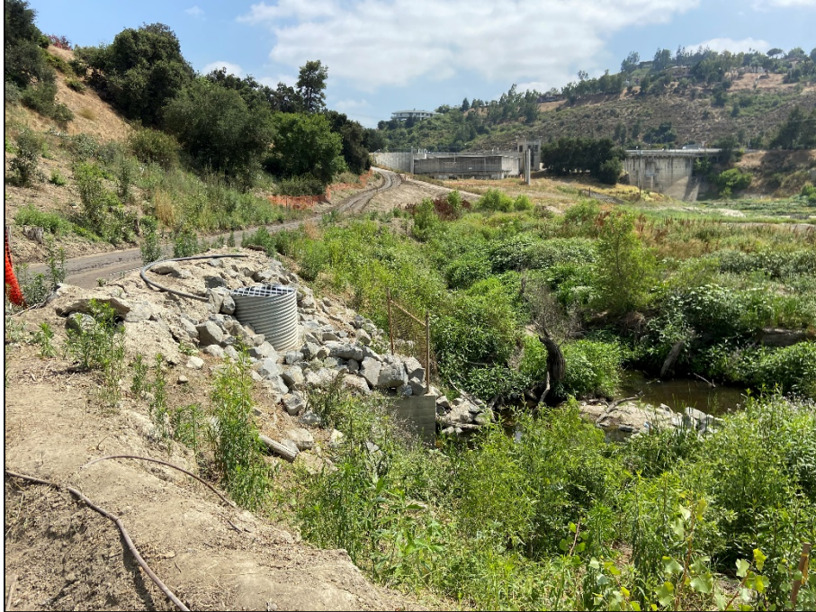
Photo 11: Overview Mitigation Area DG-3A Altadena Drain
