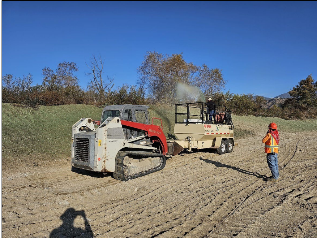
Photo 10: Phase 3, Side Slopes during hydroseeding.
