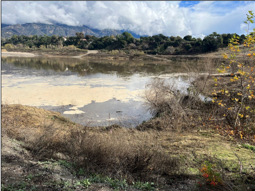
Photo 16: Phase 3, Flint Wash after hydroseeding.
