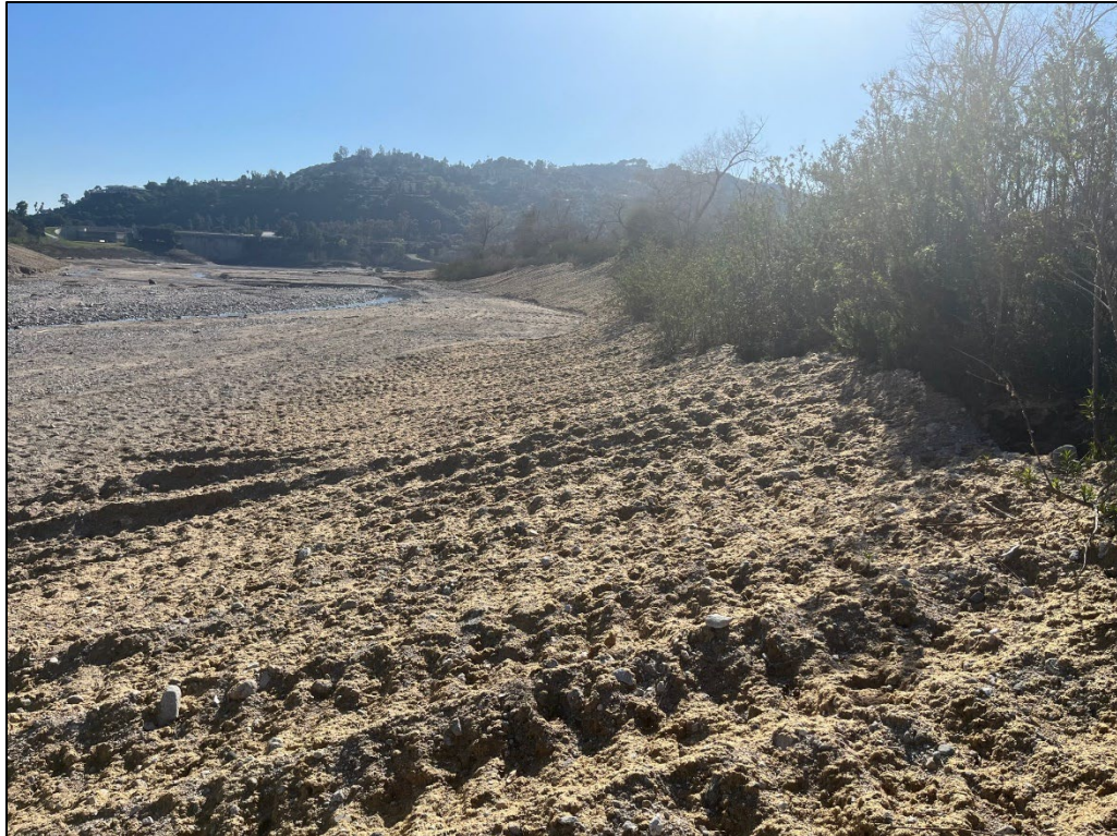
Photo 12: Phase 3, Side Slopes after hydroseeding.
