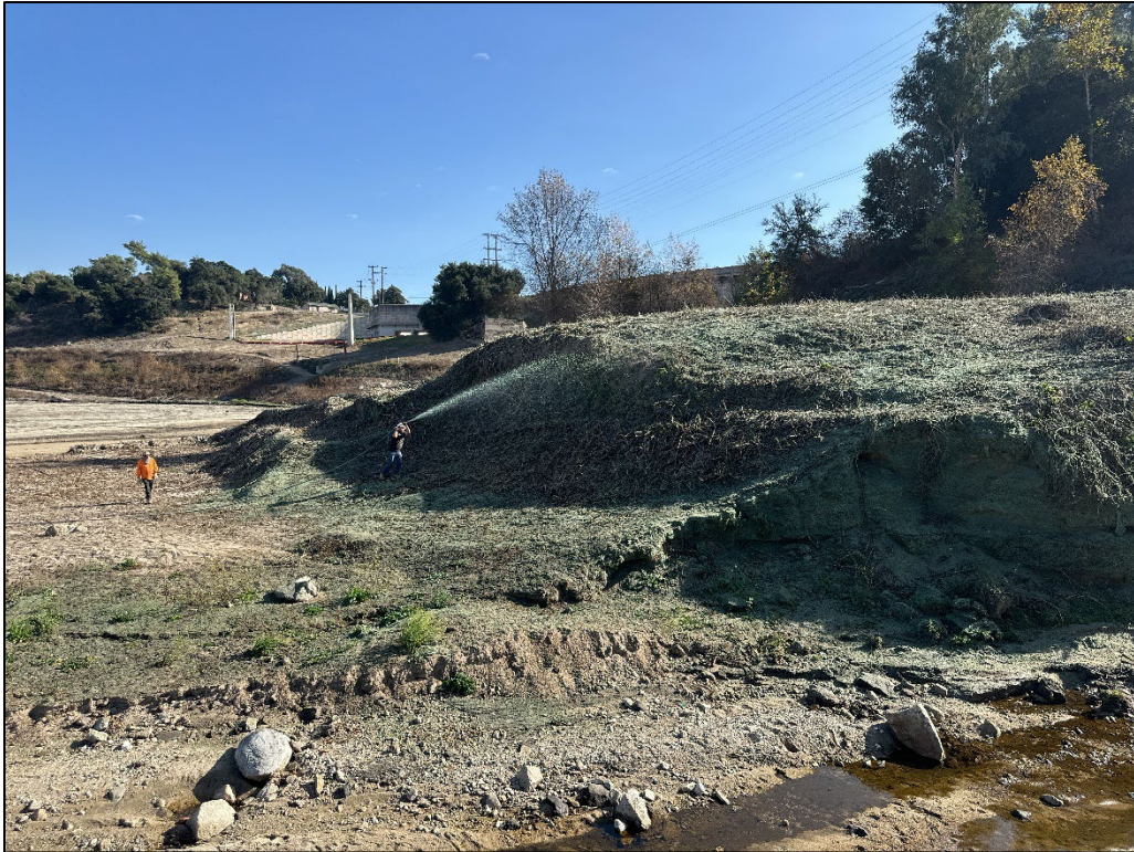
Photo 14: Phase 3, Flint Wash during hydroseeding.
