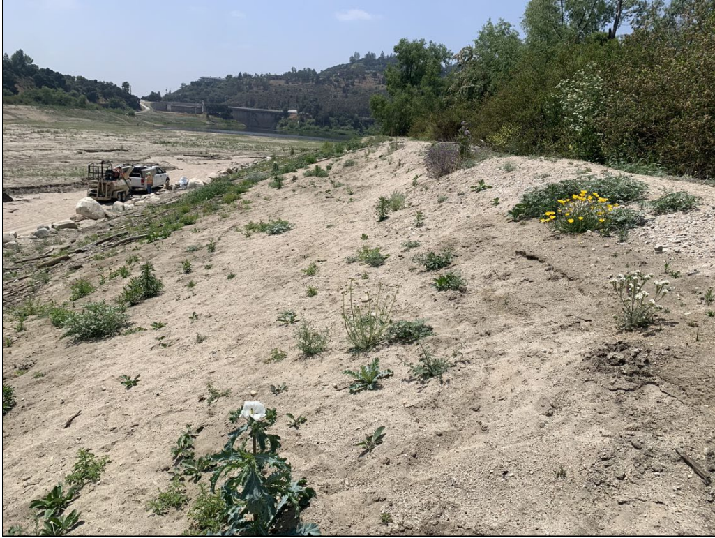
Photo 9. Phase 3, Side Slopes before hydroseeding.
