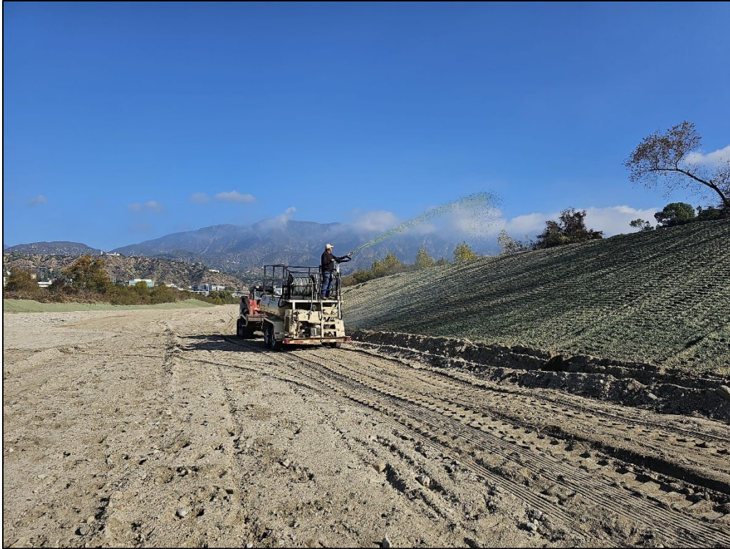
Photo 11. Phase 3, Side Slopes during hydroseeding.
