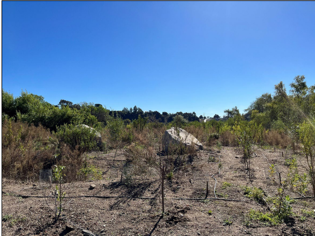
Photo 8: Phase 3, DG-4A after container plant installation.
