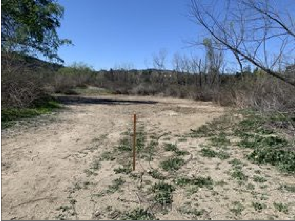
Photo 3: Phase 3, DG-4 WOUS connections before container plant installation.
