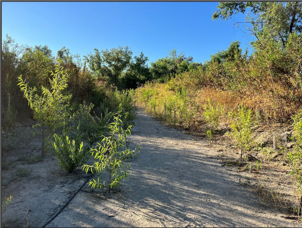
Photo 6: Phase 3, DG-4 WOUS connections after container plant installation.
