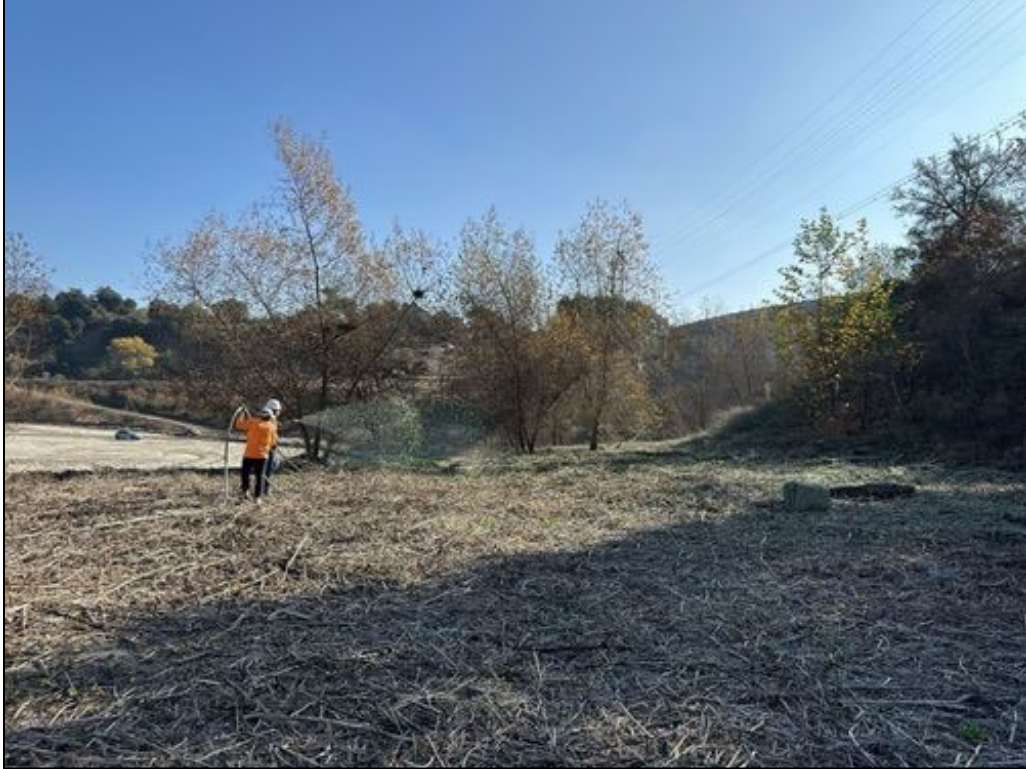
Photo 15: Phase 3, Flint Wash during hydroseeding.
