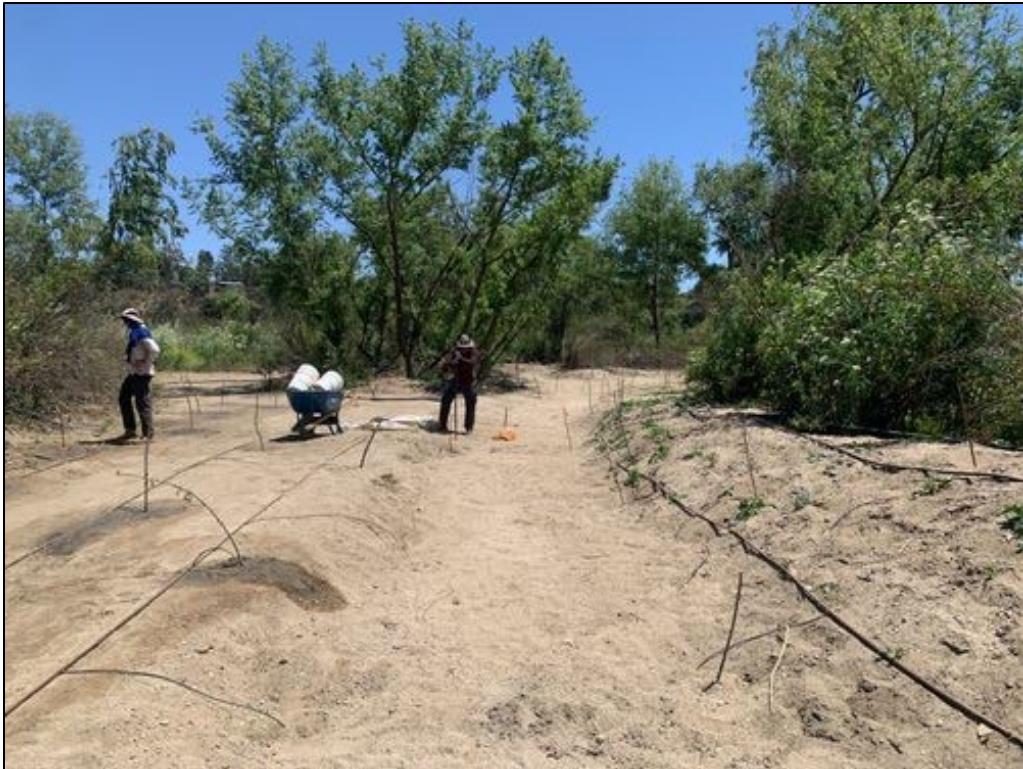
Photo 2: Phase 3, DG-4 WOUS after container plant installation.
