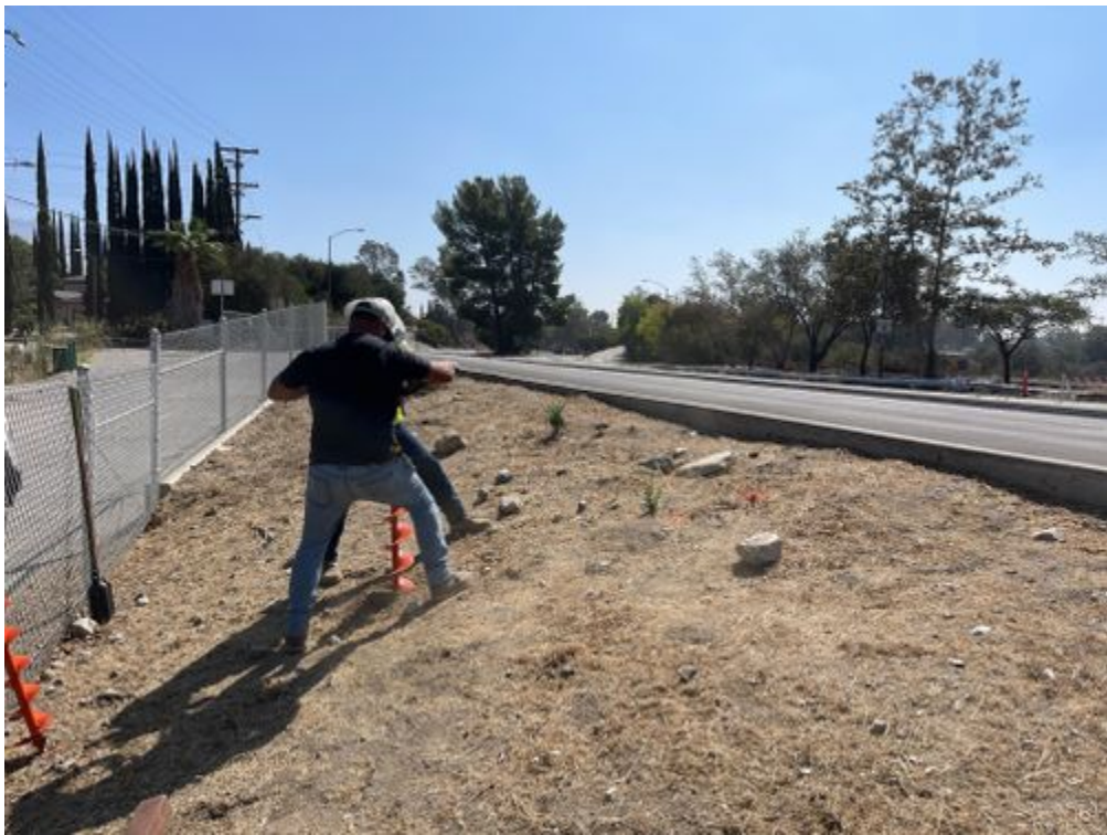
Using_gas_powered_earth_auger_to_dig_hole_for_roadside_sign_091621.jpg -118.17350883333334 34.185101113888884
