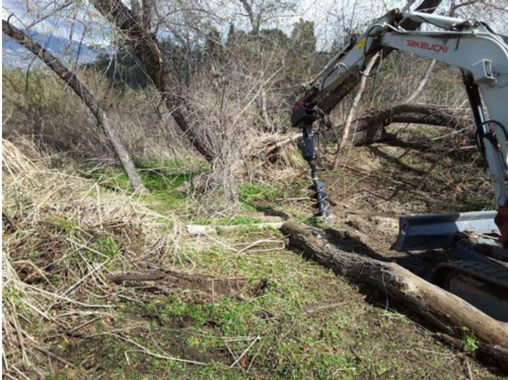
Area cleared_vegetation piled_holes started.jpg -118.17239 34.19106
