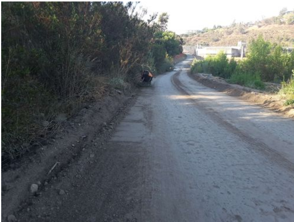
Trimming vegetation for fence.jpg -118.17306 34.18747
