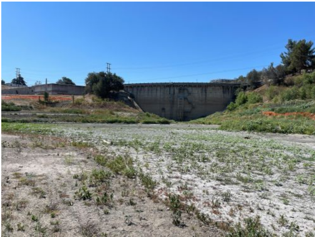
Southern end of site_063021.jpg -118.17542 34.18669
