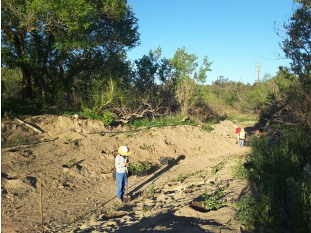
Prepping to plant_DG-W-2_facing W.jpg -118.17531 34.19155
