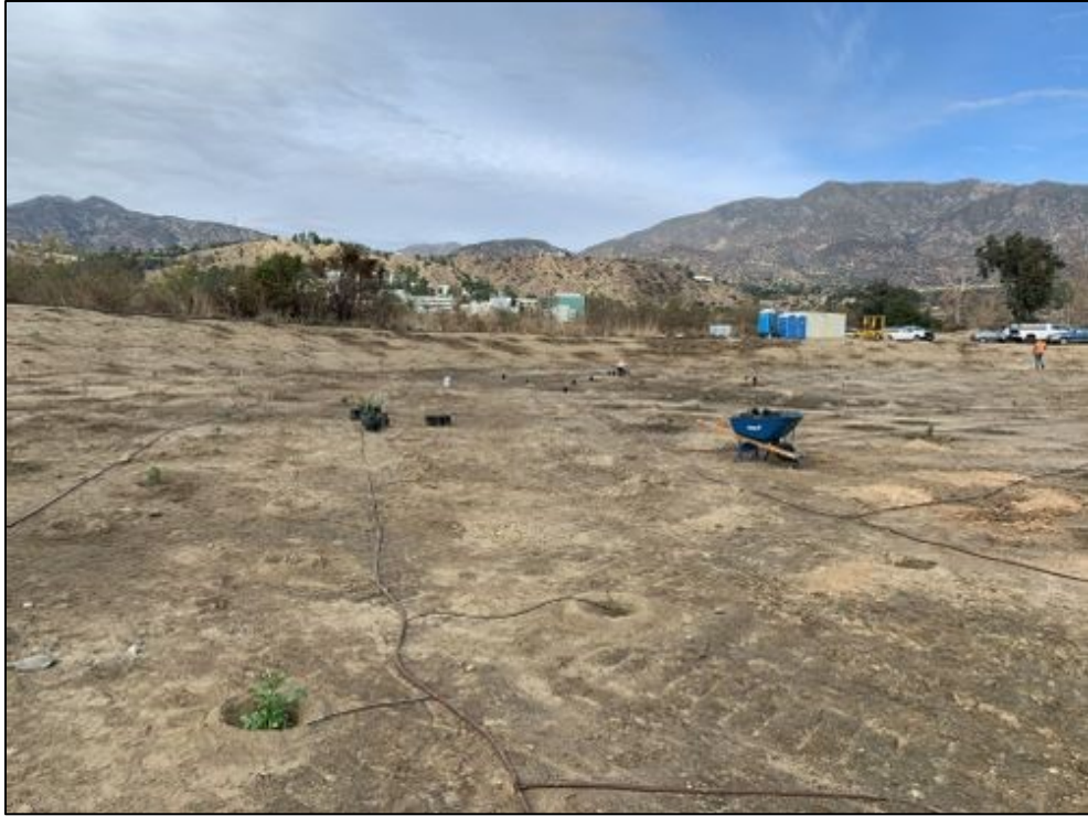
Photo 3. Overview Phase 2 Container Plant Installation
