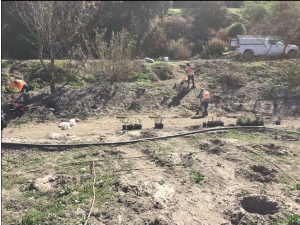
Photo 9. Overview Phase 2 Container Plant Installation
