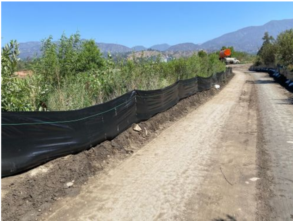
07-06-2021_silt_fence_installation_complete_facingN.jpg
