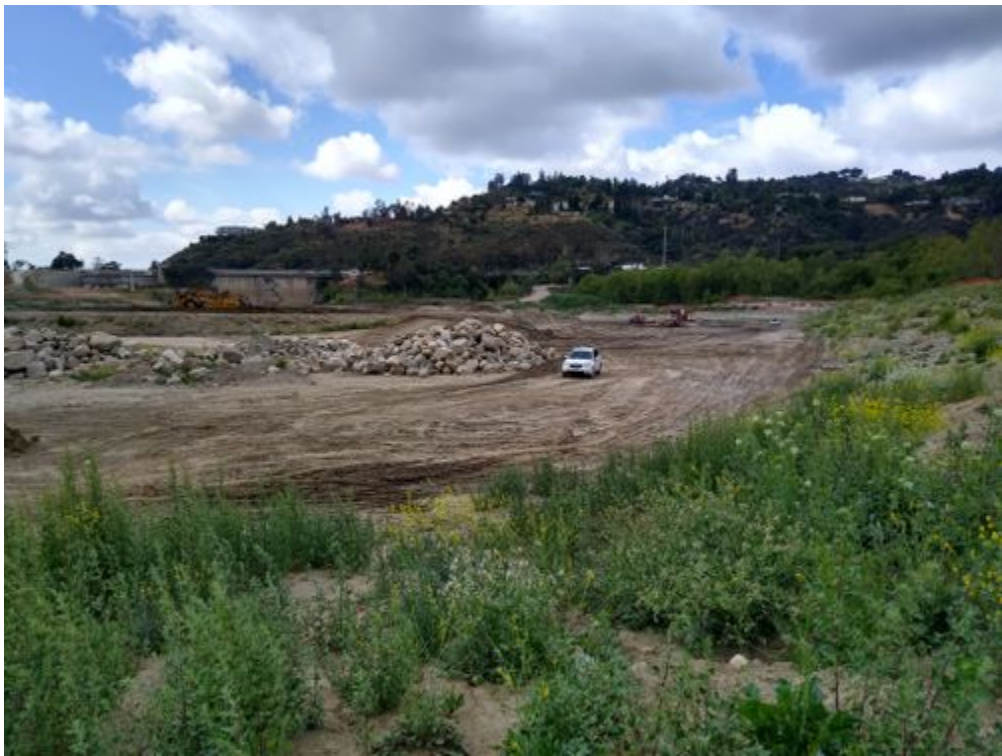
photo_2-scalehouse prep overview.jpg -118.17452 34.19029
