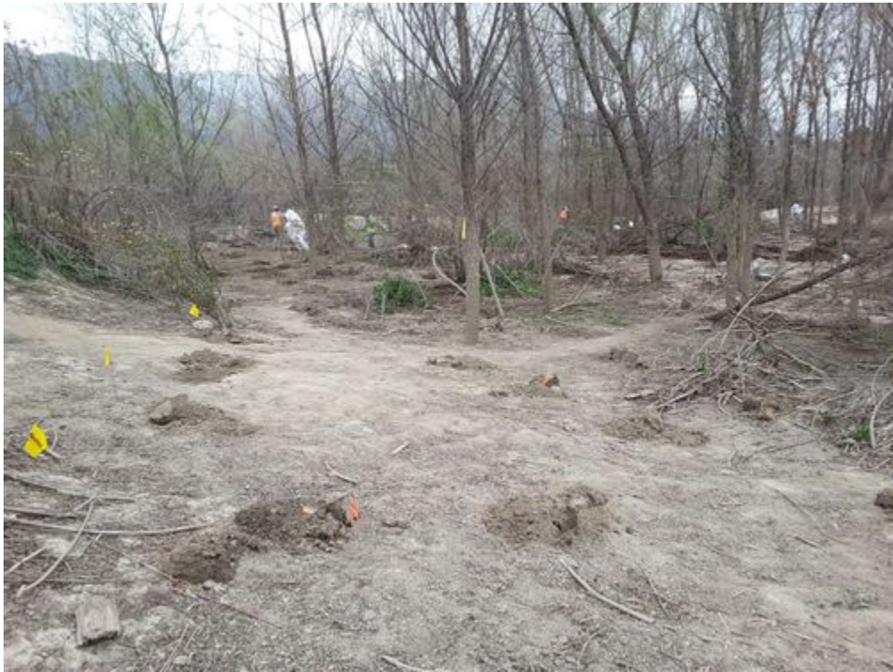
Site prep progress_facing N.jpg -118.17451 34.19327
