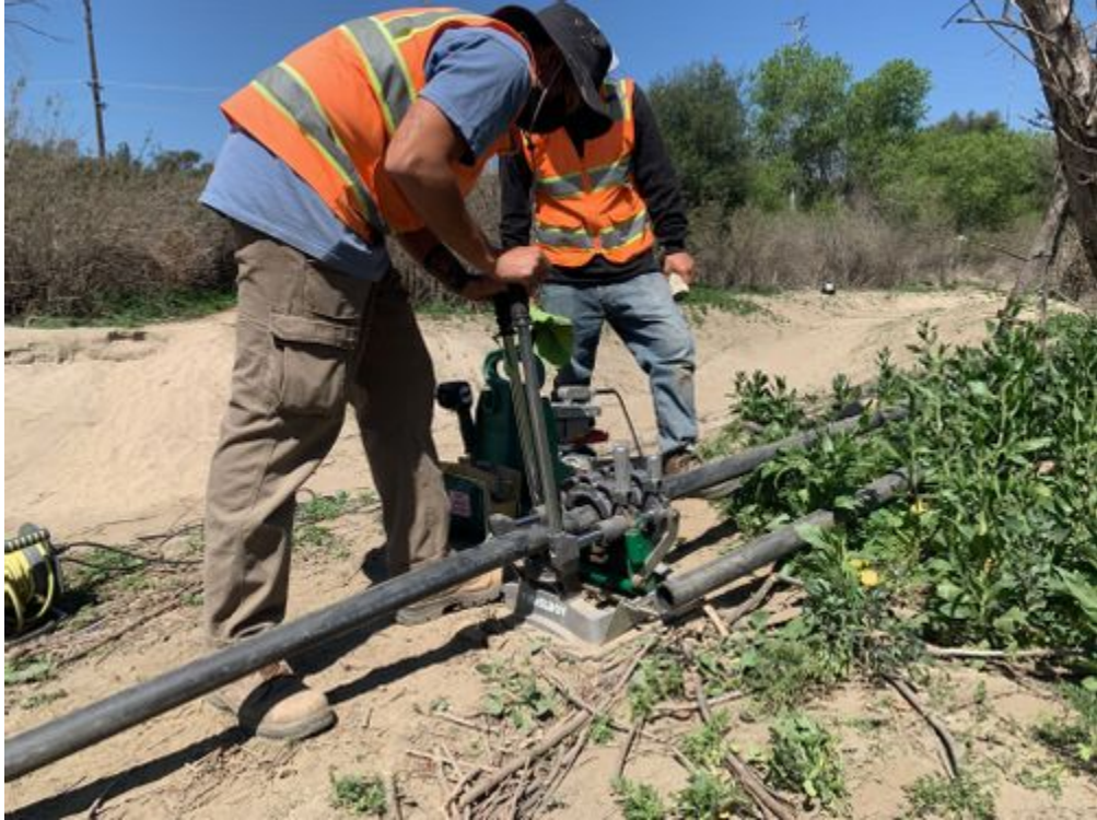
photo_3-crew_fusing_pipe_facingW.jpg -118.17456 34.19246
