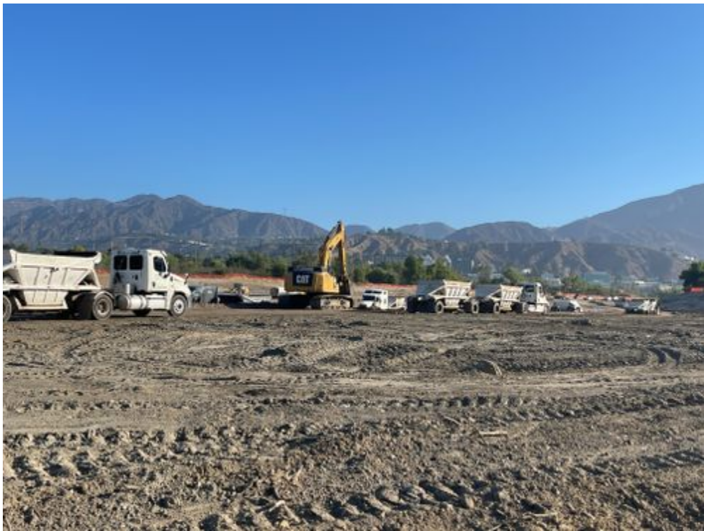
Excavator loading haulers_070721.jpg -118.17336 34.18867
