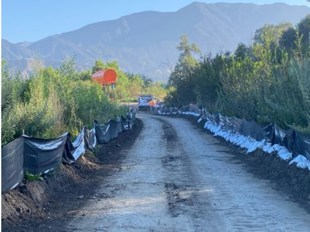
07-06-2021_silt_fence_installation_facingN.jpg
