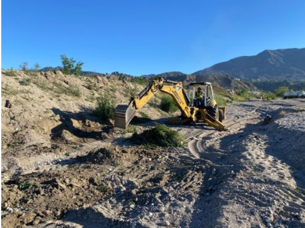
Backhoe_clearing_vegetation_facingN.jpg
