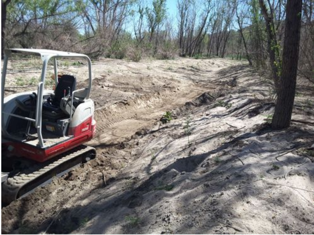
Drainage in progress.jpg -118.17411 34.19312
