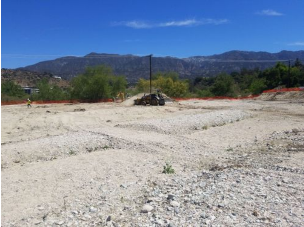
photo_3-20210430-182150looking north at backhoe and skiploder.jpg -118.17125 34.19417
