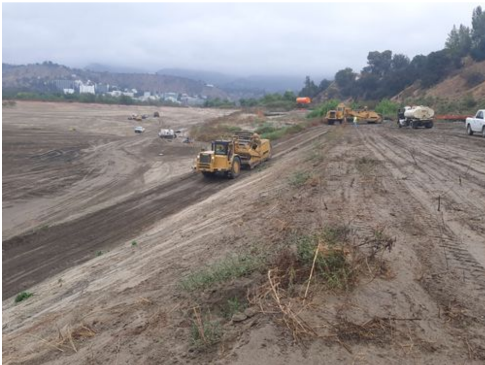
Scrapers_adding_fill_to_road_ramp_on_eastern_side_facing_north.jpg -118.17415 34.18618
