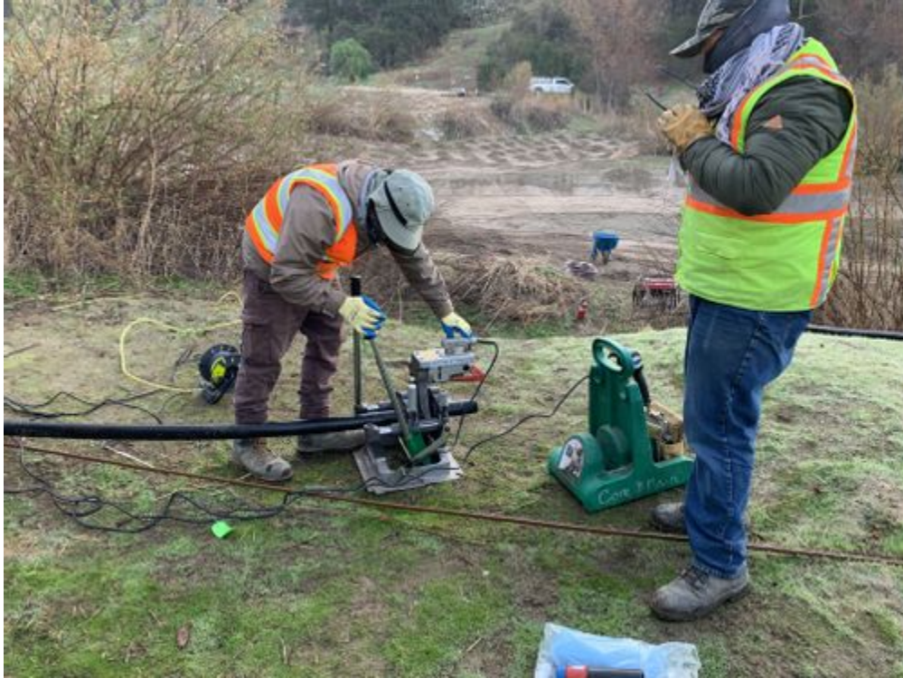
photo_1-crew_fusing_pipe_facingW.jpg -118.17202 34.19072
