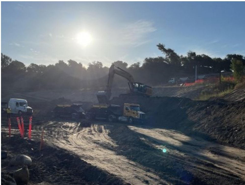
Excavator loading dirt_southern section_072221.jpg -118.17533047222223 34.18597534722222
