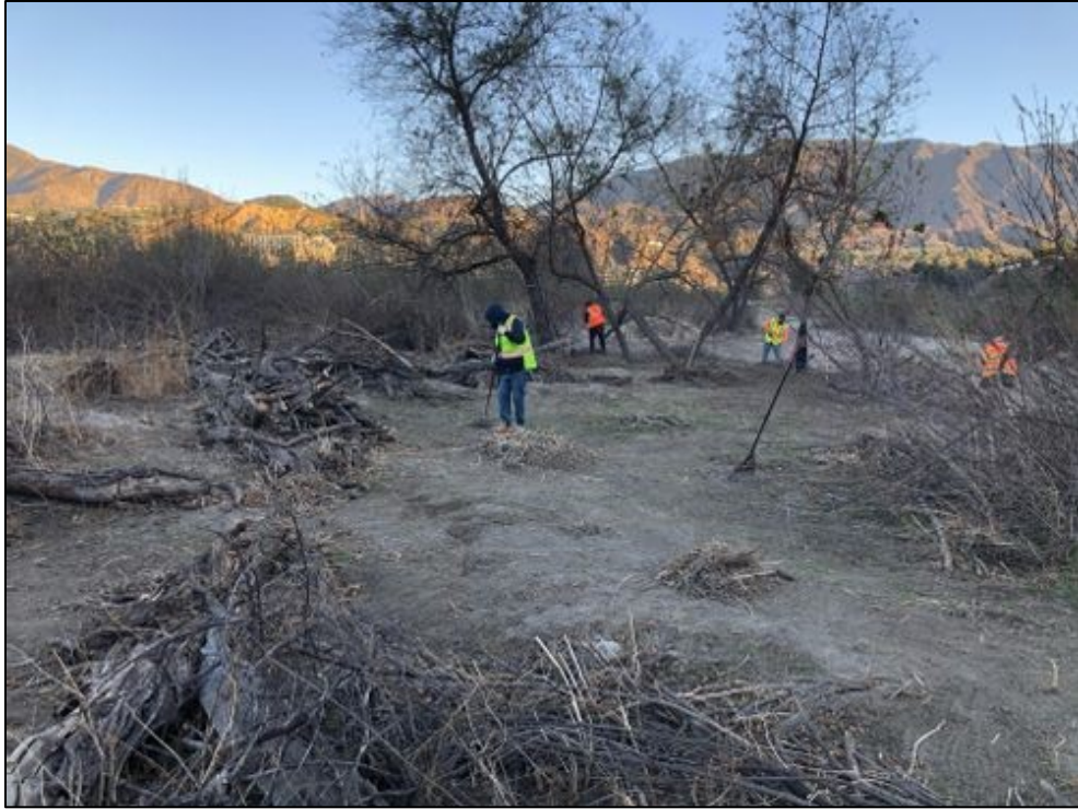
Photo 15. Overview Phase 2 Weed Abatement
