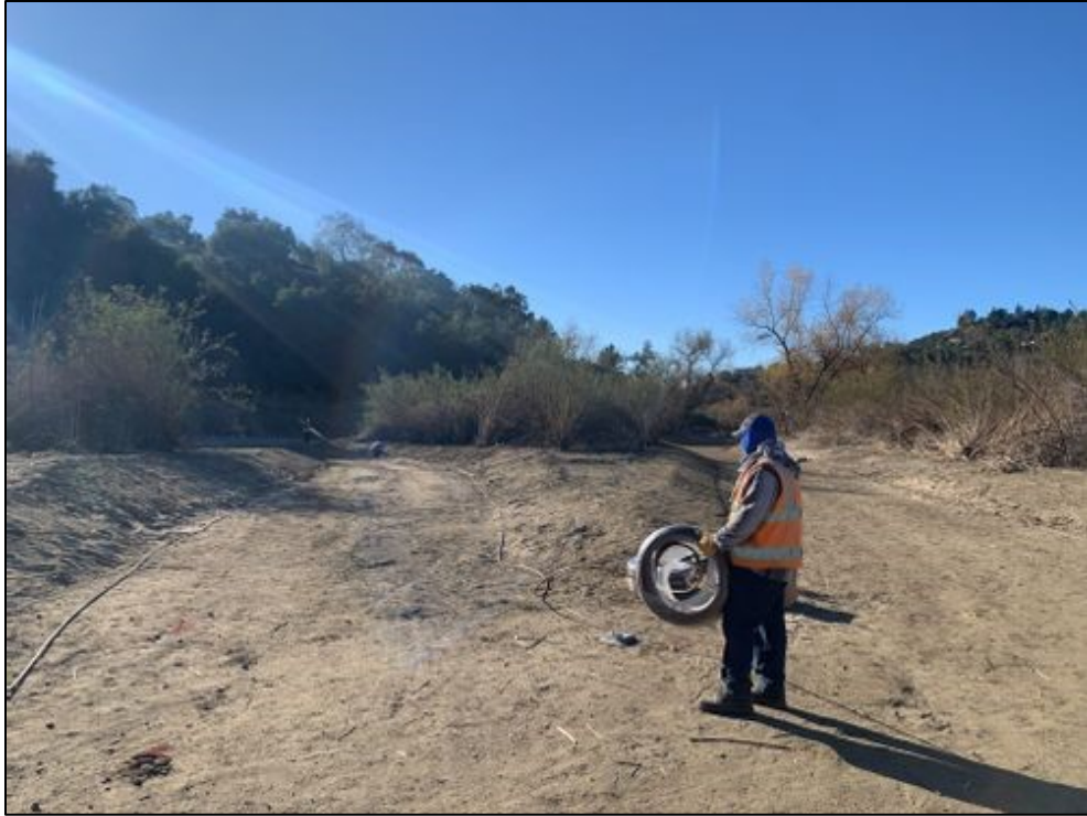
Photo 1. Overview Phase 2 Irrigation Installation
