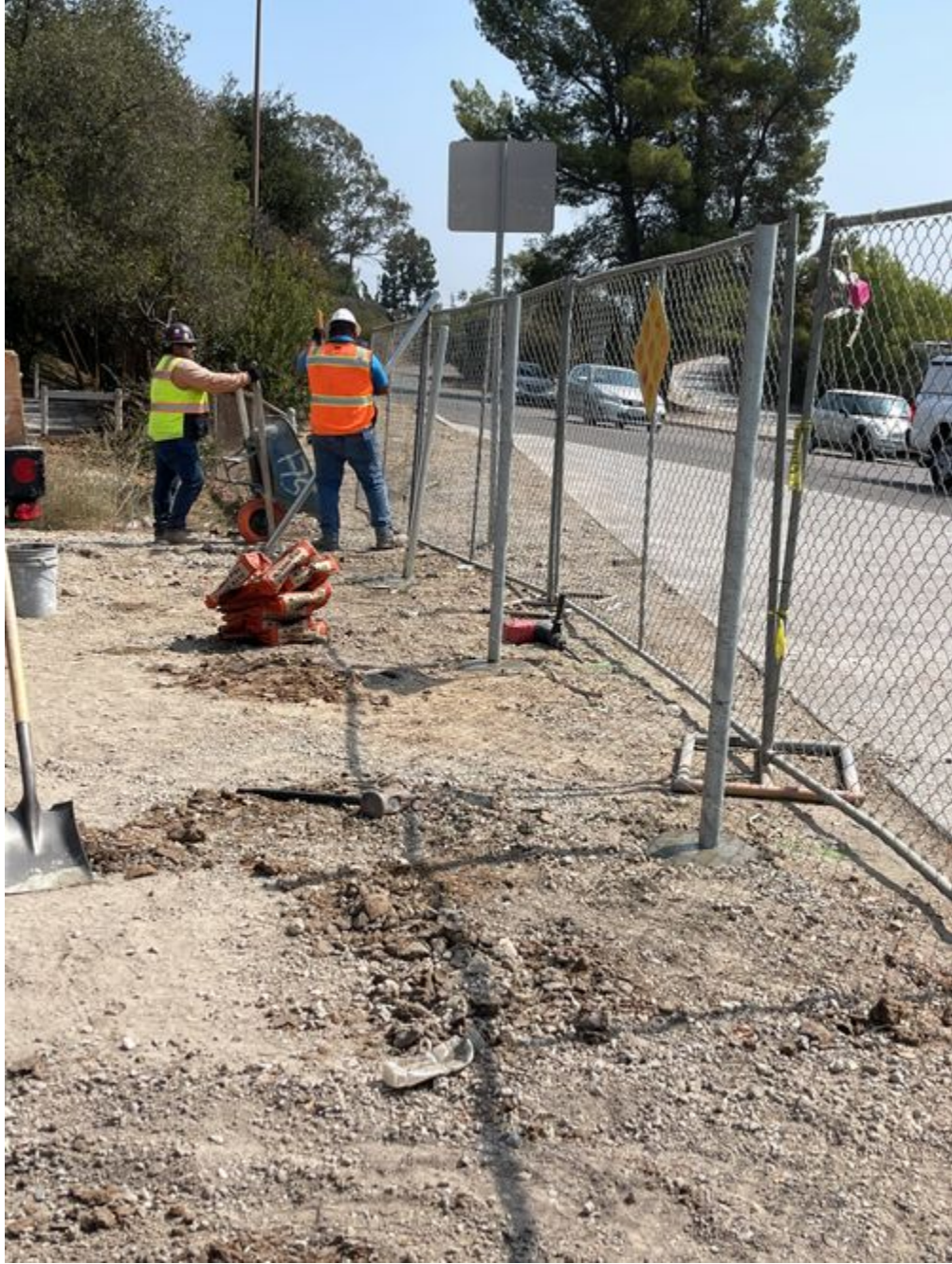
Pouring_concrete_for_fence_posts_by_main_road_092921_Ace fencing.jpg
