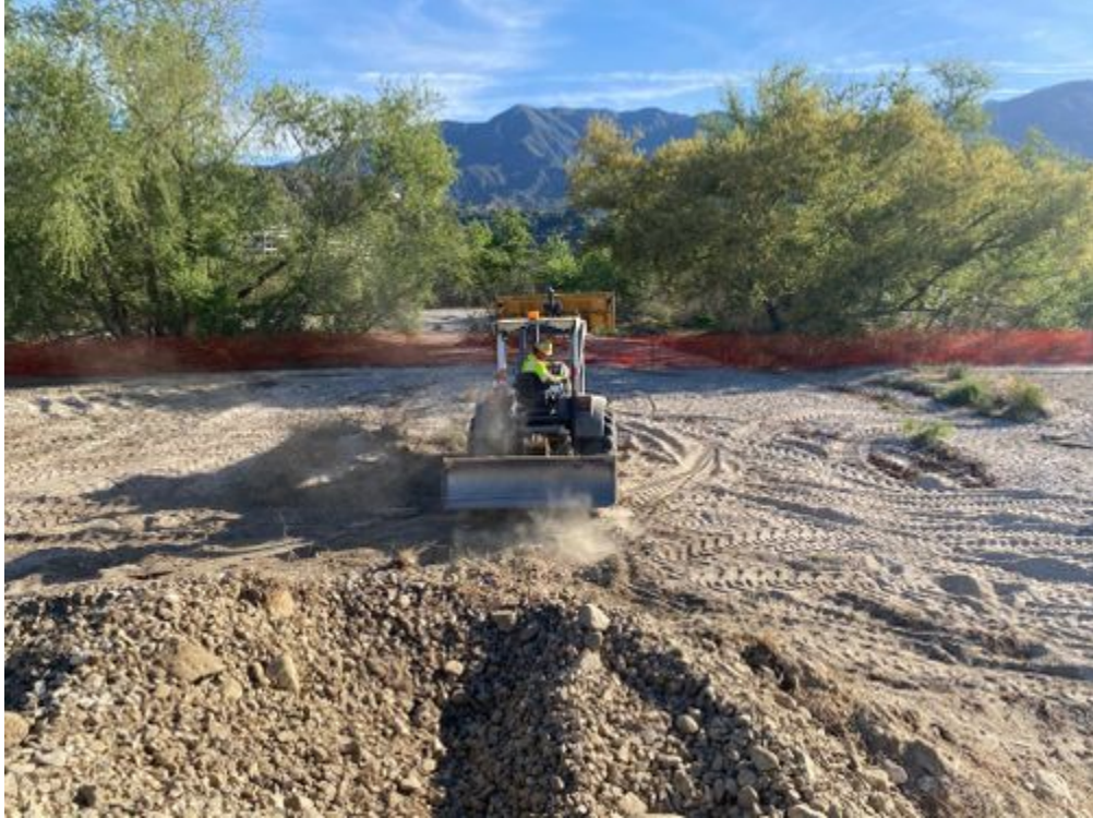
Skip_loader_removing_vegetation_piles_facingN.jpg
