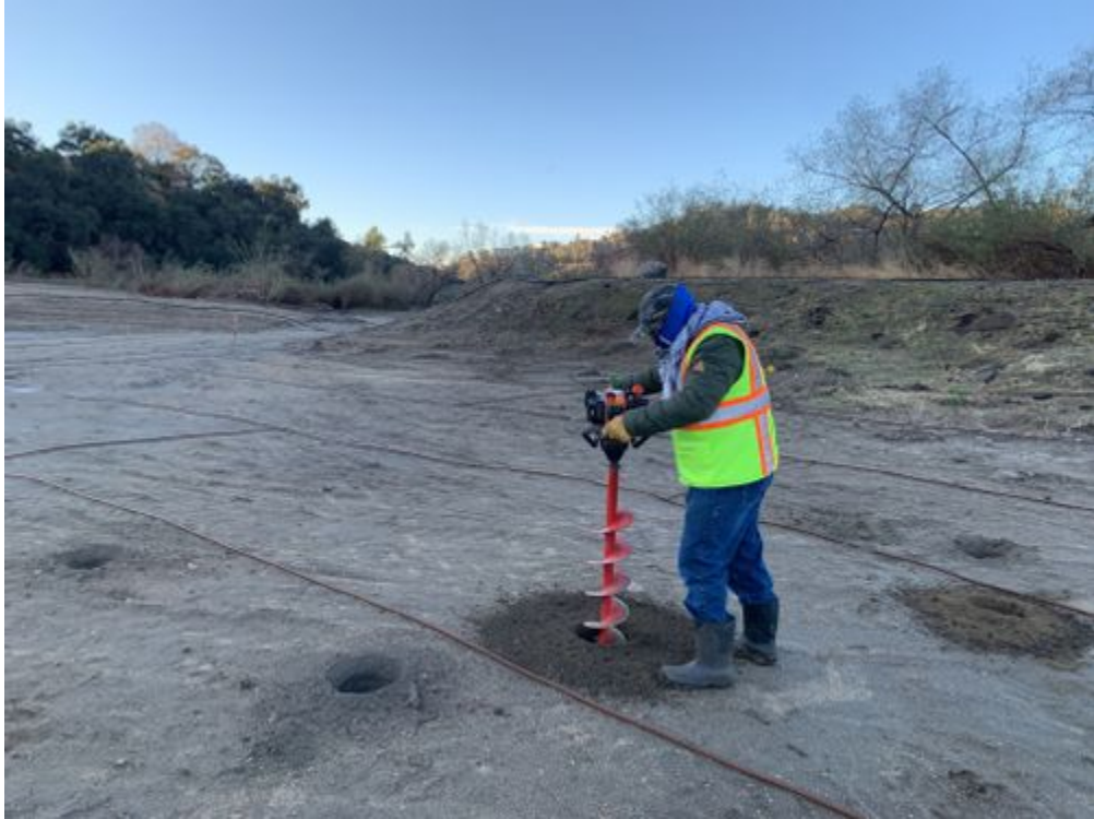
photo_1-digging_with_auger_facingS.jpg -118.1719 34.19143
