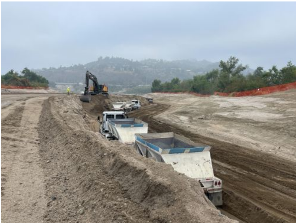
photo_4-sediment hauling activities.jpg -118.17182 34.19283
