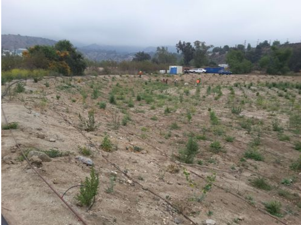
Starting work in DG-W-1.jpg -118.17222 34.19164
