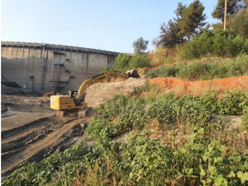
Excavator removing emergent vegetation_facing south.jpg
