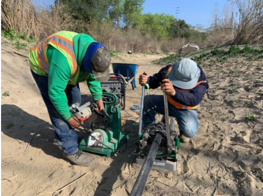
photo_3-crew_fusing_pipe_facingS.jpg -118.17463 34.19244
