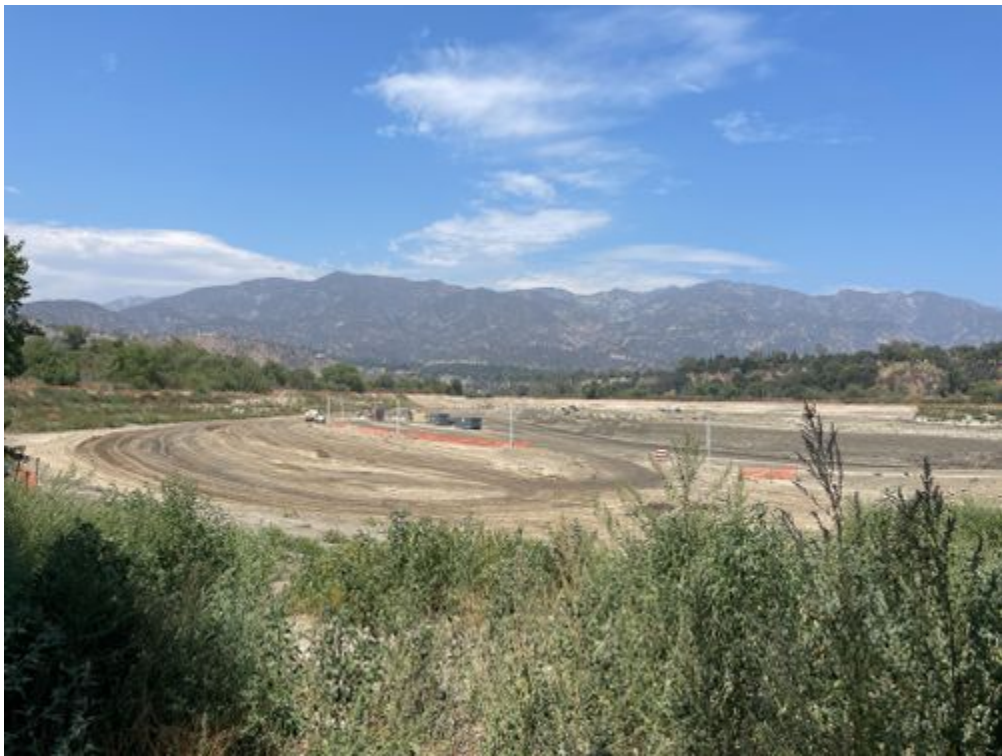
Overview of northeast portion of site_facingSW.jpg -118.17678 34.18724
