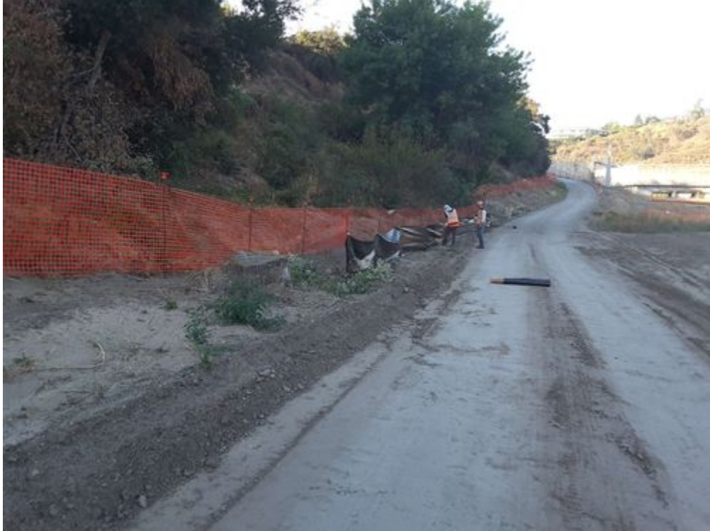
Fence install_east road_facingS.jpg -118.17327 34.18693
