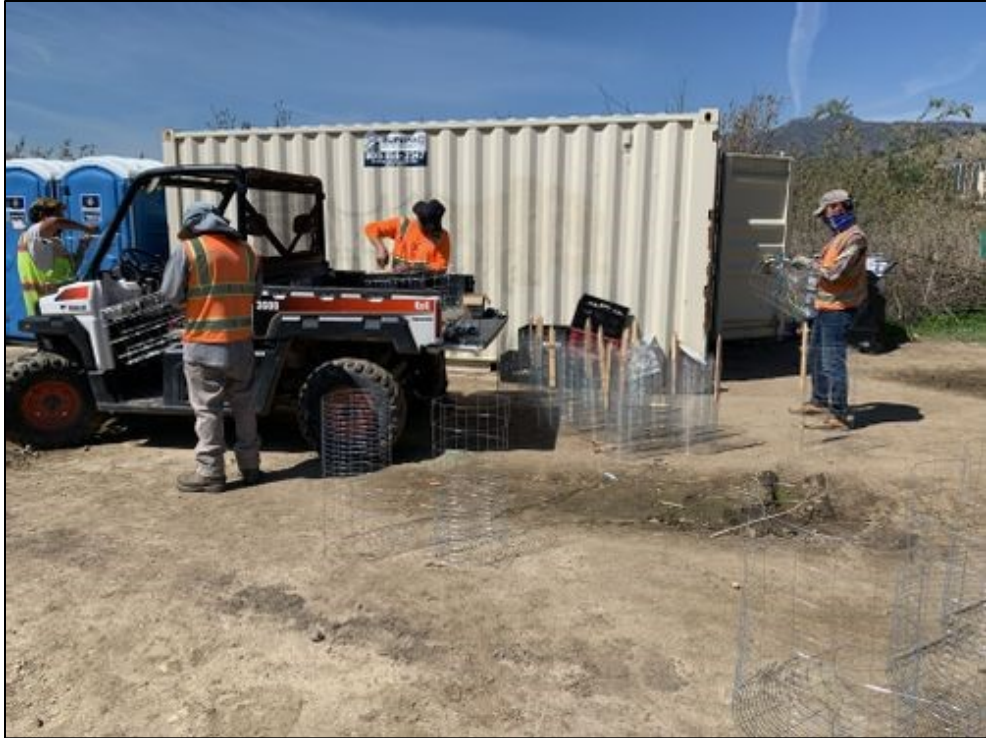
Photo 19. Overview Phase 2 Cage Creation for Container Plants
