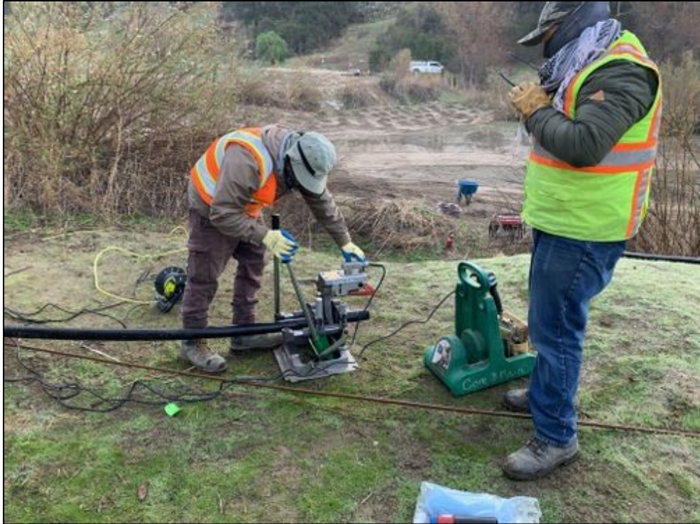
Photo 17. Overview Phase 2 Irrigation Installation
