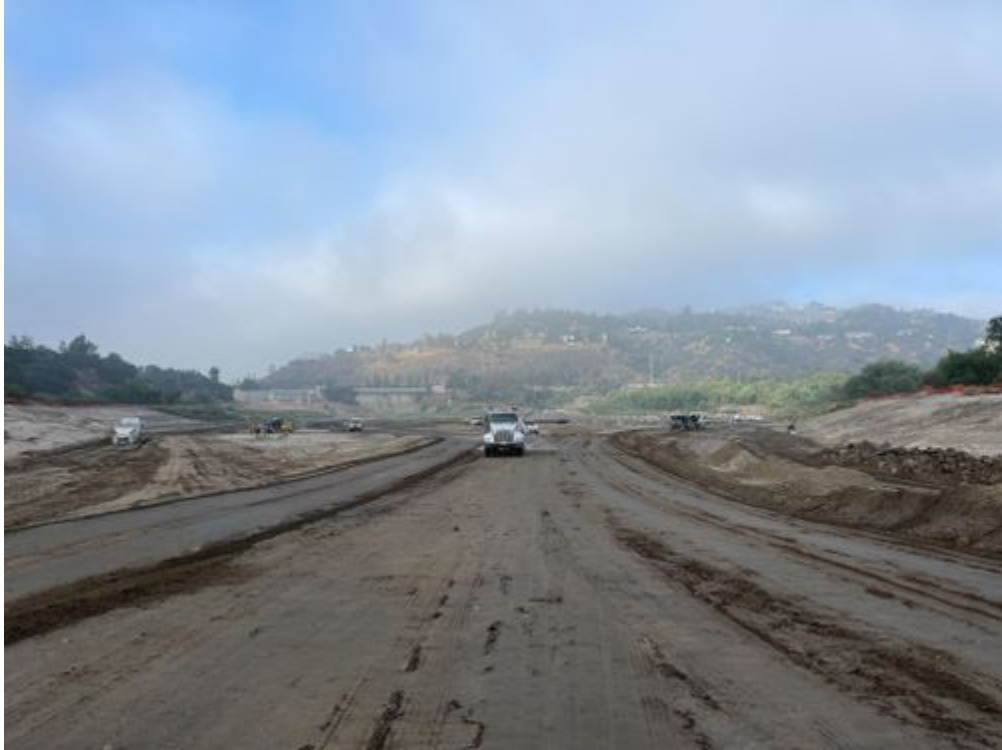
photo_3-sediment hauling activities.jpg -118.17288 34.19157
