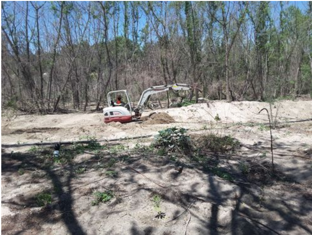
Dirt moving to fix channel_DG-W-2_facing W.jpg -118.17399 34.19296
