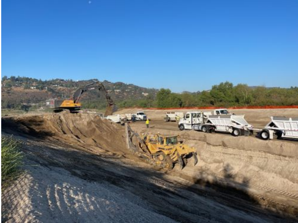
Excavator_1_eastern edge looking SW.jpg -118.1722 34.19189
