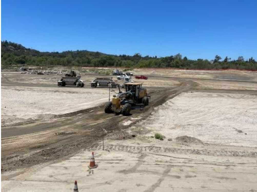
Grader_grading_alongside KILL-3 buffer.jpg -118.17293 34.18998
