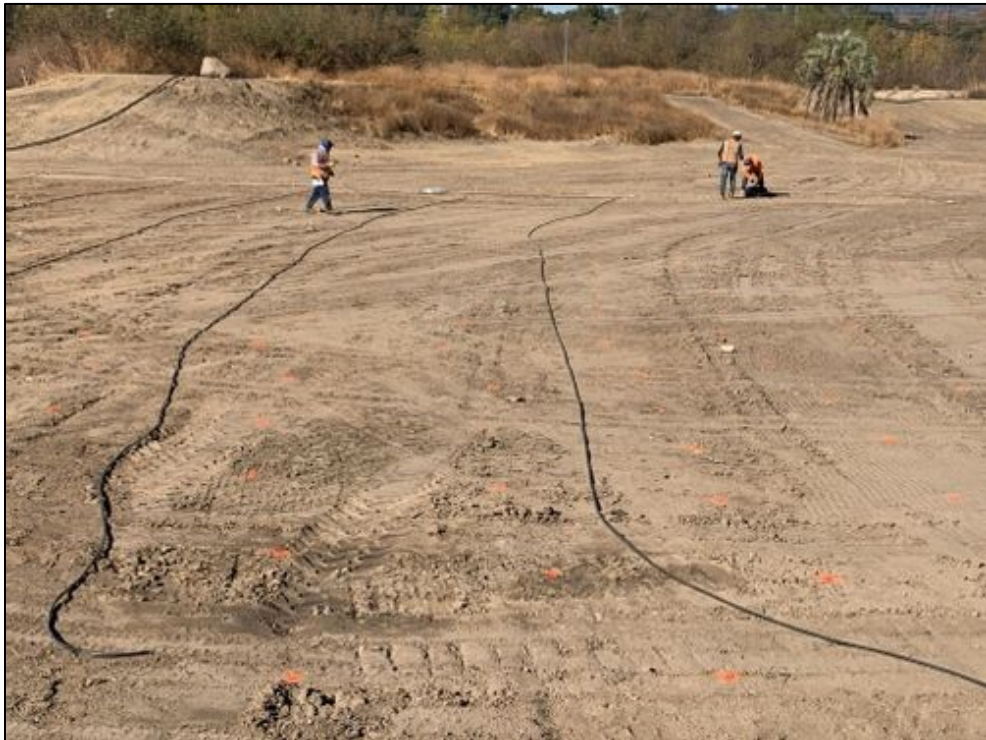
Photo 14. Overview Phase 2 Irrigation Installation
