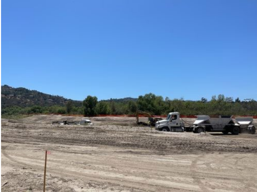
Excavator_II level_with_Johnsons field_061021.jpg -118.17212 34.19188
