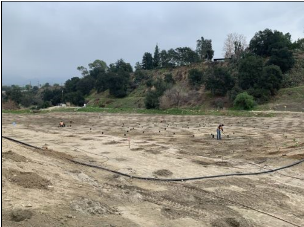
Photo 16. Overview Phase 2 Container Plant Installation
