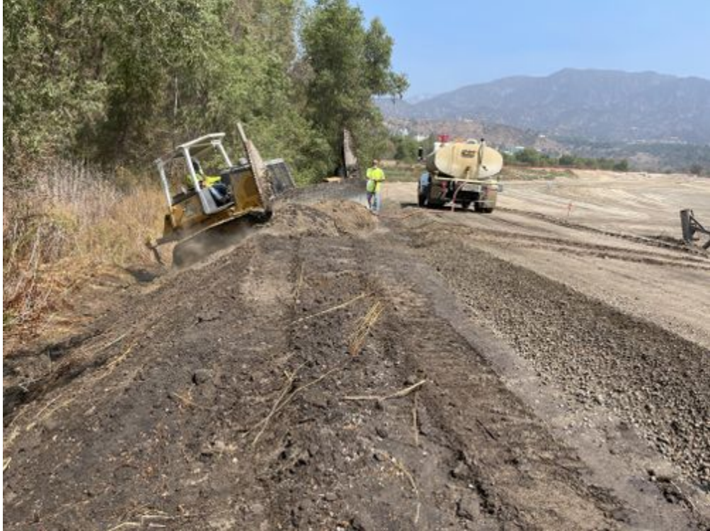
Mini_bulldozer_grading_new_road_edges_082421.jpg -118.17682 34.18668
