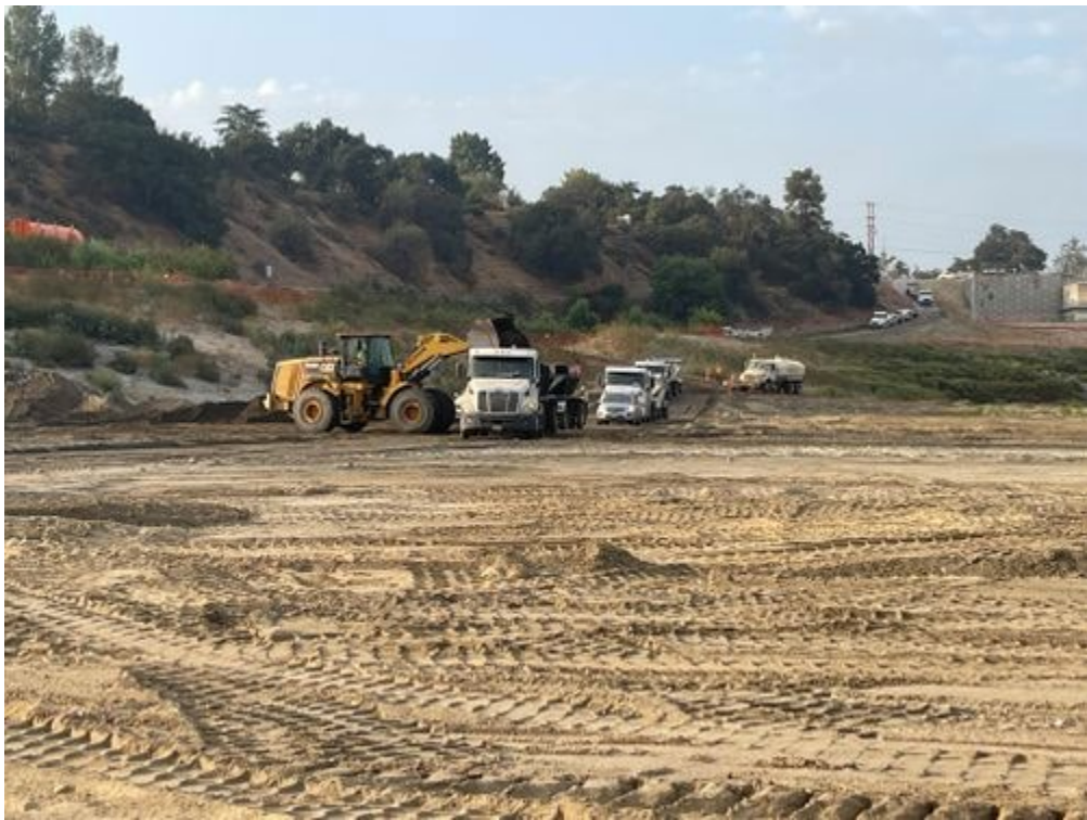
Front loader loading haulage ts_071621.jpg -118.17386 34.18941
