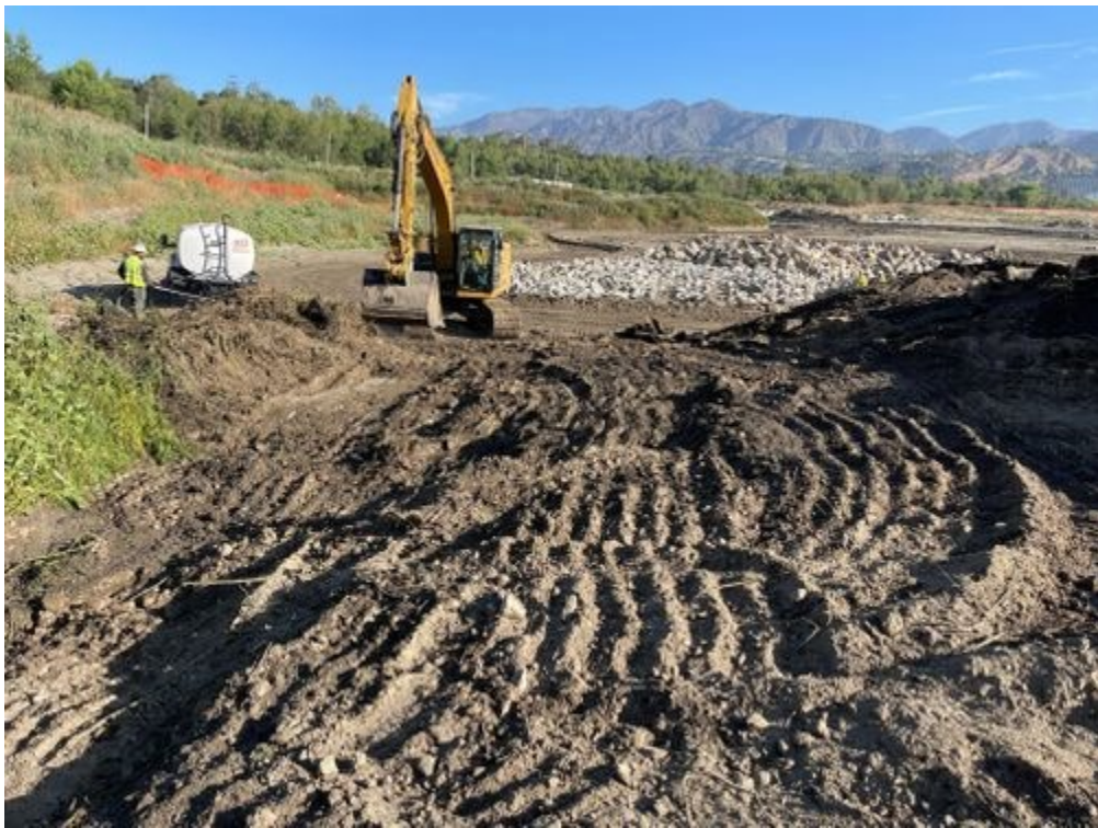
Veg removed_southern section_072221.jpg -118.17518547222222 34.18573830555555
