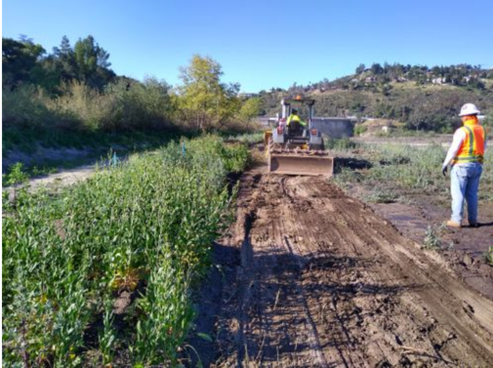
photo_1-skip loader clearing esa fenceline.jpg -118.17276 34.18913
