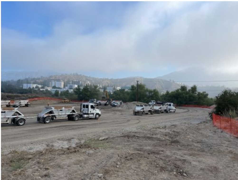
Northern end of the project site_063021.jpg -118.17018 34.19422
