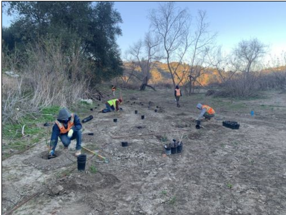
Photo 8. Overview Phase 2 Container Plant Installation
