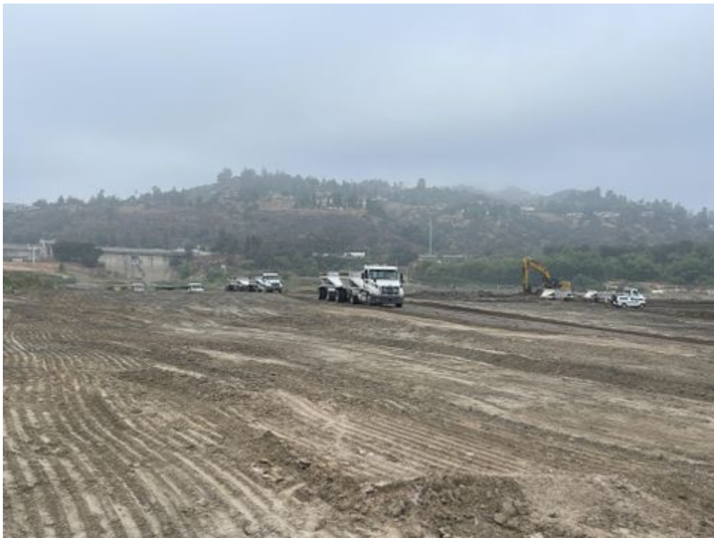
Site overview looking south_070121.jpg -118.17274 34.18975
