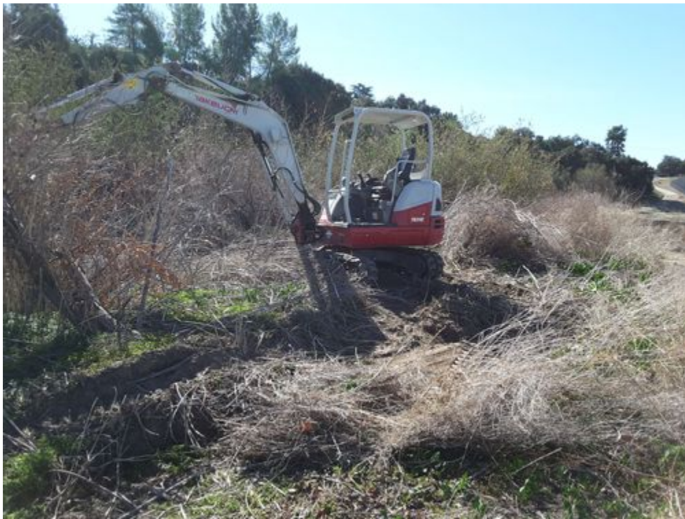
Photo 2-clearing south end of DG-2.jpg -118.17317 34.18817
