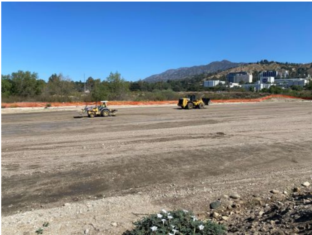
06-24-2021_compacting_soil_facingW.jpg
