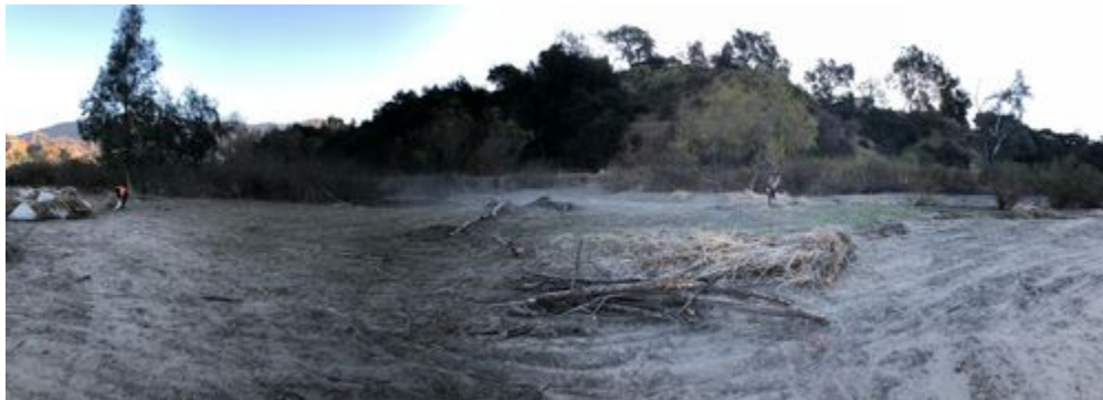
Vegetation clearing_before_facingE _1.jpg
