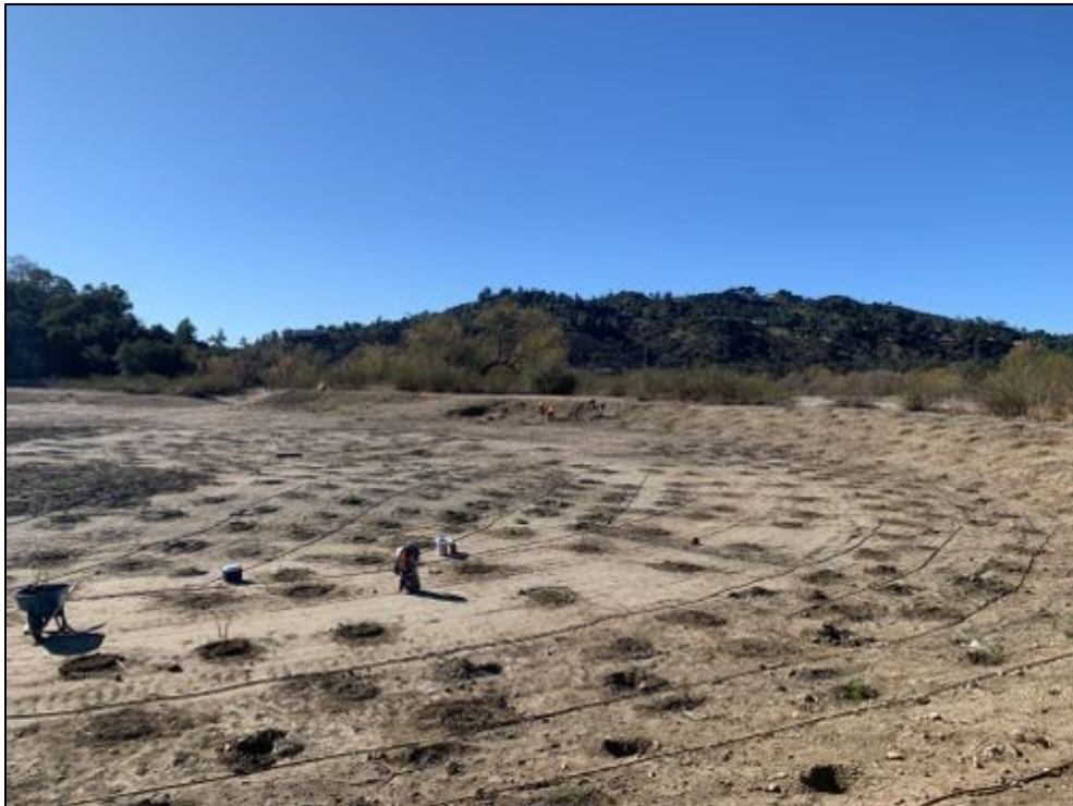
Photo 2. Overview Phase 2 Container Plant Installation
