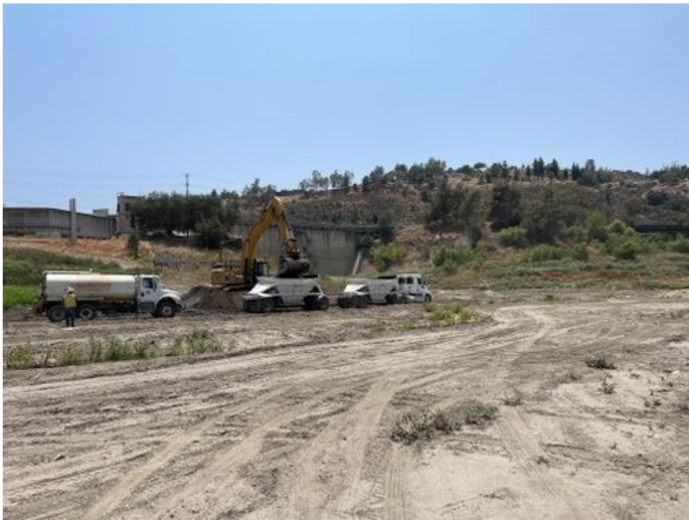
Excavator in southern section_071521.jpg -118.17382 34.18766
