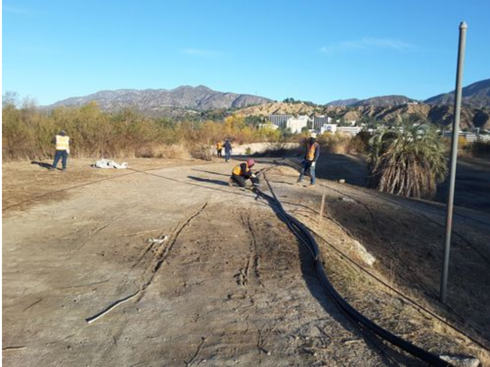
Laying irrigation_DG-W-1_facing W.jpg -118.17211 34.19127
