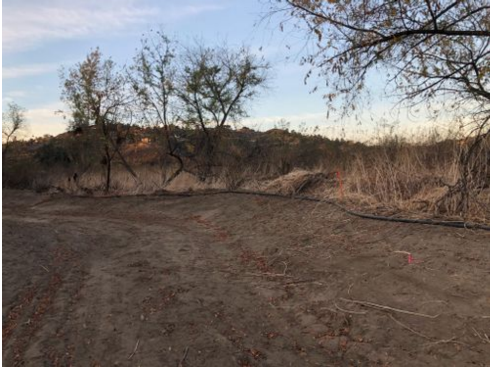
vegetation clearing_before_facing W.jpg
