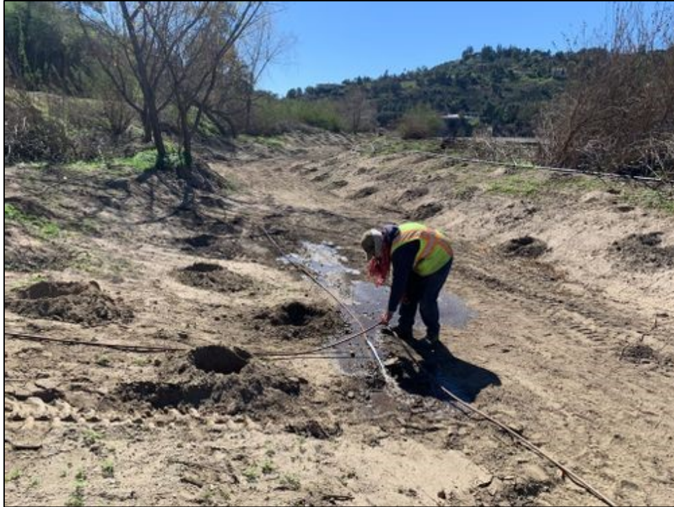
Photo 7. Overview Phase 2 Irrigation Installation
