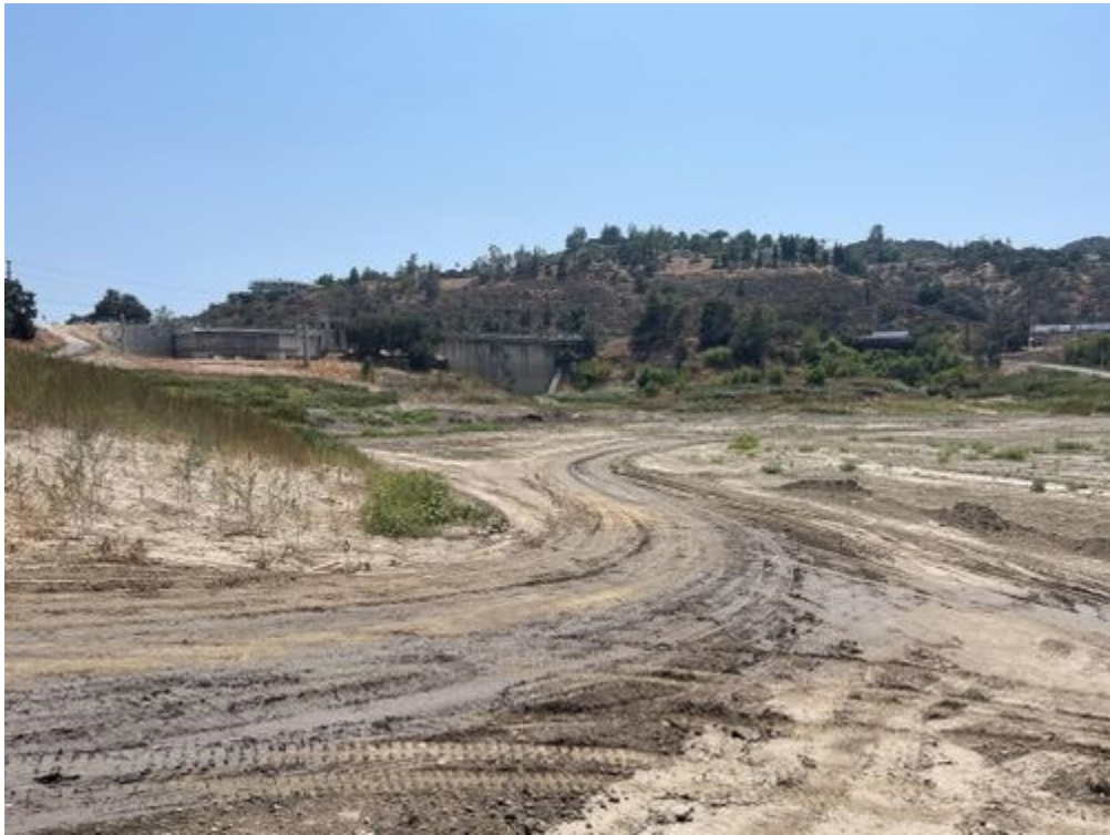
Southern end of site_071621.jpg -118.17361 34.18784
