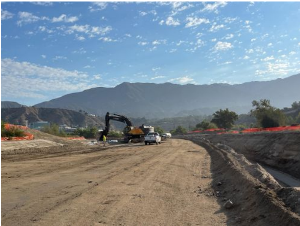
Excavator 2_taken facing N_070821.jpg -118.1718 34.19158
