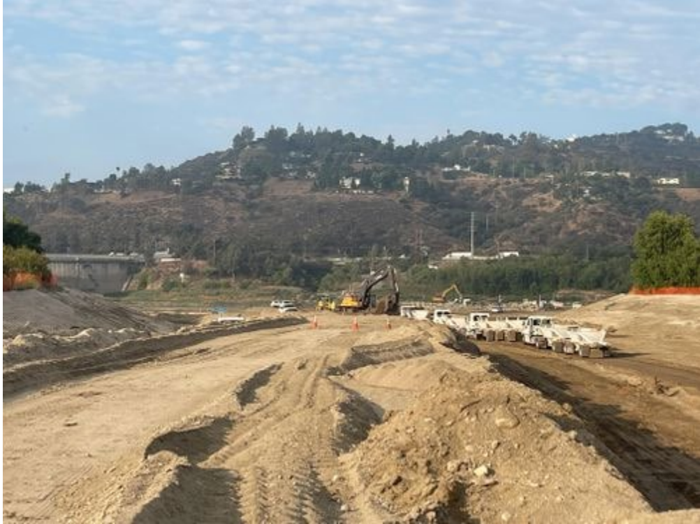
Excavator 2_looking S from marker 29_071621.jpg -118.17194 34.19278
