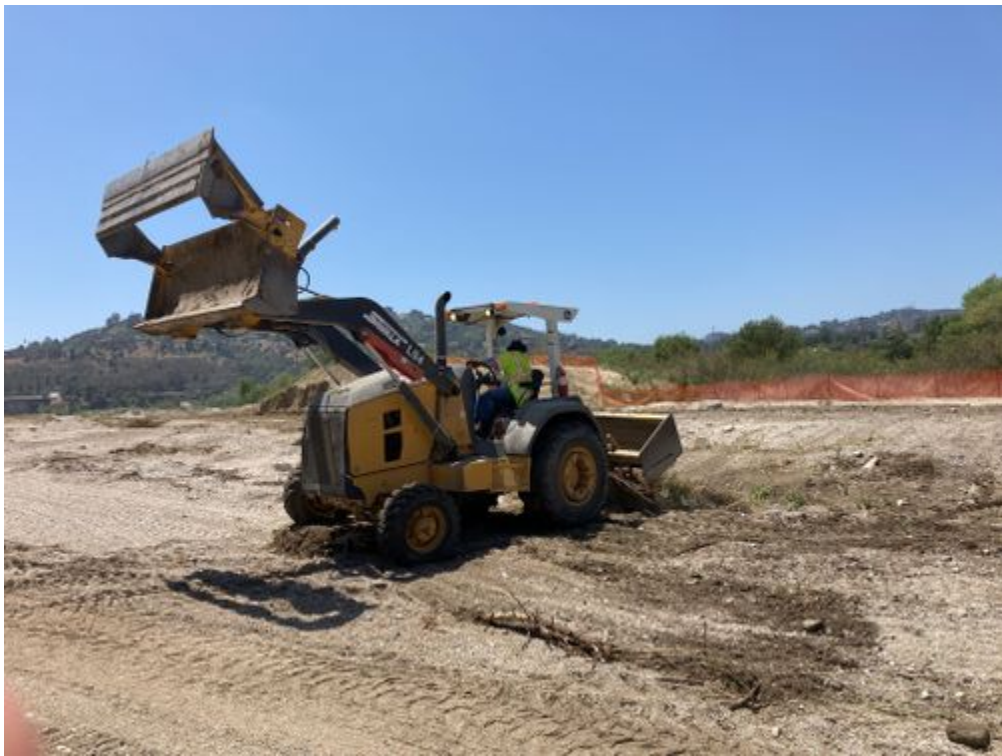
Consolidate vegetation piles_facingSW.jpg -118.17137 34.19405
