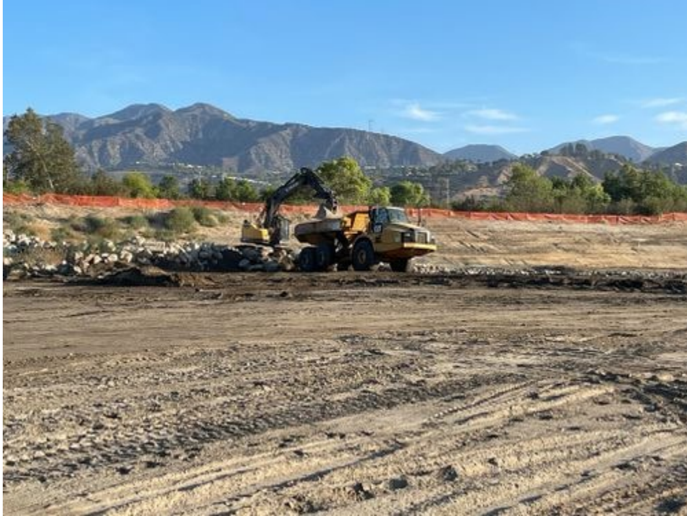
Loading rockpile to haul to the Southern section_072221.jpg -118.17424419444446 34.1891780277777
