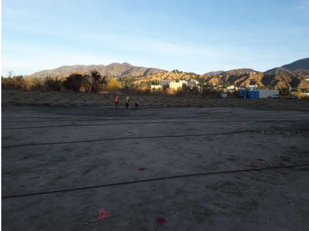
Digging holes_DG-W-1_facing NW.jpg -118.17169 34.19154
