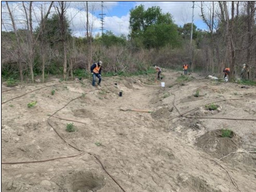
Photo 22. Overview Phase 2 Container Plant Installation
