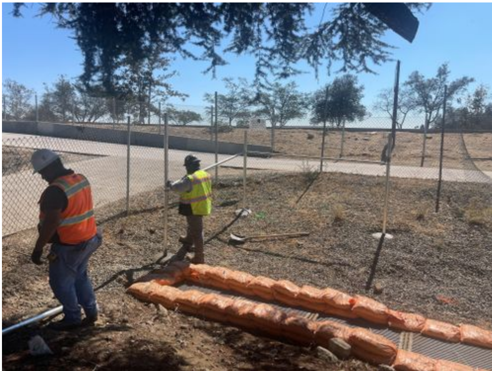
Ace_fencing_attaching_cross_bars_between_fence_posts_093021.jpg -118.17344237222223 34.18524683333333
