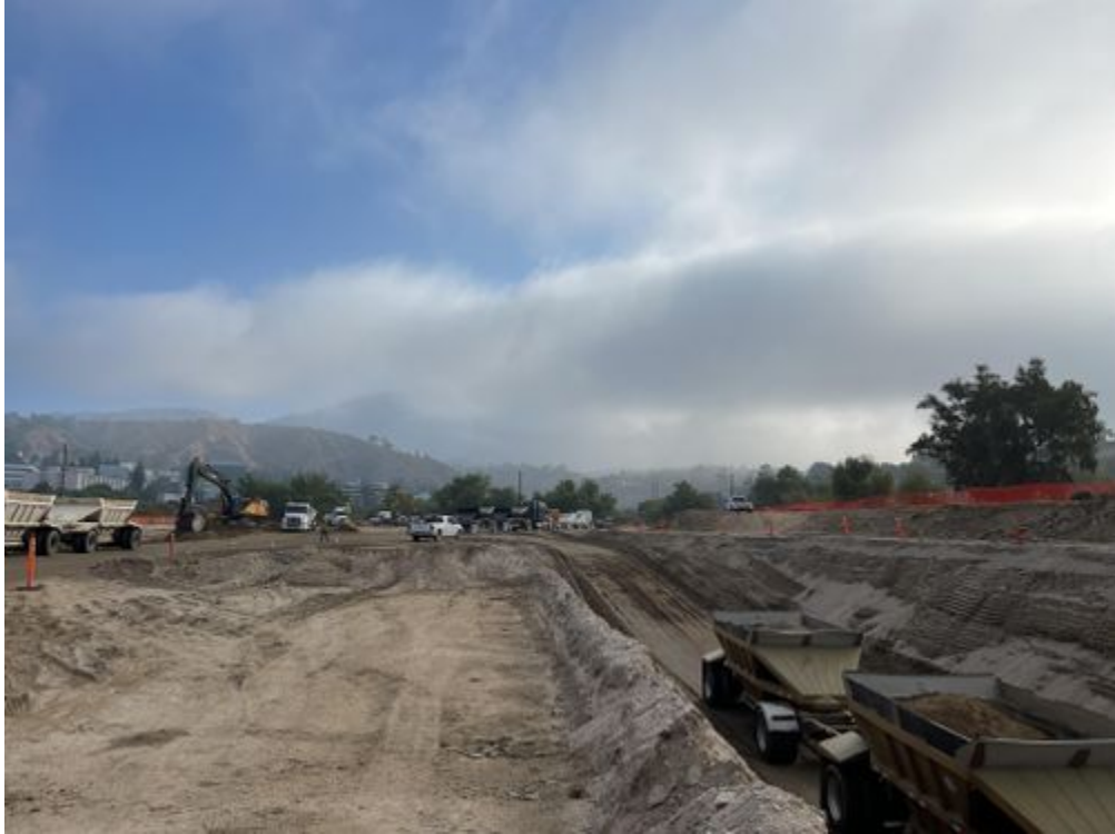
Overview of northern section of site_063021.jpg -118.17162 34.19312
