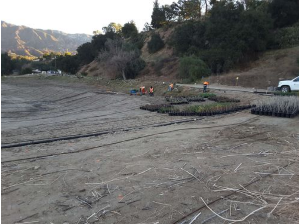
Digging holes and planting_DG-W-1_facing NE.jpg -118.17166 34.19082
