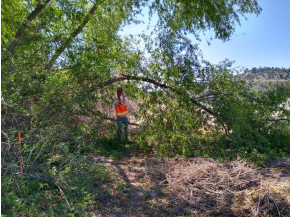
photo_3-branch of willow hanging into work area removed with chainsaw.jpg -118.17242 34.1912
