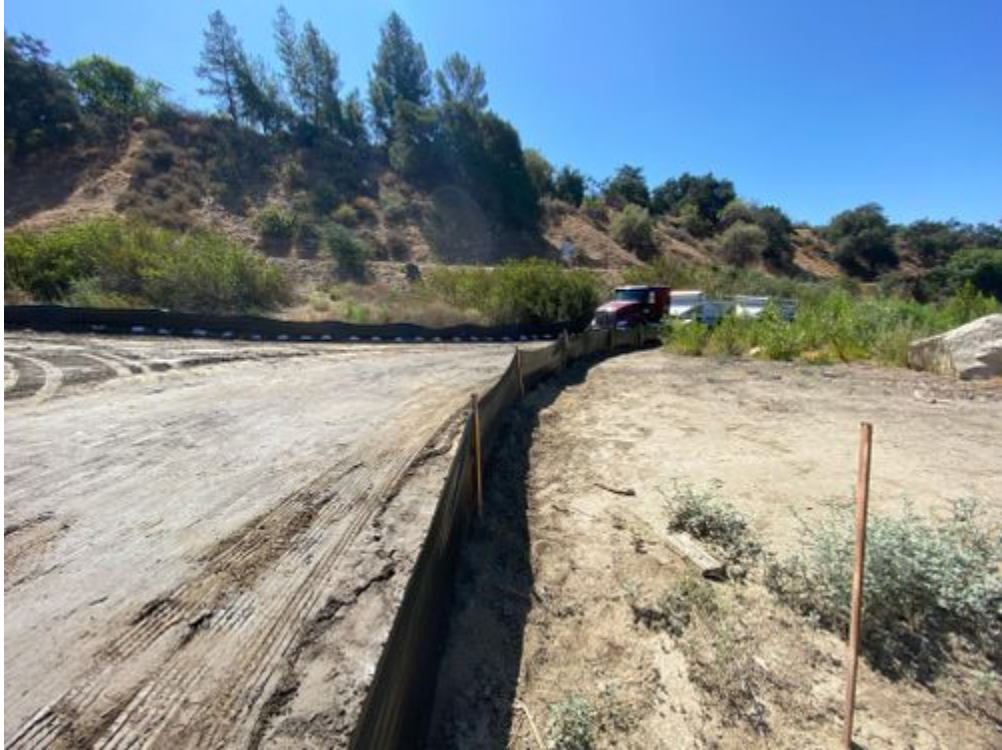
07-06-2021_silt_fence_installation_complete_facingSE.jpg
