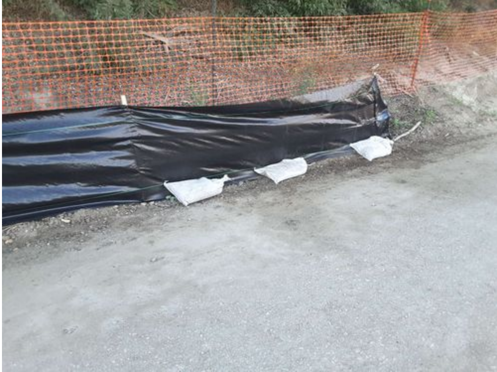
Securing fence with sandbags.jpg -118.17338 34.18655
