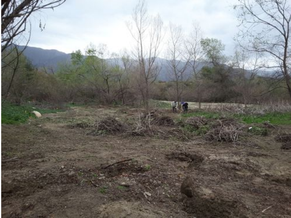
After clearing DG-W-2.jpg -118.17428 34.19342
