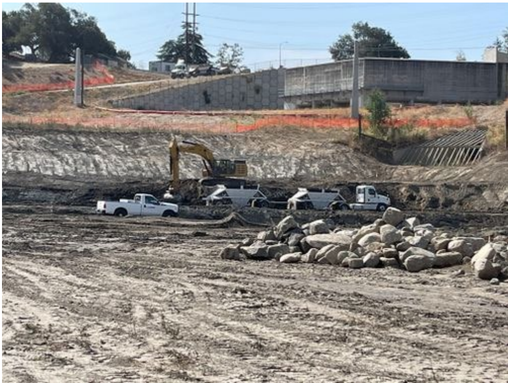
Excavator loading haulage truck_072321.jpg -118.17535026111112 34.18700996666665
