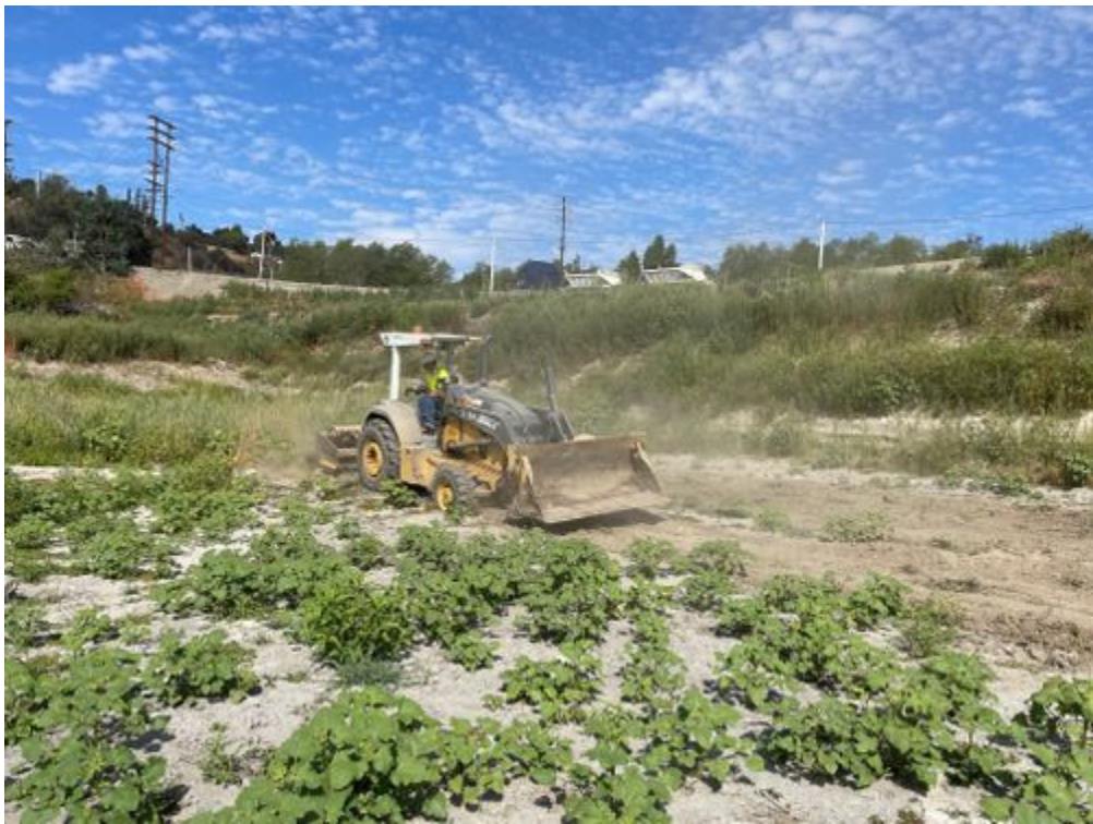
Box scraper removing vegetation _southern section_070821.jpg -118.17581 34.1867
