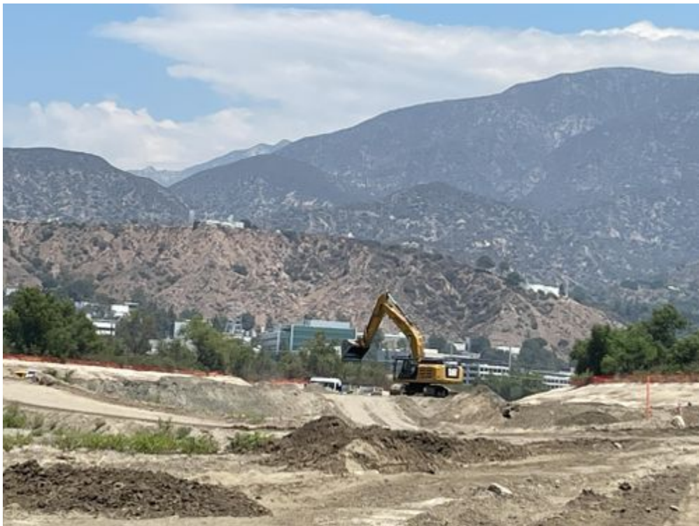
Excavator 1 loading haulage trucks_070921.jpg -118.17392 34.18737
