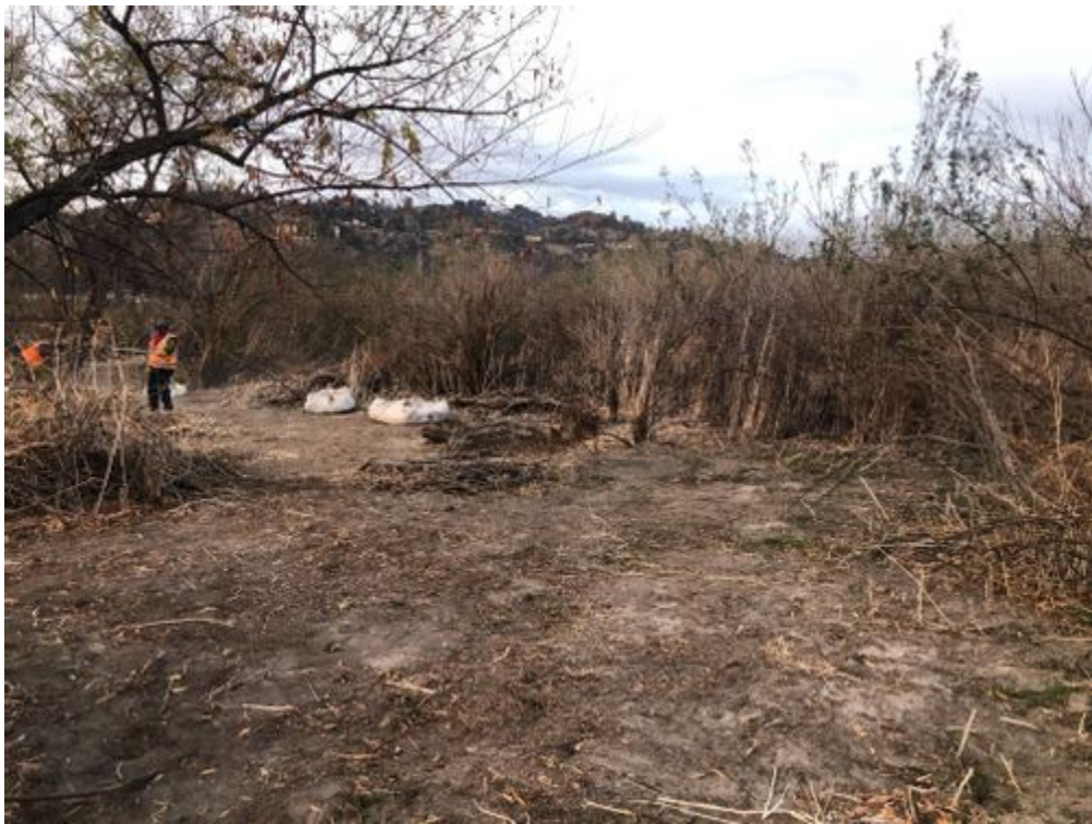
Vegetation clearing before facing S.jpg
