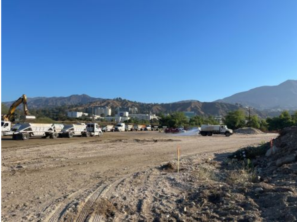
Overview of site looking NW.jpg -118.1714 34.1932
