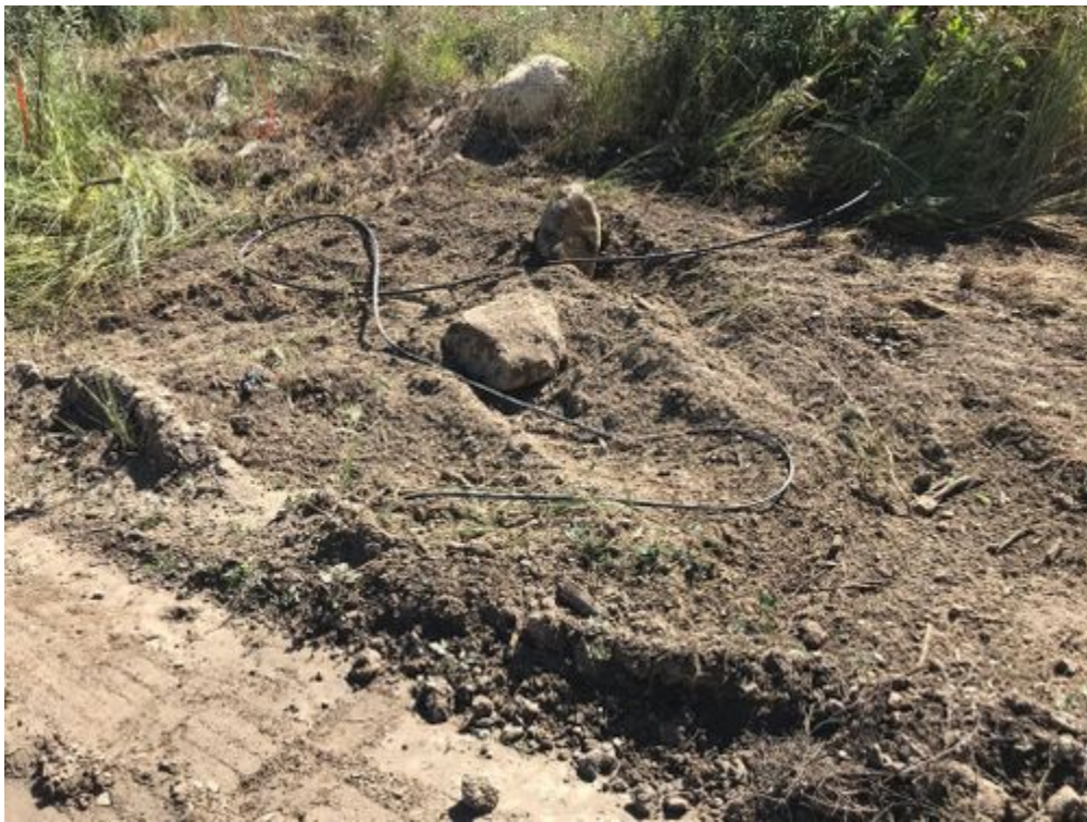
04-29-21_broken_irrigation_line.jpg
