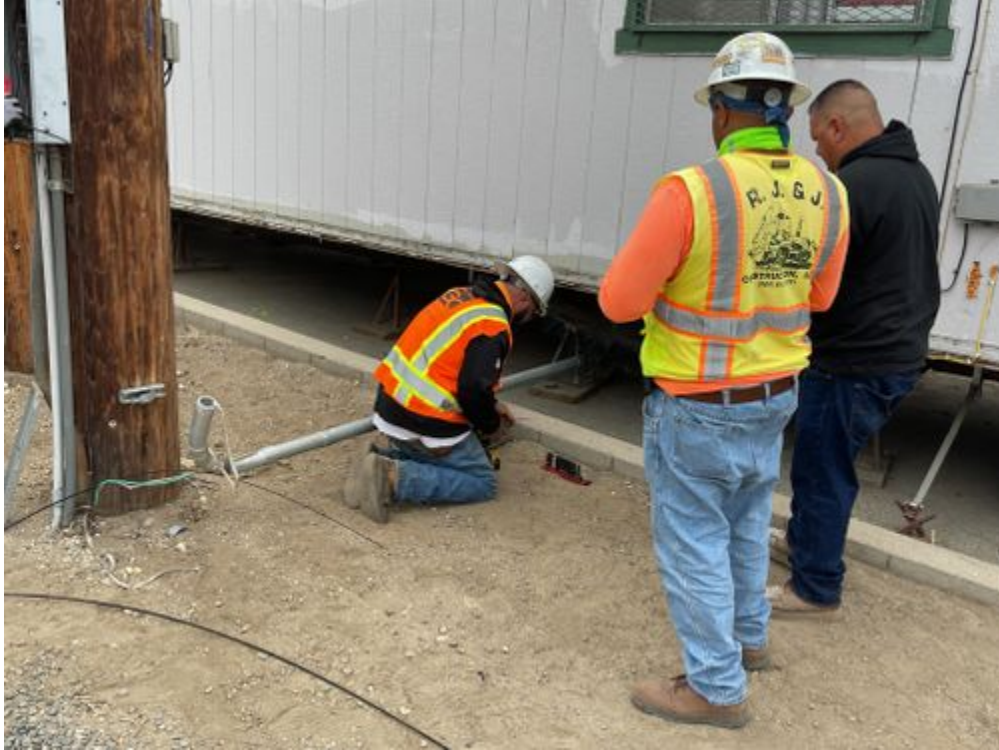
Griffiths_crew_removing_pipes_housing_wiring_092821.jpg -118.17354630555556 34.185330025
