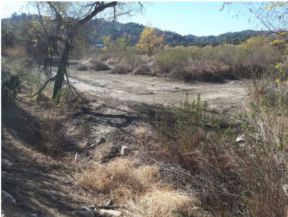
Irrigation install in progress_DG-2_facing SW.jpg -118.17141 34.19075
