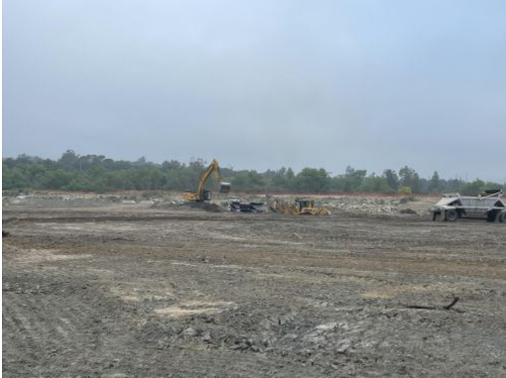
Excavator_near weigh station_070121.jpg -118.17317 34.18871
