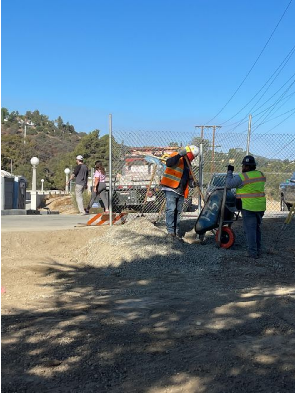
Pouring_concrete_into_fence_post_holes_093021.jpg -118.17342625 34.18525433888889
