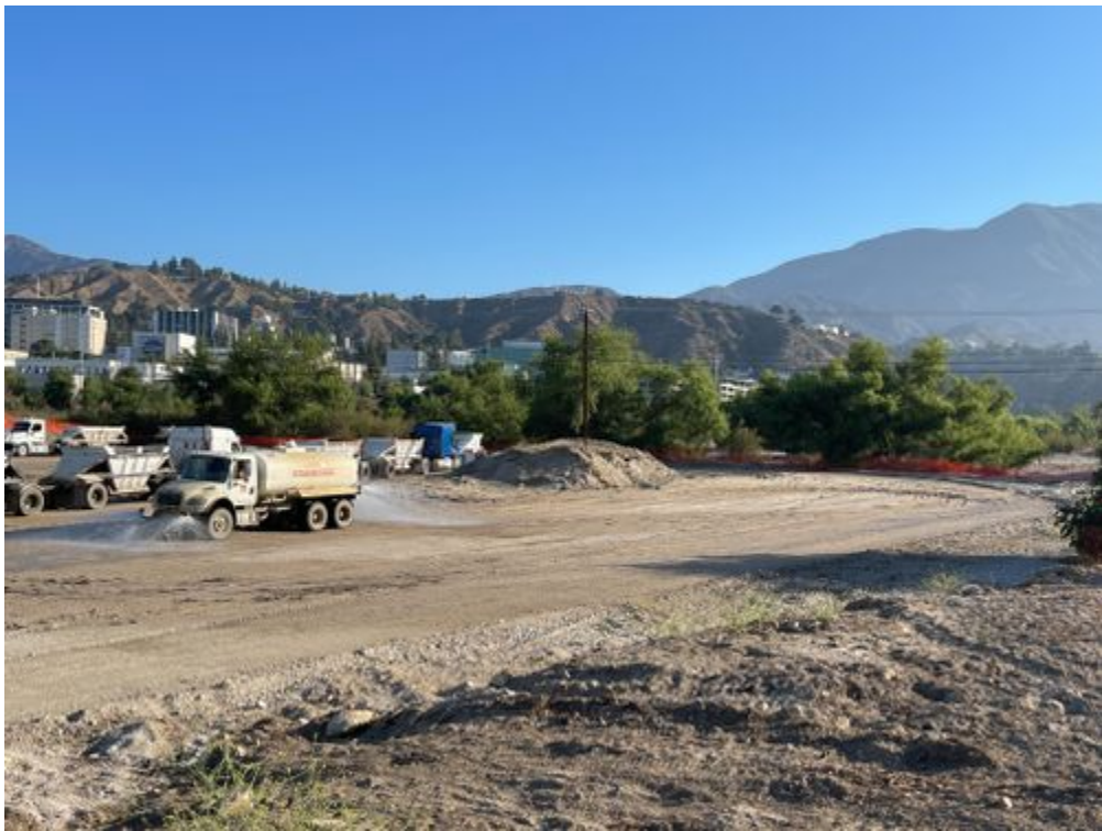
photo_4-sediment hauling activities.jpg -118.17088 34.19393
