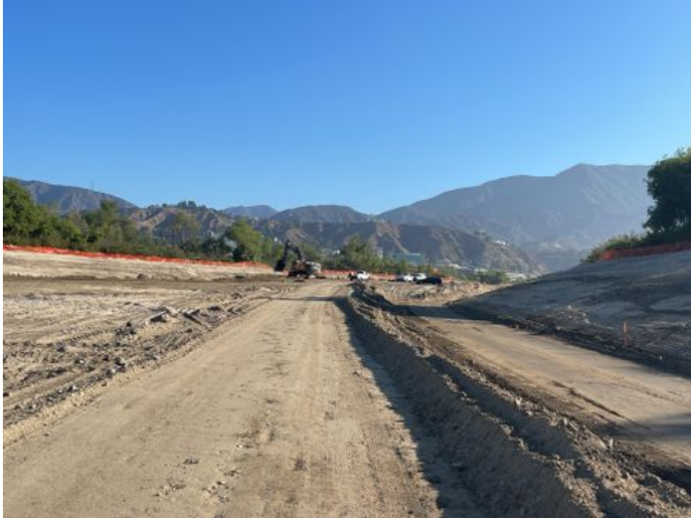
Excavator 2 towards the north end with hauler routes_070721.jpg -118.17289 34.19046
