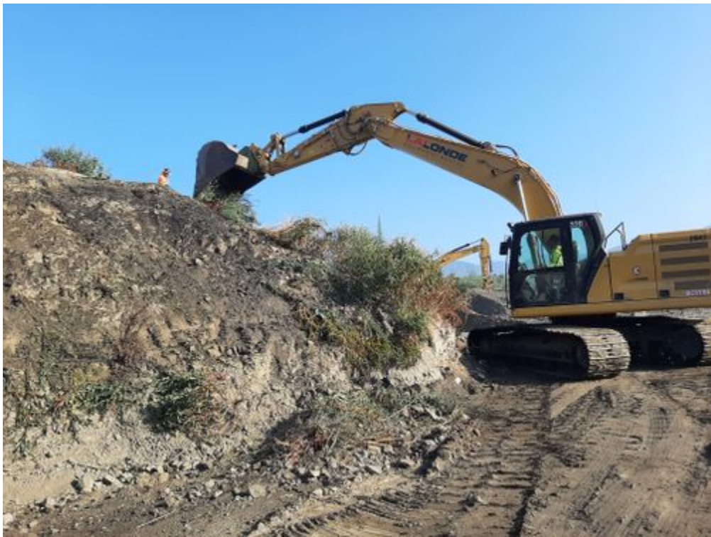
Excavator removing emergent vegetation_facing north.jpg
