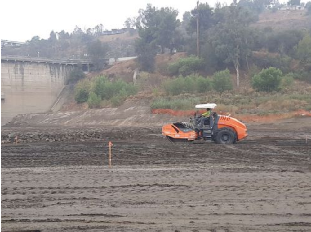
photo_4_foot/toe_roller_compacting_fill_noth_of_dam.jpg -118.1753 34.18709
