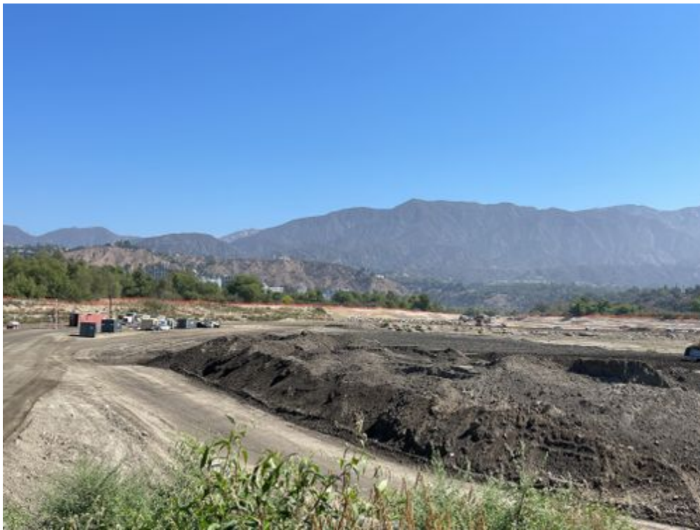
photo_4-sediment hauling activities.jpg -118.17584 34.1872
