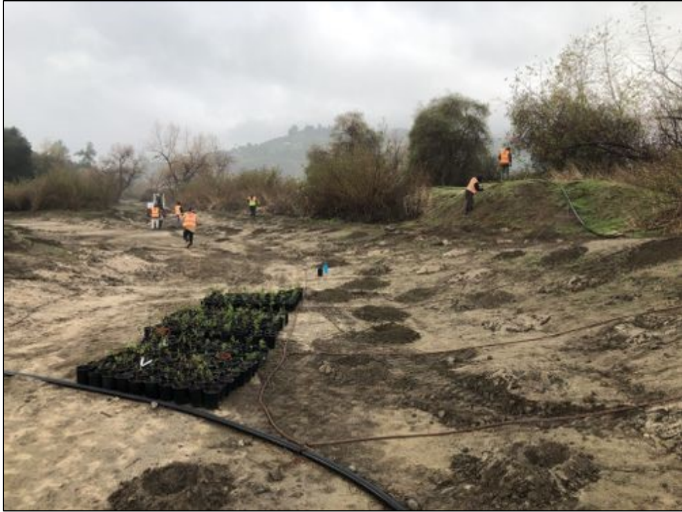
Photo 5. Overview Phase 2 Container Plant Installation
