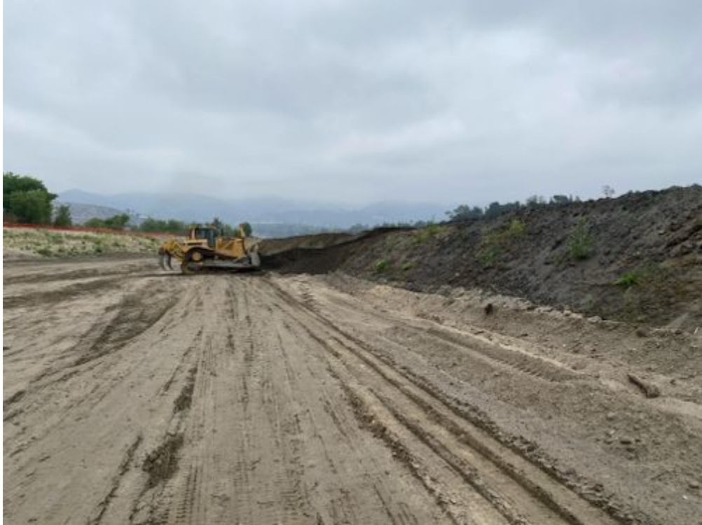
Bulldozer_removing_vegetation_facingN.jpg
