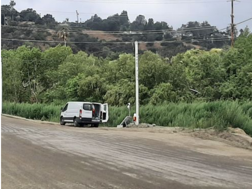
Camera and solar installation along western haul road and powerline.jpg
