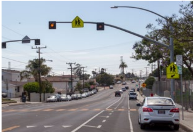
Pedestrian Activated Warning Beacons are flashing yellow lights that provide additional warning to drivers that a pedestrian is crossing the street.
