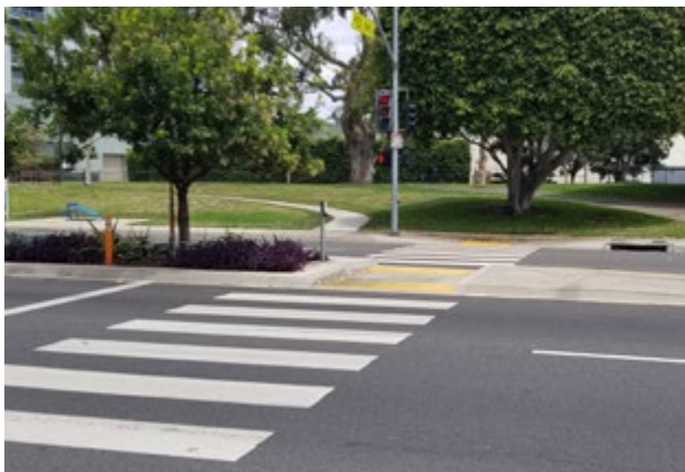
Refuge Islands provide a space within a median, mid-way through a crosswalk for people to wait for a gap in traffic before continuing to cross a wide street.
