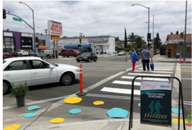
Temporary Street Enhancements include paint and flexible posts/bollards and are typically installed to determine a proposed project's impact and obtain community feedback before permanent enhancements are implemented.
