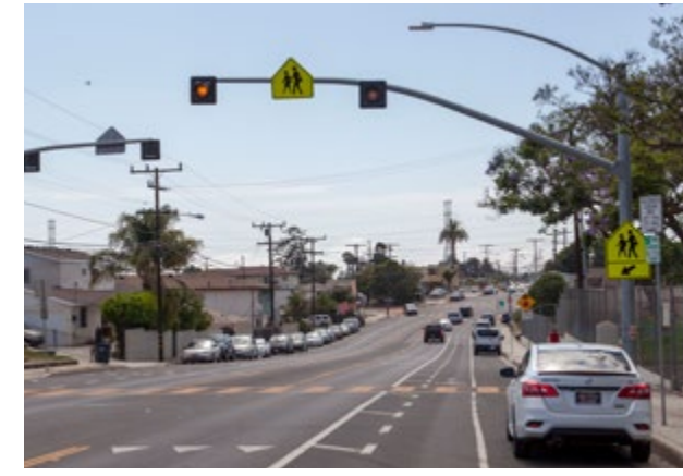
Pedestrian Activated Warning Beacons are flashing yellow lights that provide additional warning to drivers that a pedestrian is crossing the street.
