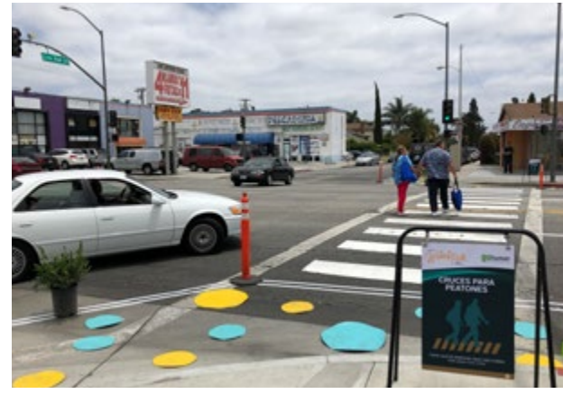
Temporary Street Enhancements include paint and flexible posts/bollards and are typically installed to determine a proposed project's impact and obtain community feedback before permanent enhancements are implemented.
