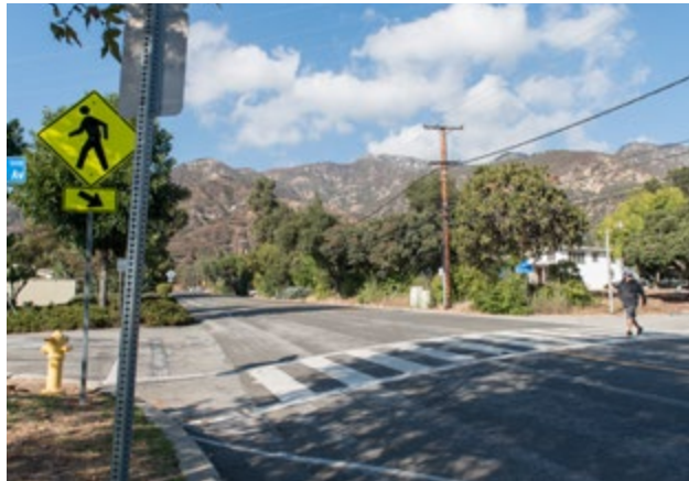
High visibility crosswalks make pedestrian crossings easier to see and alert drivers that they are approaching a pedestrian crossing.
