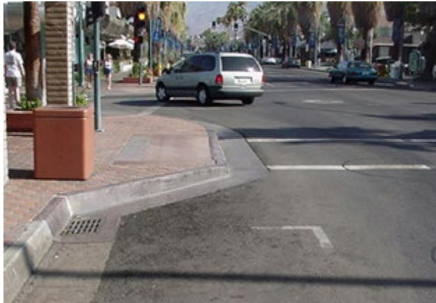
Curb extensions (also known as bulb-outs) shorten the crossing distance for pedestrians, slow down turning vehicles, and enhance the ability for pedestrians and motorists to see each other.
