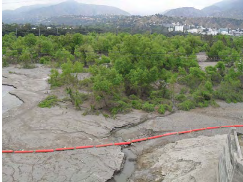
Photo 1: Photo taken looking northwest depicting the Arroyo Seco stream in the Devil's Gate Reservoir directly behind the dam wall. Scoured and Black Willow Series vegetation communities are within the reservoir along the ephemeral stream.
