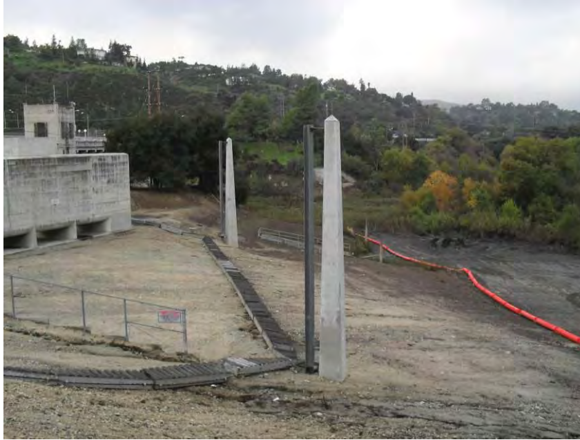
Photo 1: Photo taken from Photo Point 1 looking west depicting the spillway of the reservoir with Black Willow Series on the right and Sage Scrub and Oak Woodland at the back. The orange blockage devices are used to prevent debris from building up behind the dam.
