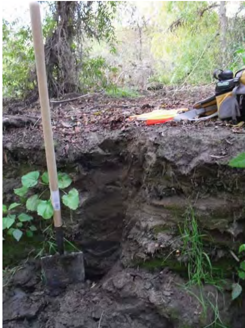
Photo 6: Photo from Photo Point 5 depicting Soil Pit #3. This eroded bank gave a soil profile of 3 feet. Sediment build up was very high at this location as well as with most other soil pit locations. Due to sediment build up following rain events, top soil does not have time to mature in a reservoir like it would under natural conditions (problematic soils).
