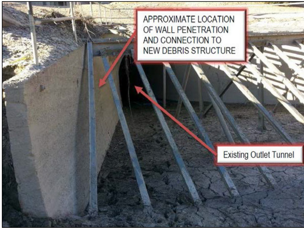
Pump Station Alternative 2 Pipe Inlet Location
