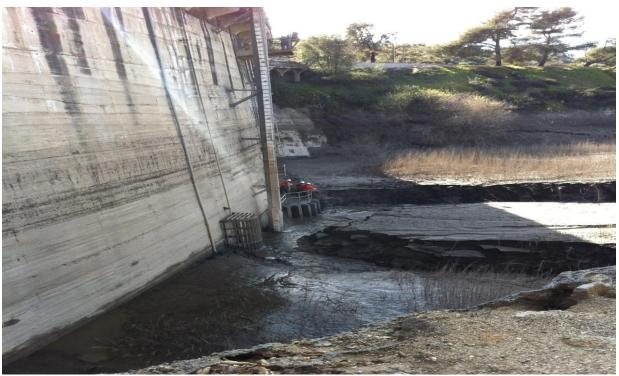
A-4 Sediment Threatening Sluice Gate Post-Station Fire
