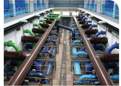
The water from WBMWD is treated at the MWD Weymouth Treatment Plant using conventional treatment methods, which include coagulation, flocculation, sedimentation and filtration. The water is then disinfected to kill any microorganisms, such as bacteria, and reduce the potential for their regrowth in the distribution pipes.
